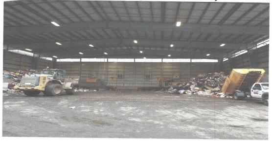
The City's existing transfer station was designed and built 40 years ago using compaction technology. With this type of facility, all waste is deposited on the transfer floor and pushed into a pit where a ram compacts the materials into a trailer. These trailers are transported to the SWA processing or disposal facility where materials are then pushed off the trailer. The existing transfer station represents the following challenges:
