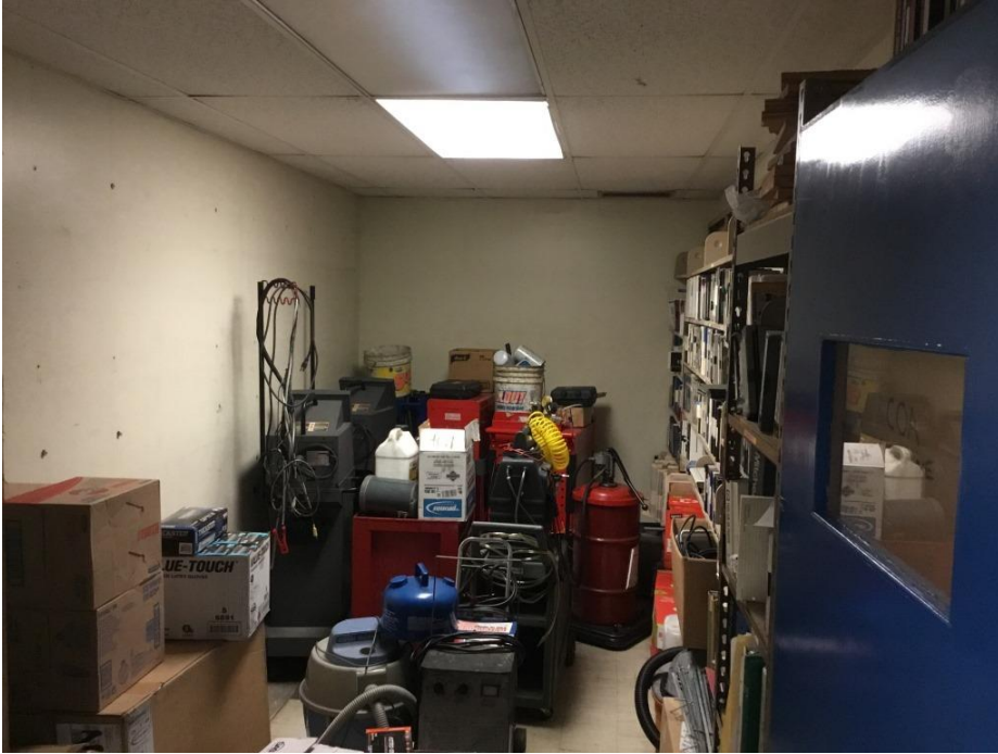
Photograph 5: View depicting the storage room on the second floor and show the asbestos-containing white 9-inch vinyl floor tiles and associated mastic.
