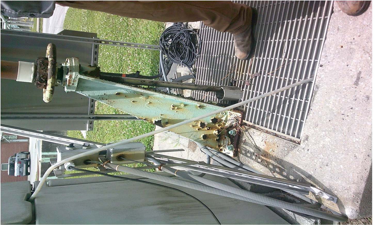
Figure 3: Stem Guide Bearings,
