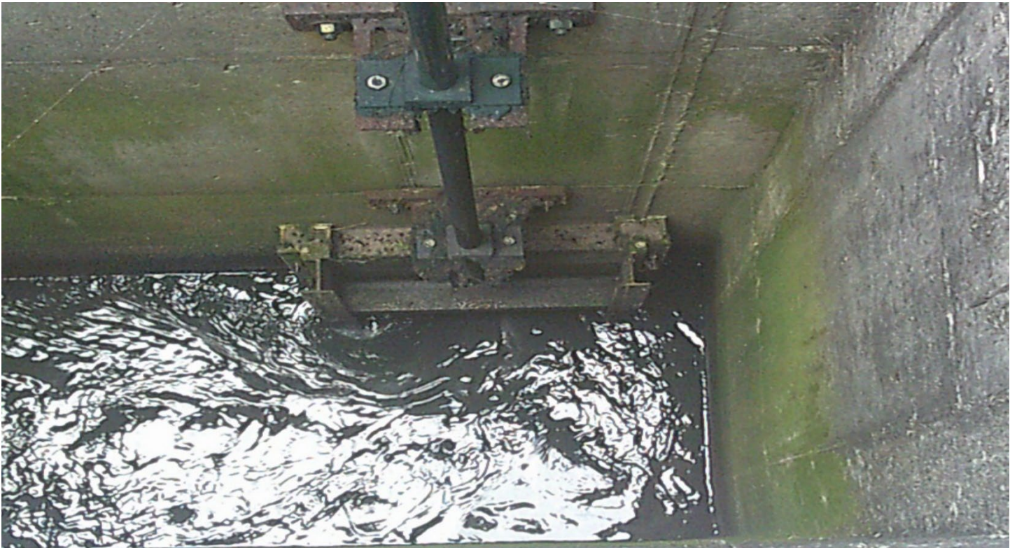
Figure 3: Stem Guide Bearings,
