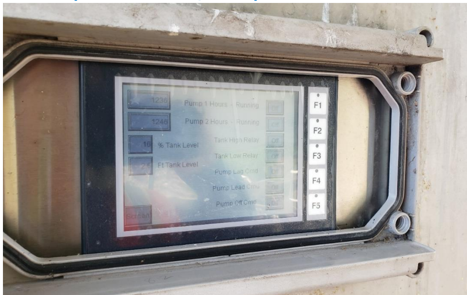
Figure 1-36 Closeup View of Cell 1B/3 Pump Station Controls
