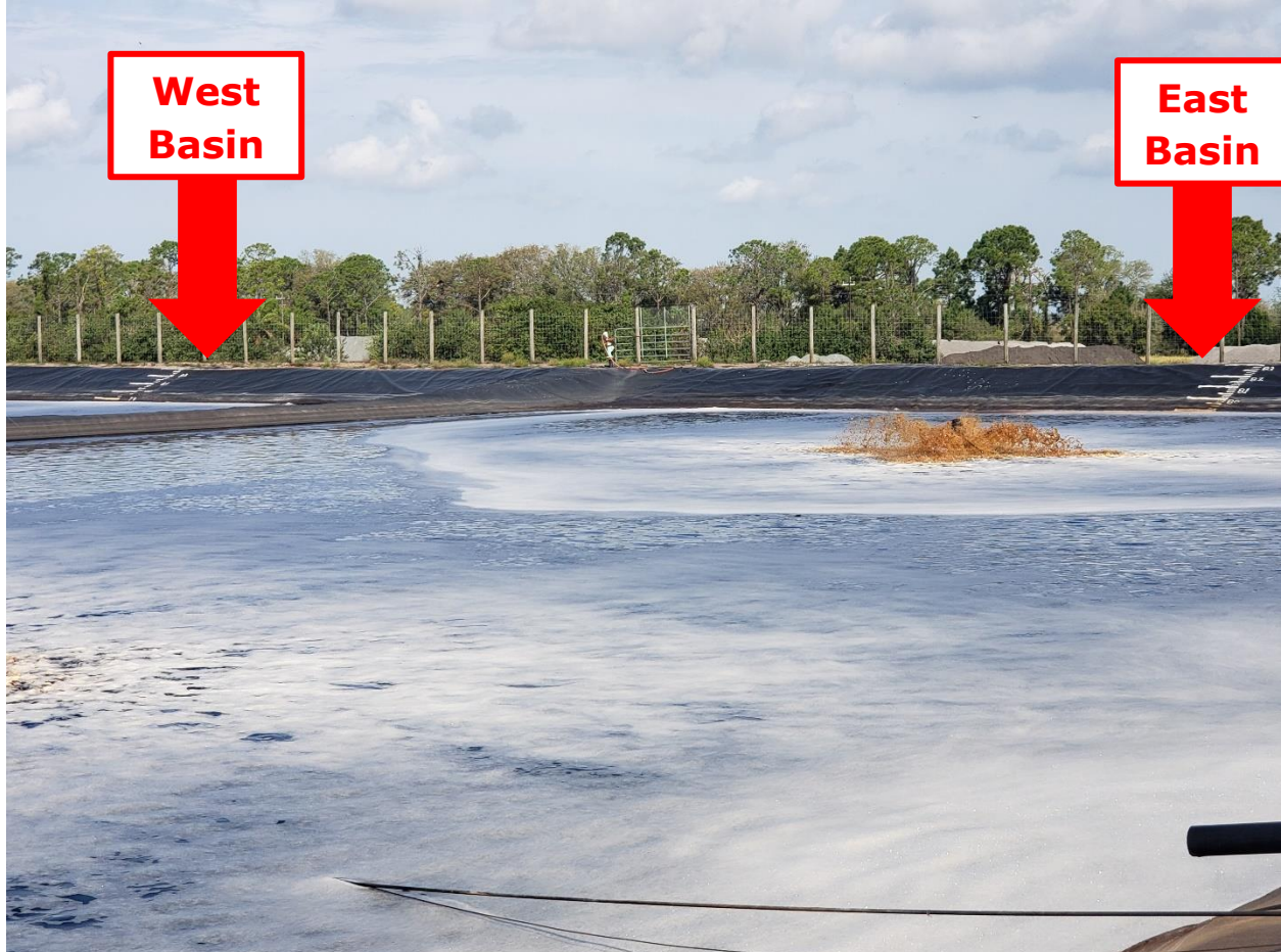
Figure 1-40 Leachate Impoundment Basins with Rain Gauge Indicators Identified
