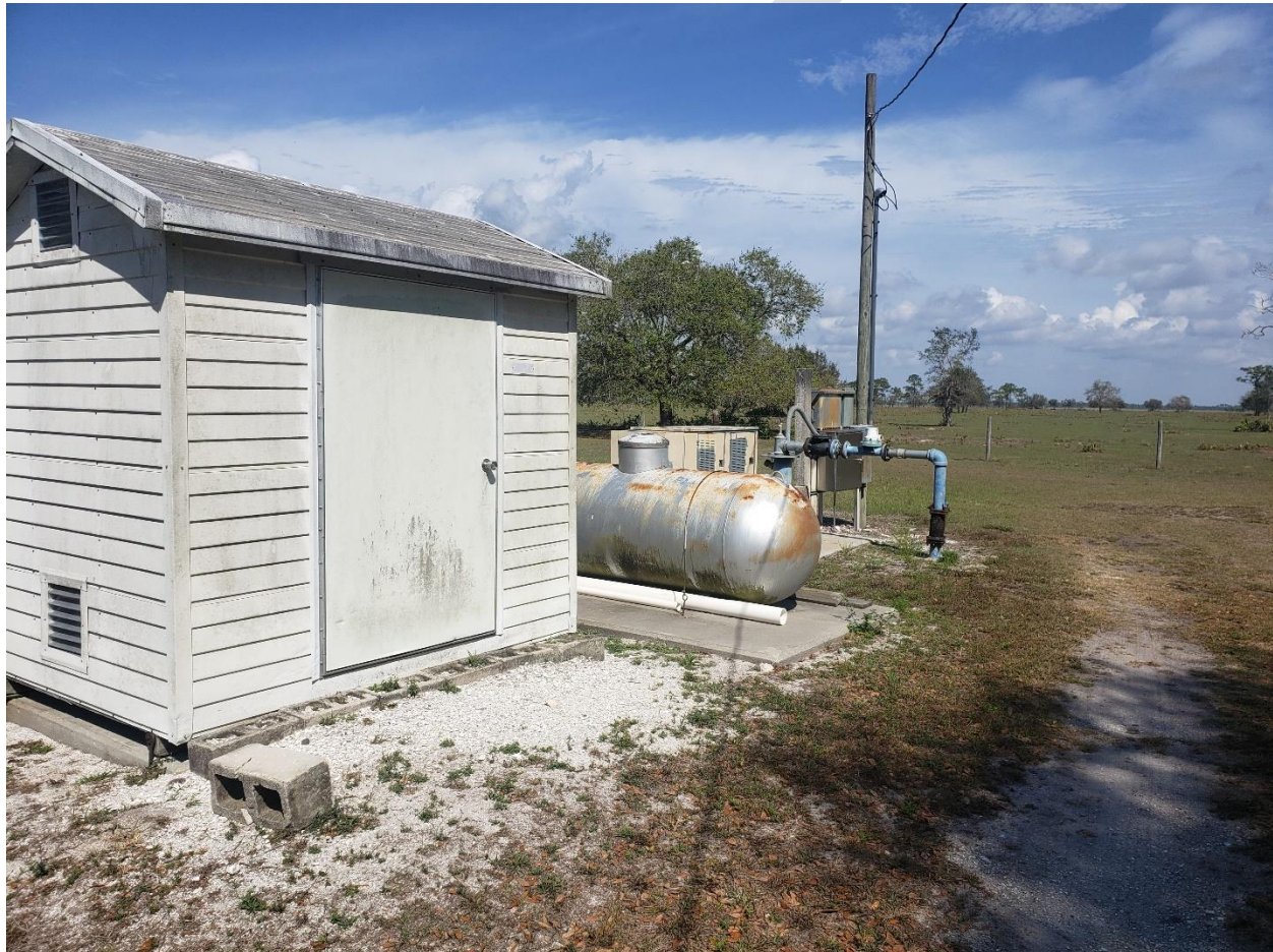
Figure 3-1 Supply Well System
