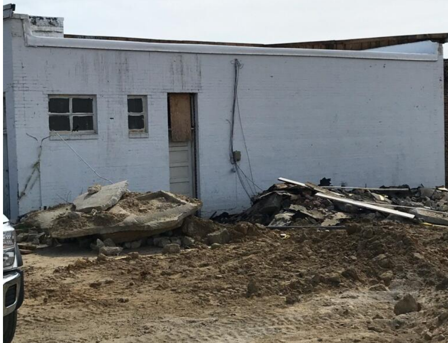
Site photo 6: Nearby construction west of driveway with concrete slab
