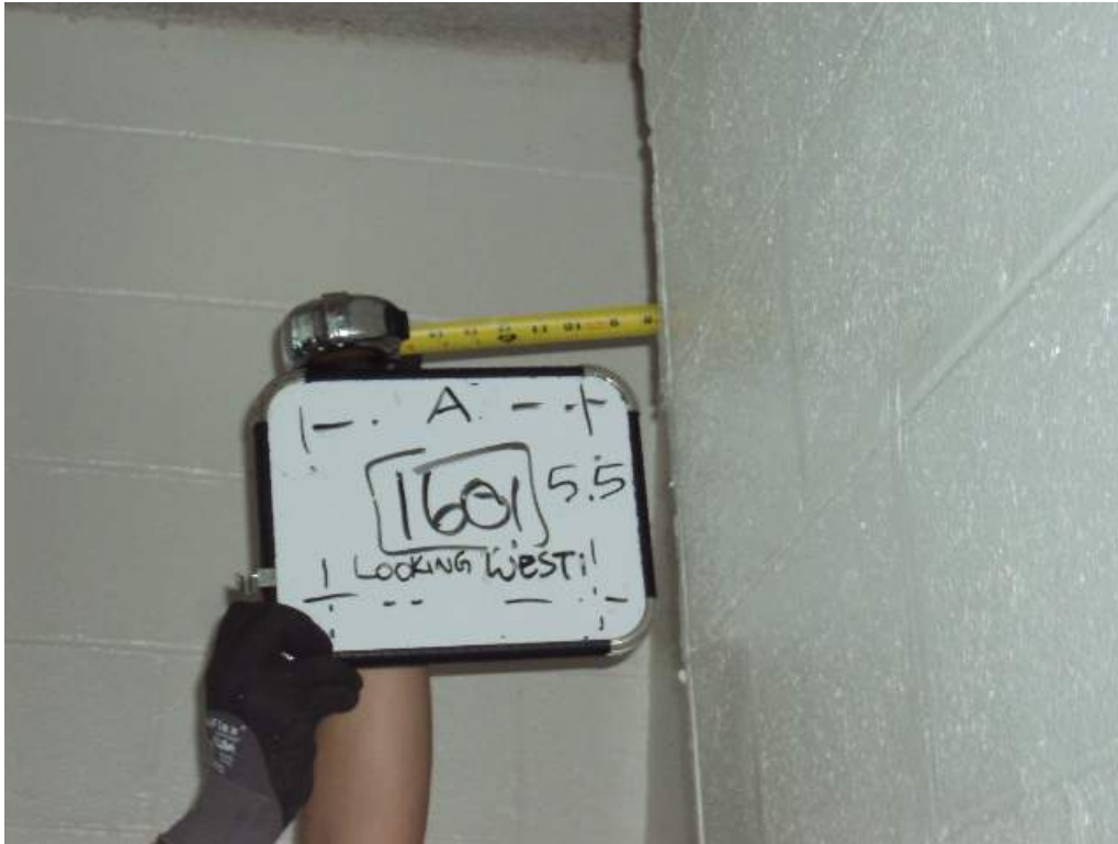
Photo 110: 1 st Floor – Room 1601– Along col line 5.5 and A – Looking West – Sheared, displaced and partially collapsed CMU wall
