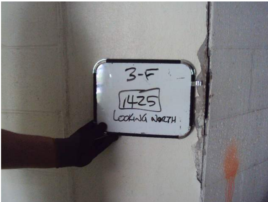
Photo 113: 1 st Floor – Room 1425– At col line 3-F – Looking North – Vertical crack between concrete col and CMU wall along with CMU displacement
