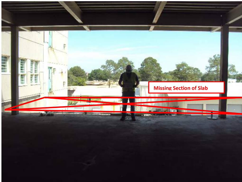
Photo 37: 3 rd Floor – Room 3206 – Looking North – Missing section of exercise concrete floor
