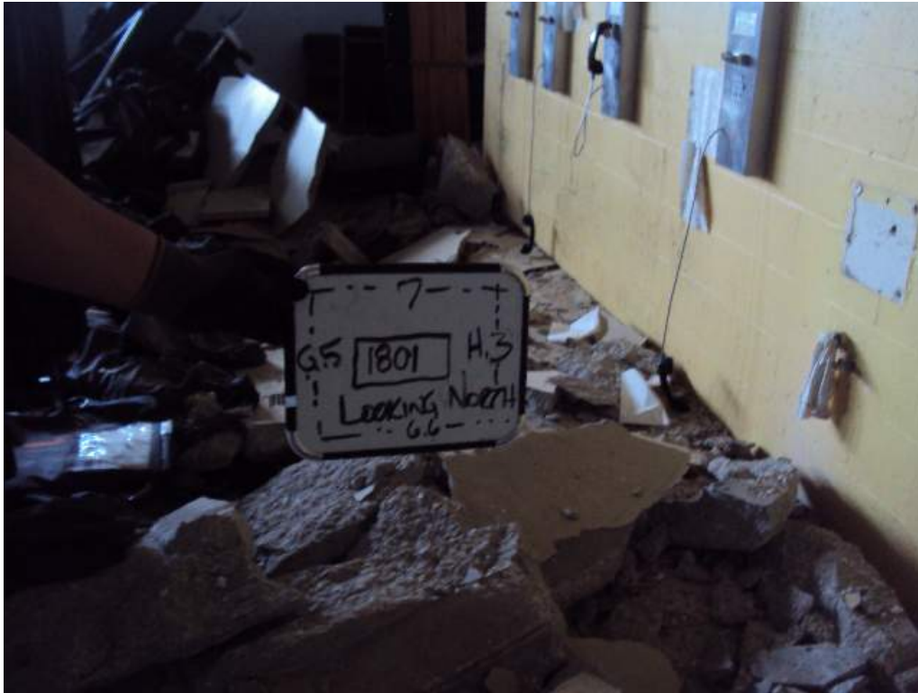
Photo 132: 1 st Floor –Room 1801 – Between column lines 6.6 and 7 & G.5 and H.3 – Looking North – Buckled, sheared and collapsed concrete slab
