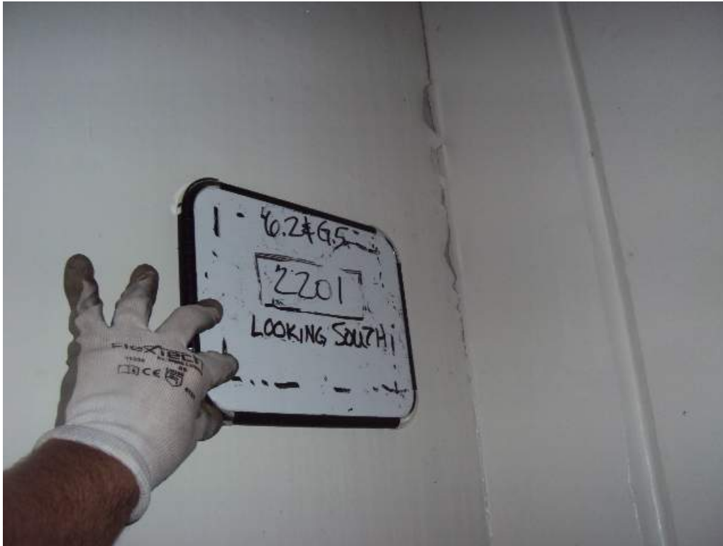
Photo 78: 2 nd Floor – Room 2201 North Dormitory – At col line 6.5 & G.5 – Looking South –Vertical crack at the CMU wall intersection
