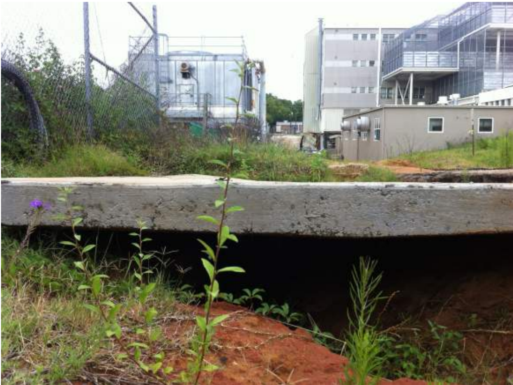
Photo 12: Northwest Concrete Slab Undermining- Looking East
