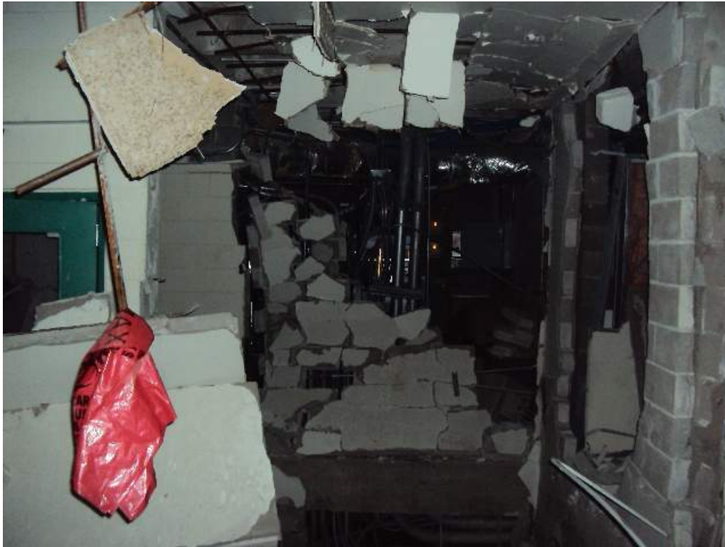
Photo 136: 1 st Floor –Room 1106 – Along col line G between col lines 4.7 and 5.5 – Looking South – Collapsed CMU walls
