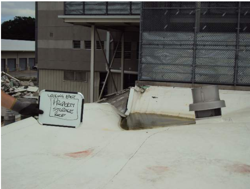
Photo 12: 1 st Floor Roof –Between col lines D and E & 7 and 8 – Looking East - Collapsed portion of roof
