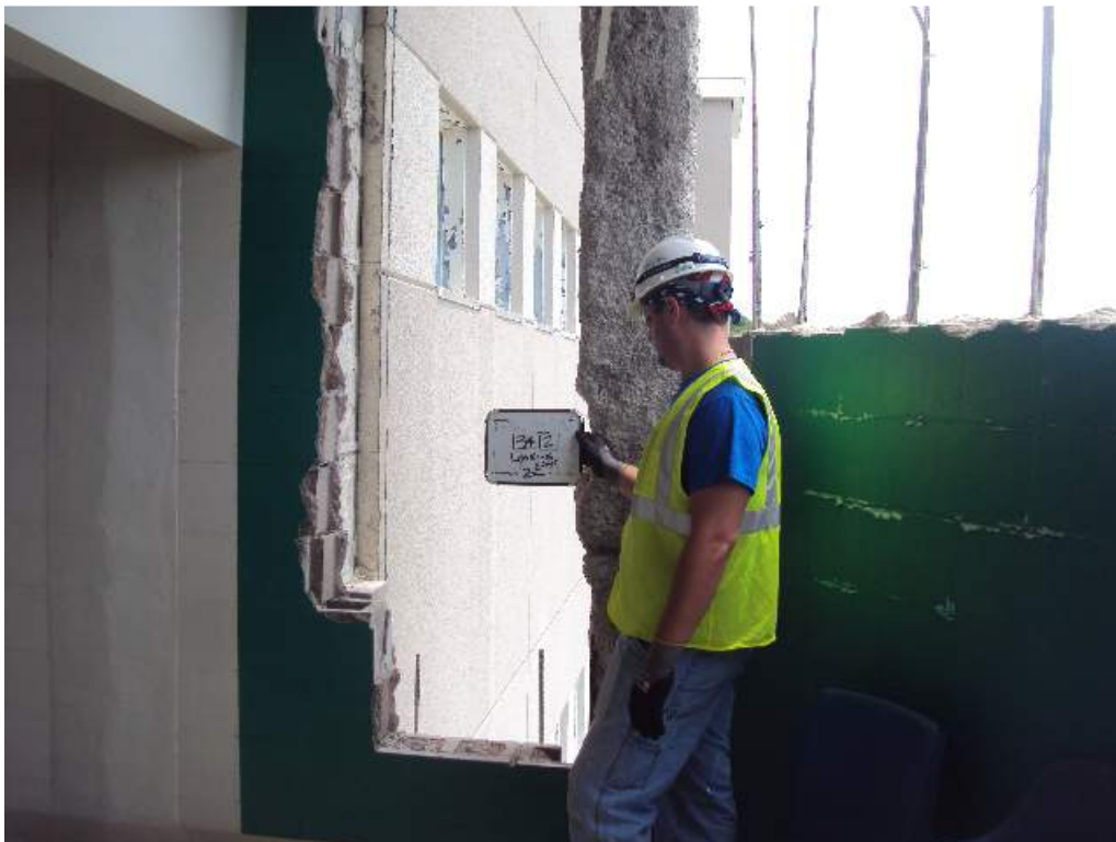
Photo 48: 3 rd Floor – Room 3412 – At col line K1.8 – Looking East – Missing portions of CMU wall with exposed reinforcement
