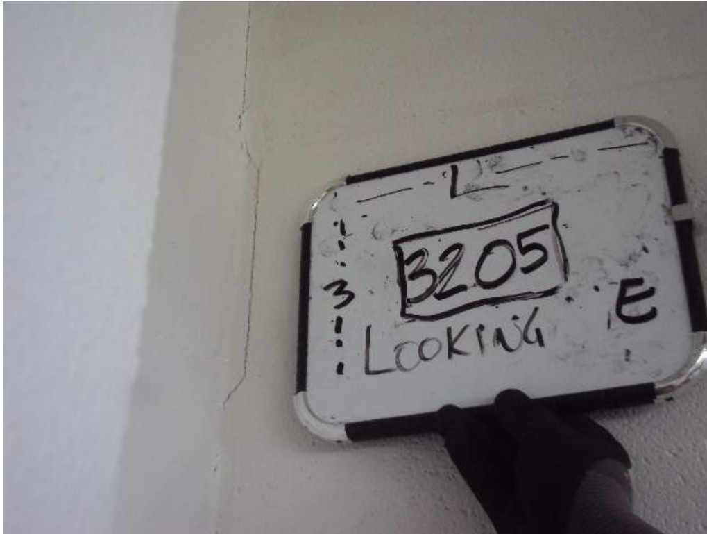
Photo 31: 3 rd Floor – Room 3205 – Along col line 3 and L – Looking East – Vertical crack between the concrete column to CMU wall
