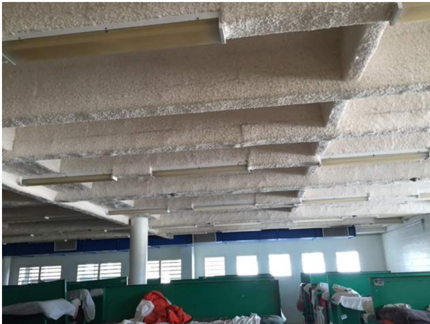
Duct work with internal insulation to be replaced- Typical for east and west wing detention areas.
