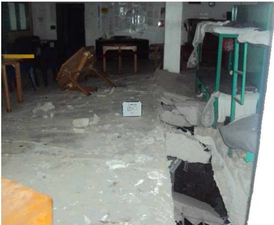
Photo 53: 2 nd Floor – Room 2201-East Dormitory –Along col line 4 between column lines L and M – Looking West - Buckled, collapsed and sheared floor slab
