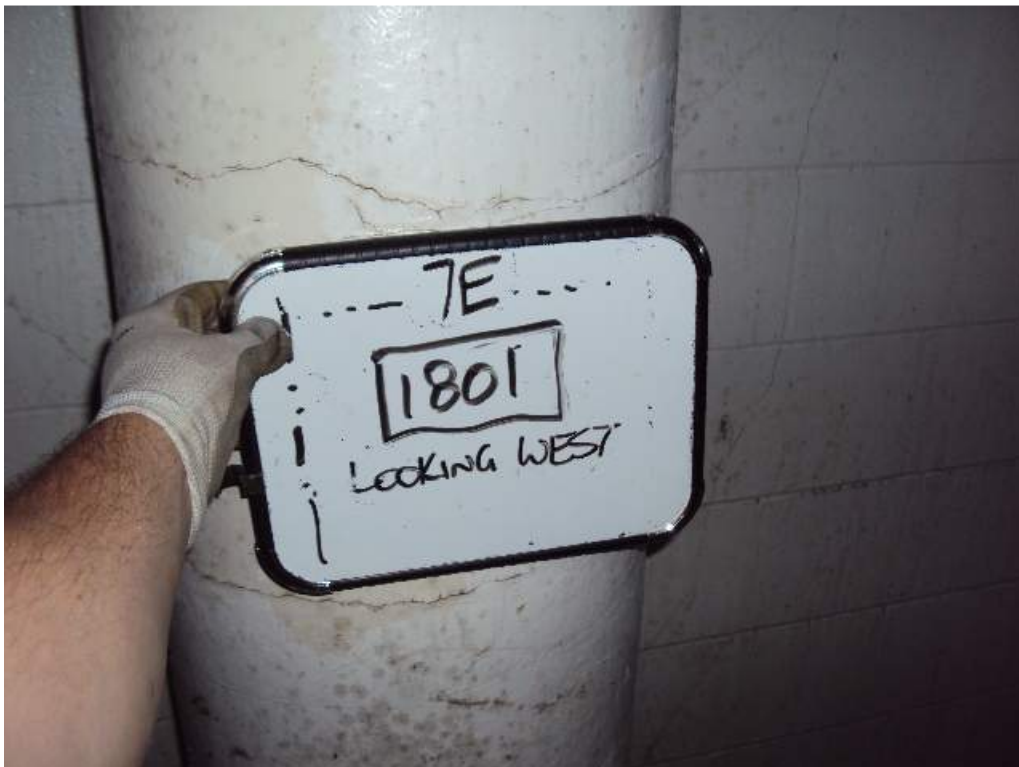
Photo 125: 1 st Floor –Room 1801 – At col line 7E – Looking West – Cracked columns
