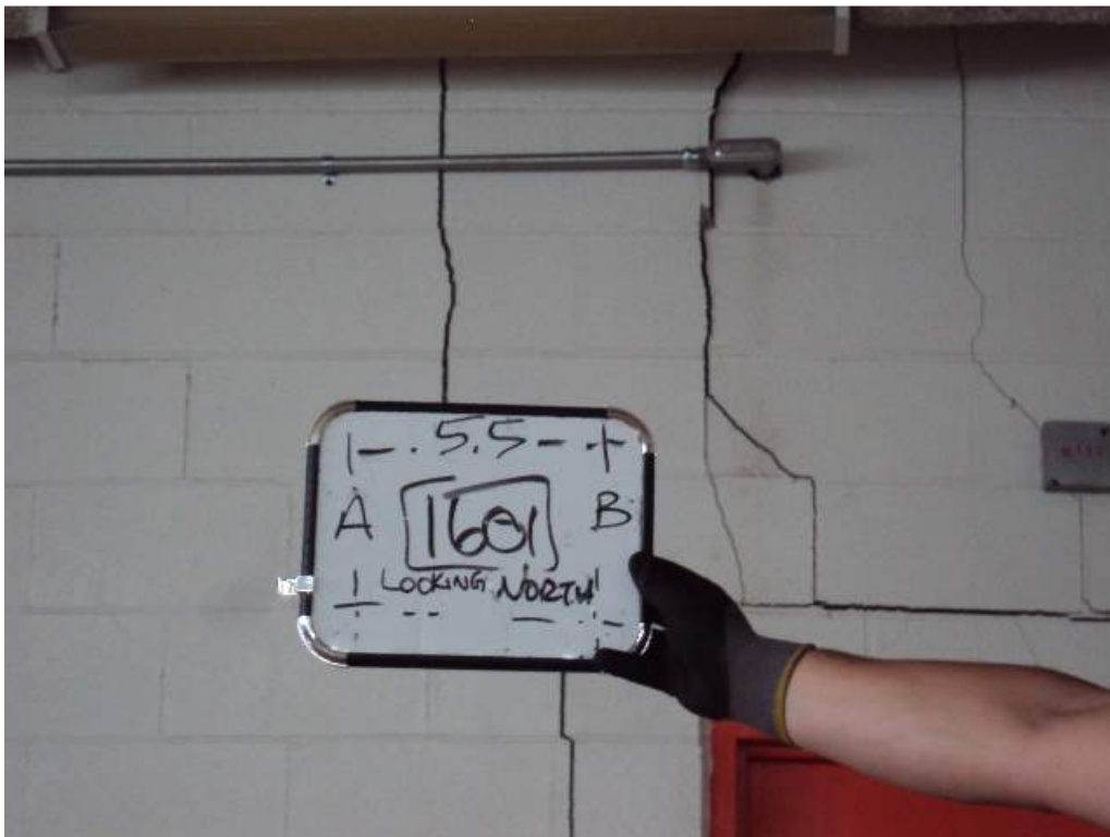
Photo 111: 1 st Floor – Room 1601– Along col line 5.5 and between A and B – Looking North – Sheared, displaced and partially collapsed CMU wall
