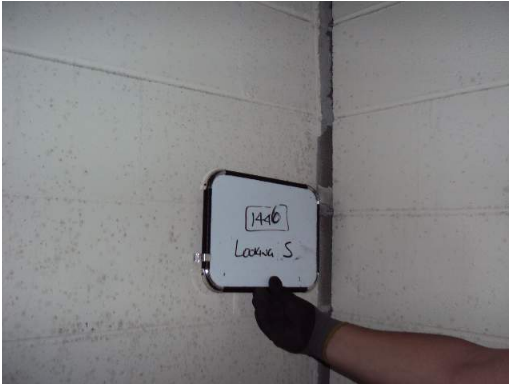
Photo 140: 1 st Floor –Room 1446 – Between column lines G and H & 5 and 5.5 – Looking South– CMU wall with horizontal translation
