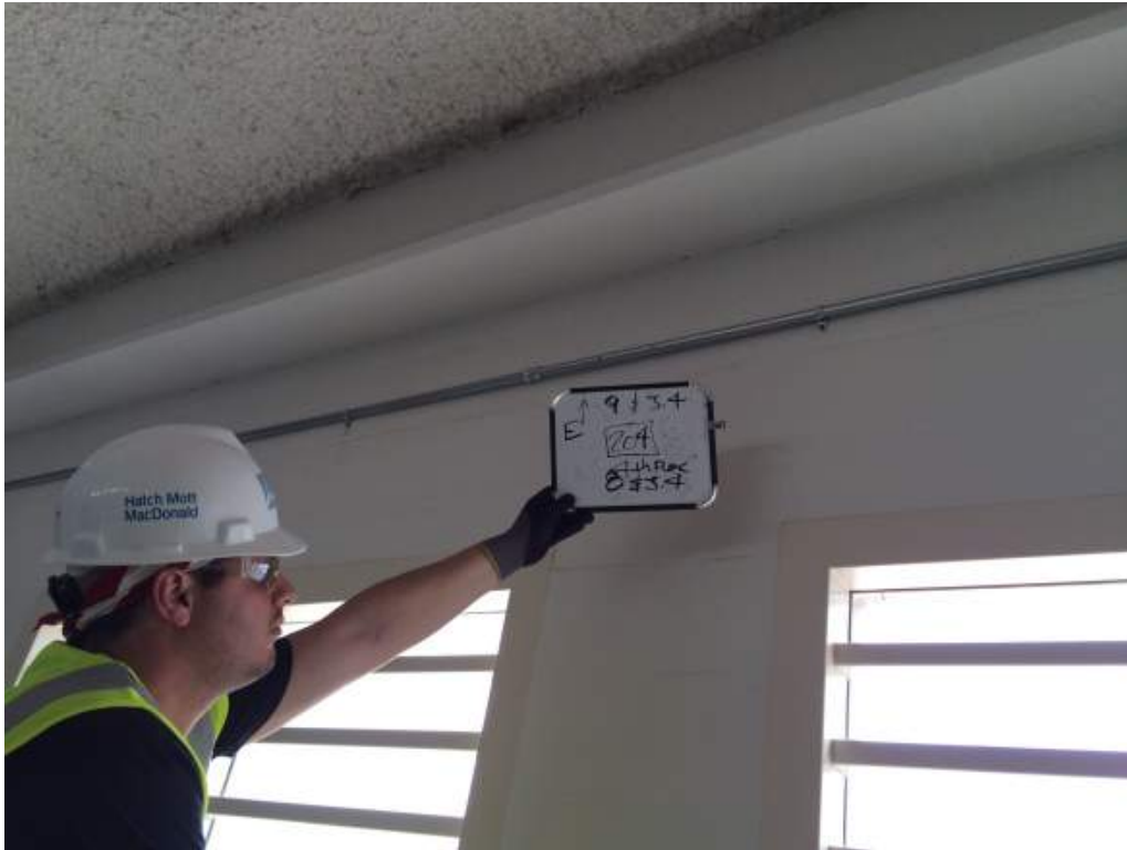
Photo 19: 4 th Floor – Room 204 –Along col Line J.4 Between 8 and 9 –Looking East– Horizontal crack @ top of CMU wall
