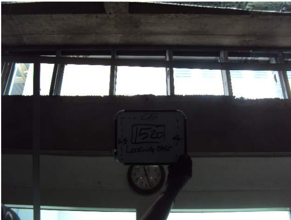
Photo 133: 1 st Floor –Room 1520 – Along col line C.5 between col lines 4 and 5.5 – Looking East – Partially collapsed exterior light gage stud wall
