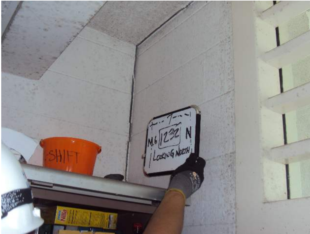
Photo 108: 1 st Floor – Room 1232– Along col line 7 between col lines M.6 and N – Looking North – Vertical and horizontal cracks in CMU walls with CMU wall displacement
