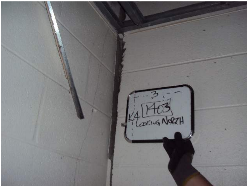
Photo 117: 1 st Floor – Room 1403– Along col line K4 adjacent to col line 3 – Looking North– Vertical crack at CMU wall corner along with wall displacement
