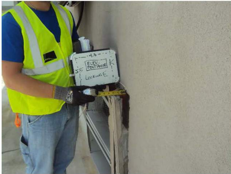
Photo 1: Elevator Penthouse –Along col line 4.3 between col lines J.5 and K – Looking East - Damaged exhaust vent and wall section at the elevator shaft
