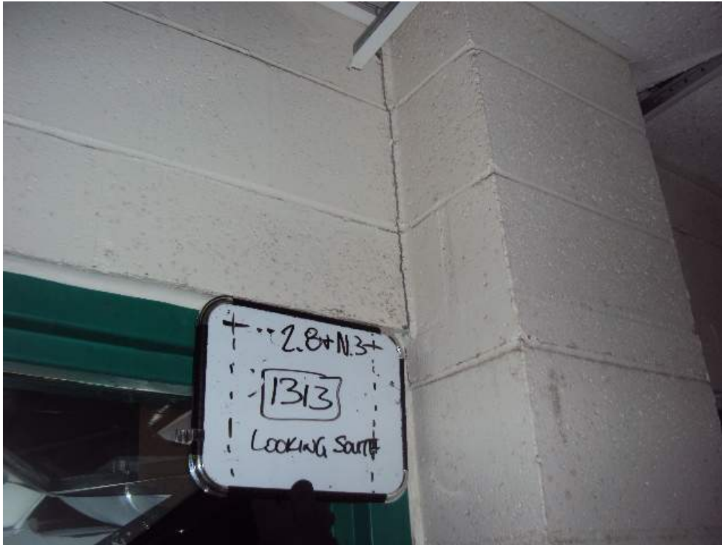
Photo 104: 1 st Floor – Room 1313– At col line 2.8 and N.3 – Looking South – Vertical crack in CMU wall
