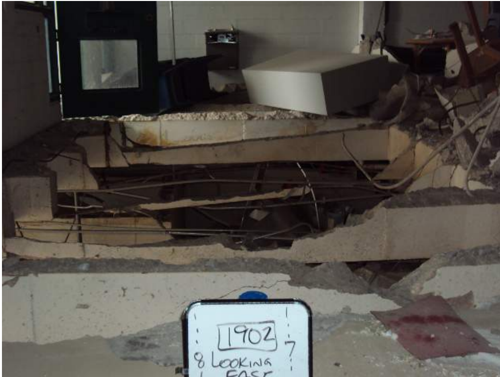
Photo 142: 1 st Floor –Room 1902 – Between column lines J.5 and L & 6.6 and 8 – Looking East– Collapsed concrete floor
