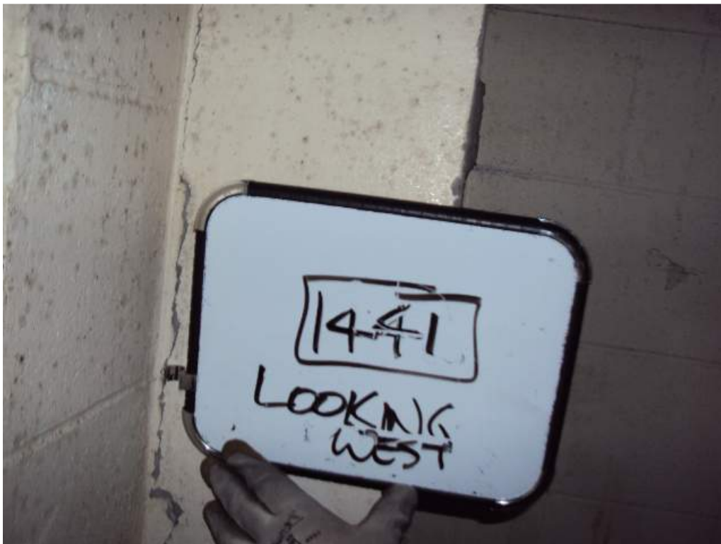
Photo 141: 1 st Floor –Room 1441 – At column lines K.4 and 6.6 – Looking West– Vertical crack between concrete column and CMU wall
