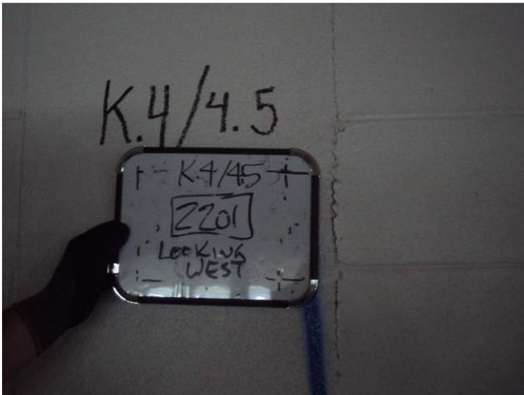
Photo 65: 2 nd Floor – Room 2201 – East Dormitory – At column line 4.5&K.4-Looking West-Vertical cracks between a concrete column and CMU wall
