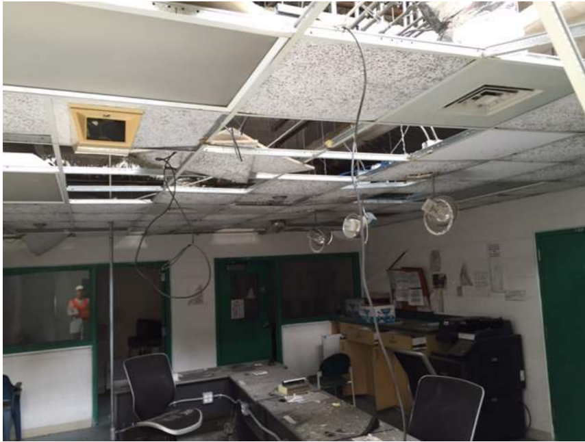
First floor control area lighting fixture damage.
