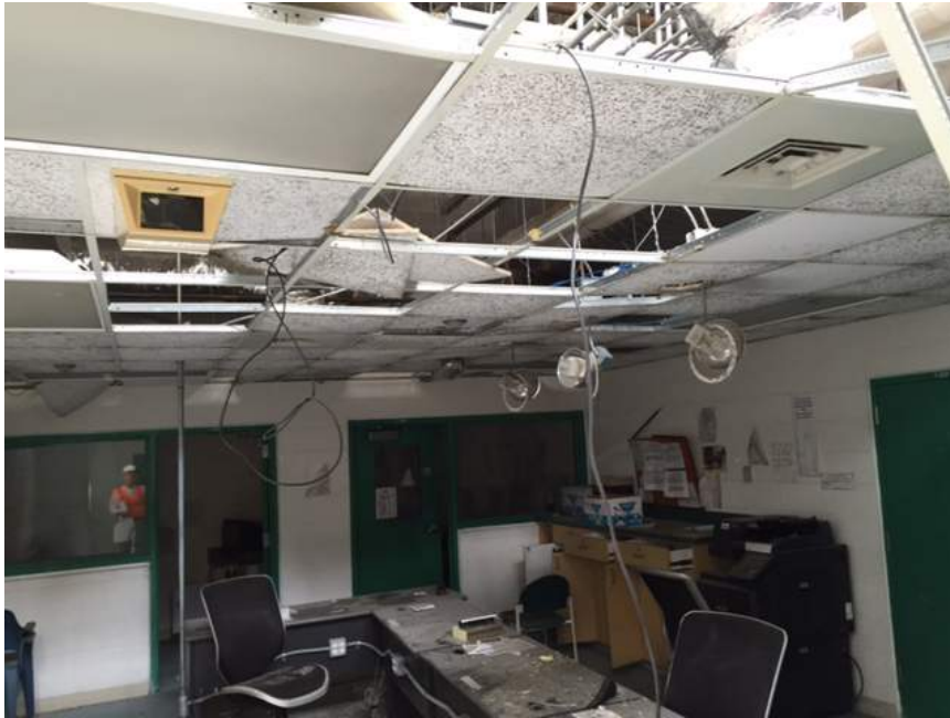
First floor- Exposed duct work to be reinsulated.
