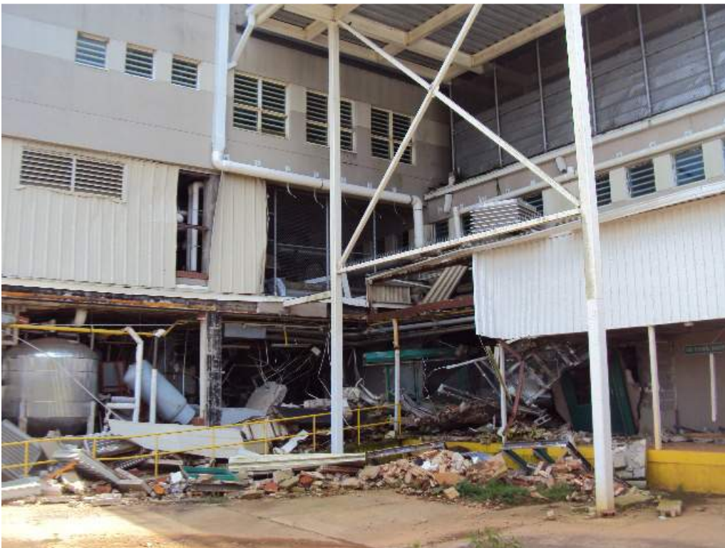
Photo 157: Basement –Room 140, 141 and 143– Between col lines G.5 and H.3 & 8 and 10 – Looking Southeast– Collapsed CMU walls and walkway roofs
