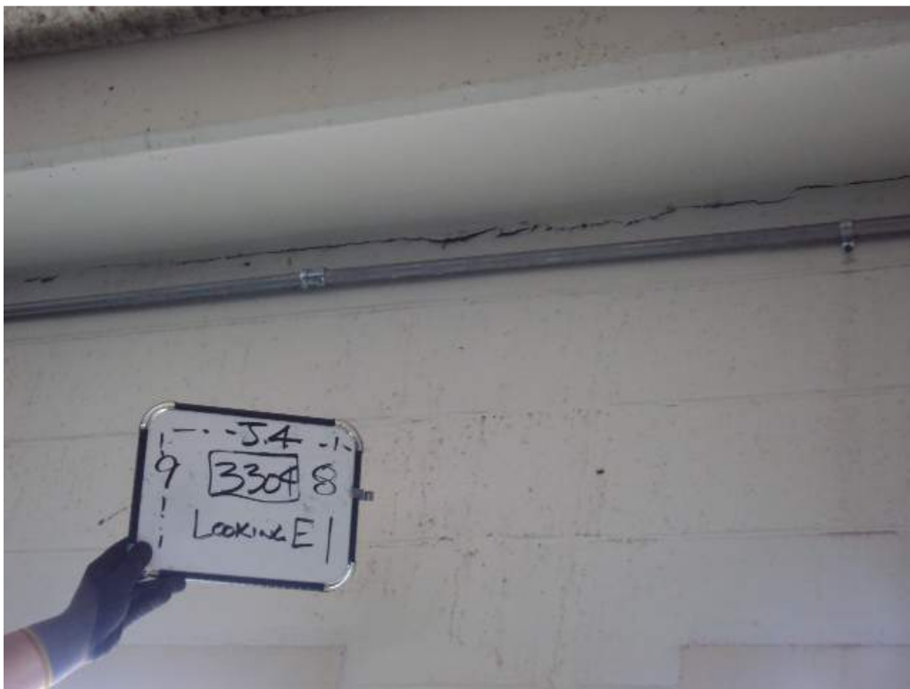
Photo 40: 3 rd Floor – Room 3304 – Along col line J.4 between col lines 8 and 9 –Looking East – Horizontal crack between the concrete beam and CMU wall
