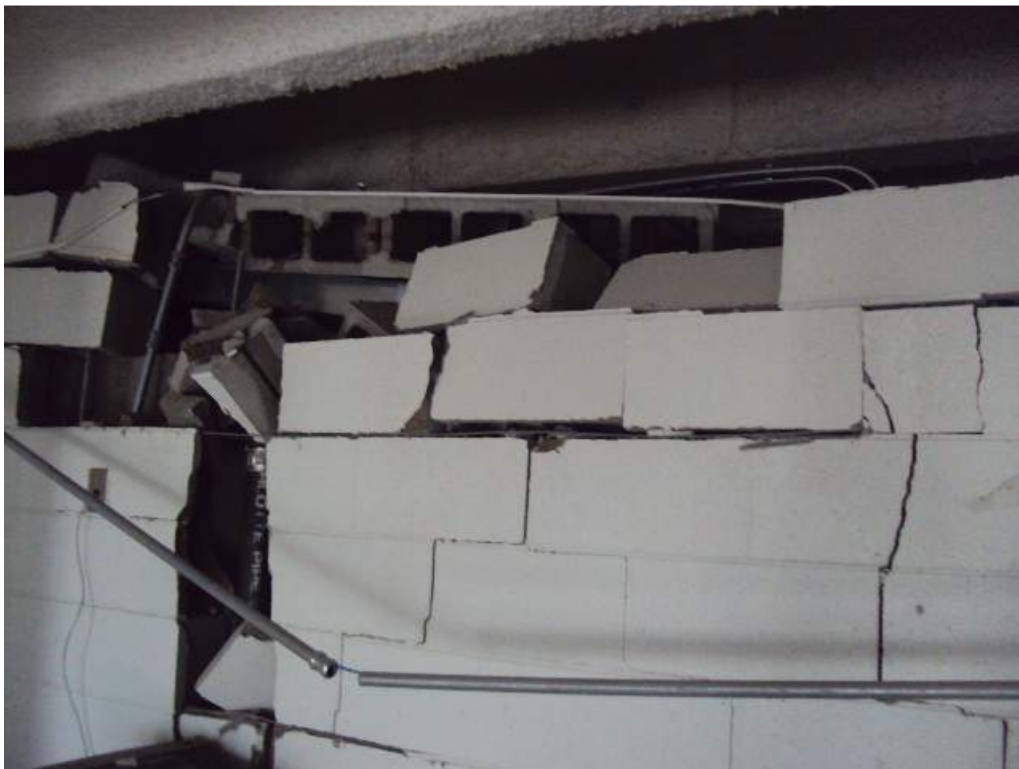
Photo 145: 1 st Floor –Room 1902 – Along col line 6.6 between col lines J.5 and L – Looking South– Collapsed CMU wall
