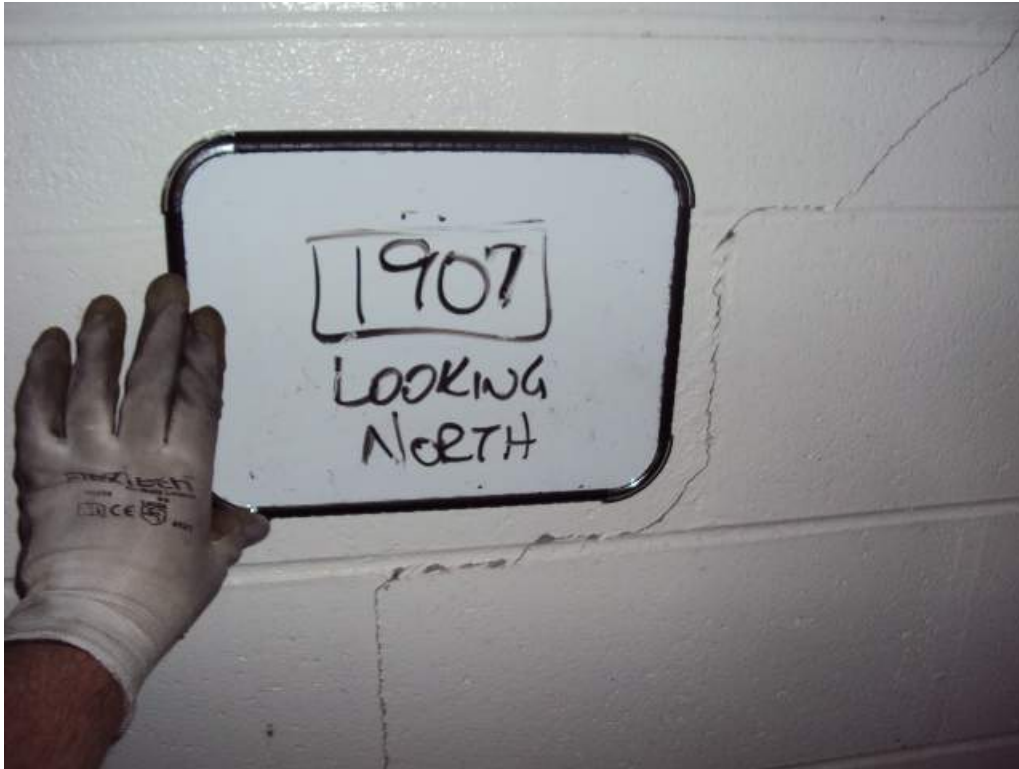
Photo 146: 1 st Floor –Room 1907 – Along col line 8 between col lines H.5 and J.5 – Looking North– Stair step crack in CMU wall
