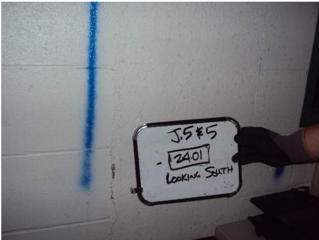
Photo 87: 2 nd Floor – Room 2401– At col lines J.5 and 5 – Looking South –Vertical crack between conc col and CMU wall
