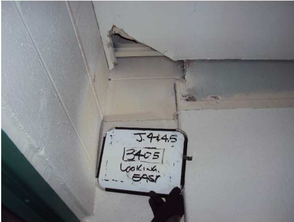
Photo 45: 3 rd Floor – Room 3405 – At col line J.4 and 4.5 – Looking East – Crack at CMU wall corner & between concrete col and CMU wall
