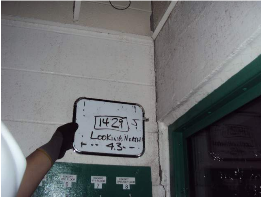
Photo 114: 1 st Floor – Room 1429– At col line J and 4.3 – Looking North – Vertical crack at corner of CMU wall
