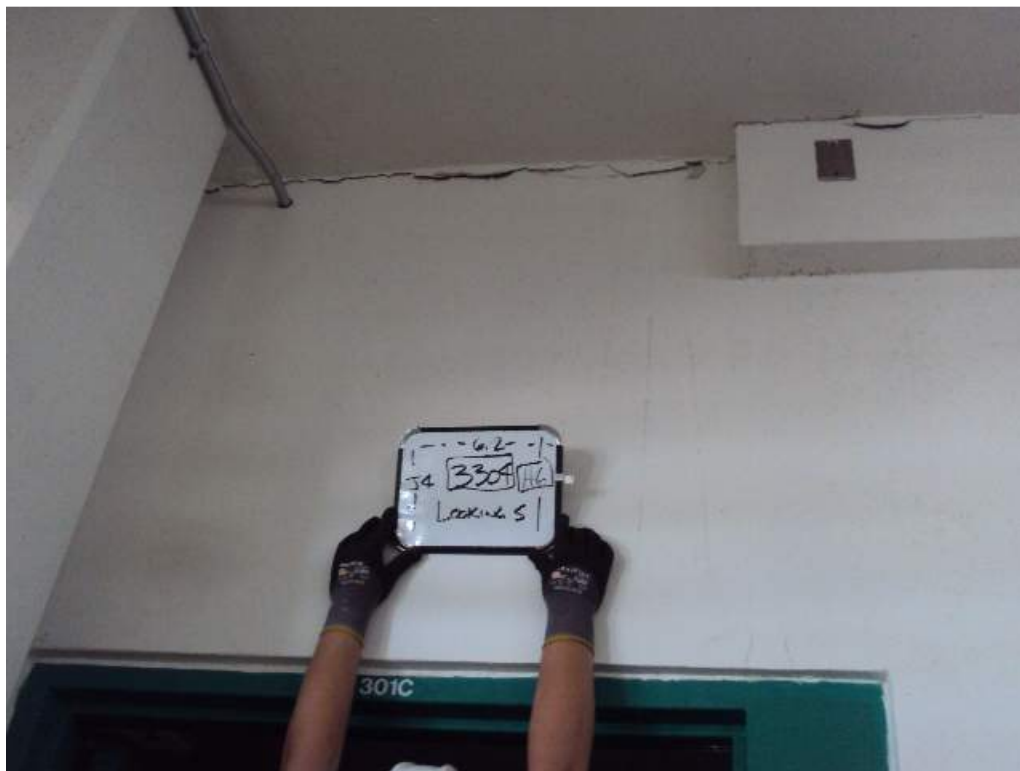
Photo 38: 3 rd Floor – Room 3304 – Along col line 6.2 between col lines H.6 and J.4 – Looking South – Horizontal crack at top of CMU wall
