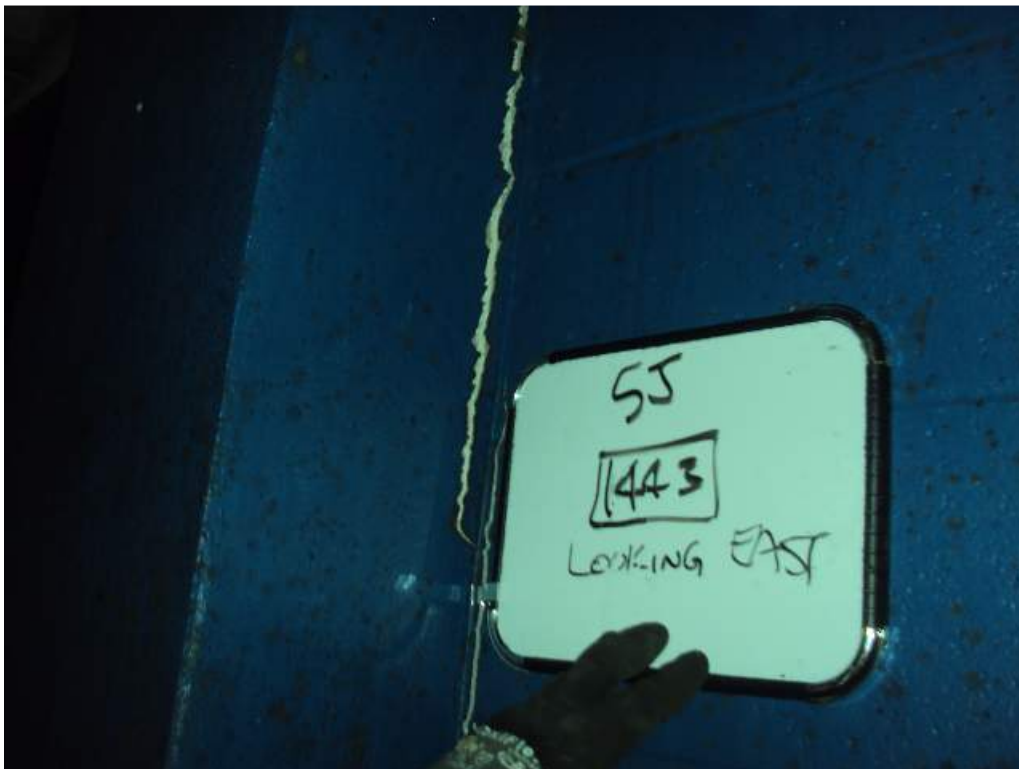
Photo 137: 1 st Floor –Room 1443 – At column line 5J – Looking East – Vertical crack between concrete column and CMU wall
