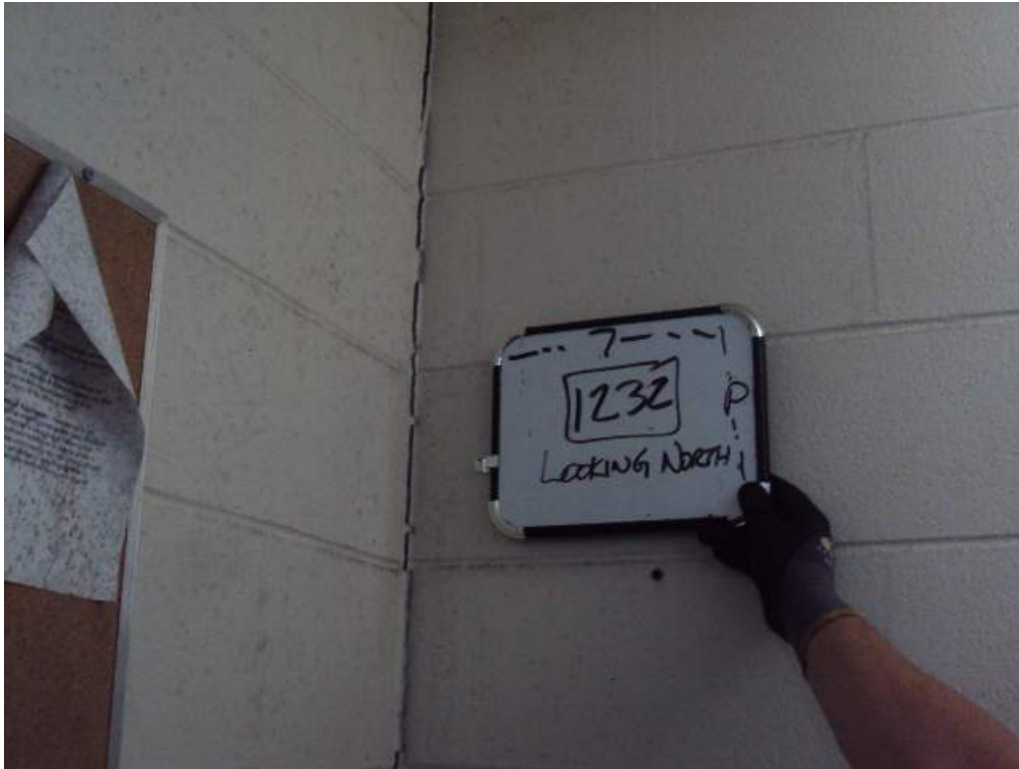
Photo 106: 1 st Floor – Room 1232– Along col line 7 adjacent to P – Looking North – Vertical crack at corner of CMU wall
