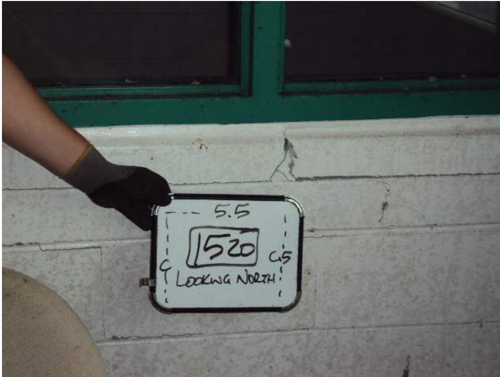
Photo 134: 1 st Floor –Room 1520 – Along col line 5.5 between col lines C and C.5 – Looking North – Stair step crack in CMU wall
