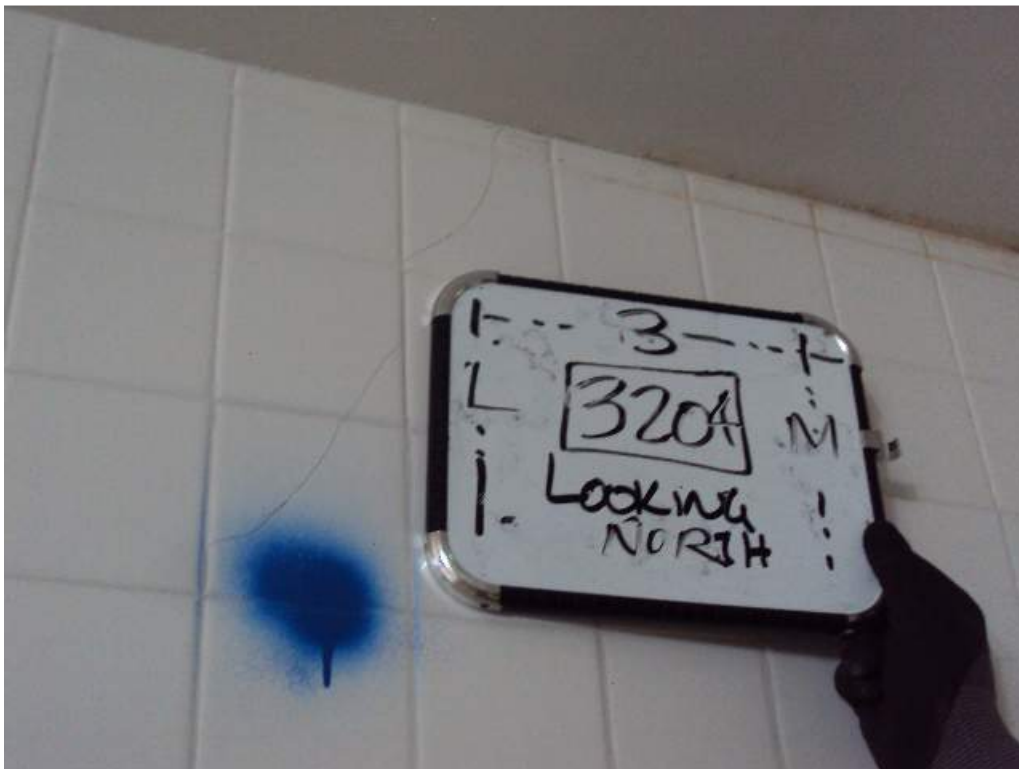
Photo 36: 3 rd Floor – Room 3204 – Along col line 3 between L and M – Looking North – Stair step crack in tile in restroom walls
