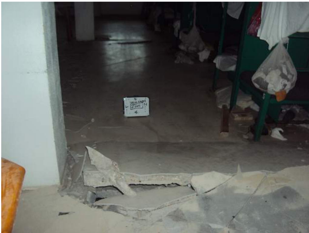
Photo 57: 2 nd Floor – Room 2201-East Dormitory –Between column lines 4 and 5 & L and M - Looking North - Buckled, collapsed and sheared floor slab
