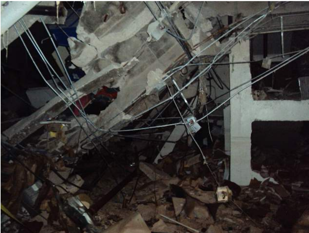
Photo 155: Basement –Room 128, 129 & 132– Between col lines J.5 and K.8 & 3 and 5 – Looking South– Collapsed CMU walls and floor slabs
