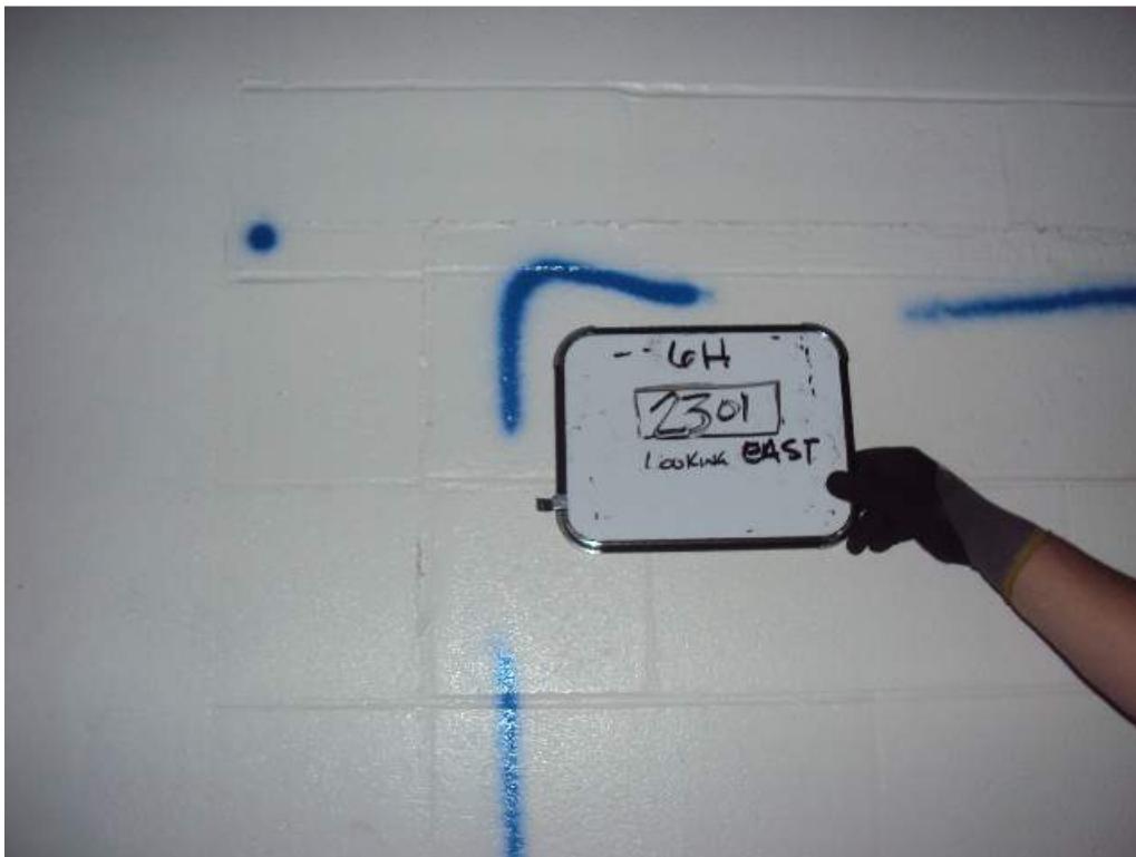
Photo 73: 2 nd Floor – Room 2301 – At col line 6H-Looking East –Stair step cracks in CMU wall
