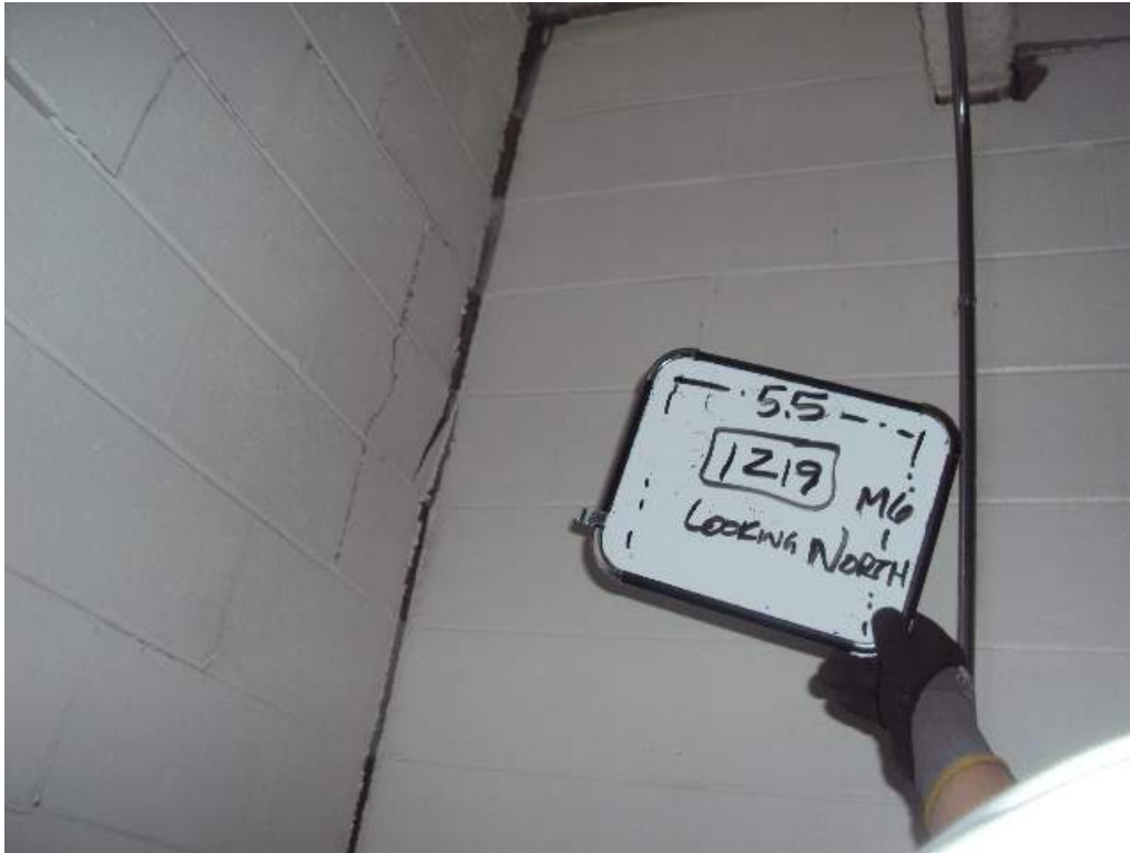
Photo 98: 1 st Floor – Room 1219– Along col line 5.5 adjacent to M6– Looking North-Partially collapsed CMU wall
