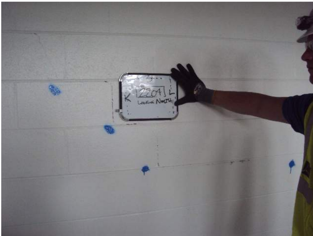
Photo 69: 2 nd Floor – Room 2204 – Along col line 3 between col lines L and M-Looking North –Stair step crack in CMU wall
