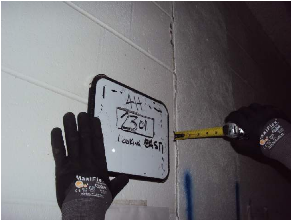
Photo 74: 2 nd Floor – Room 2301 – At col line 4H-Looking East –Vertical crack between conc col and CMU wall and CMU wall displacement
