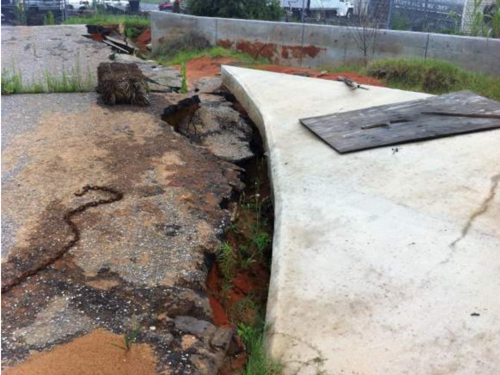
Photo 11: Northwest Concrete Landing Undermining- Looking Southwest
