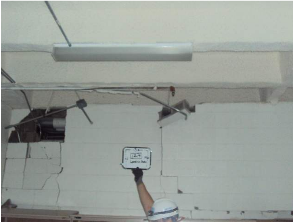
Photo 96: 1 st Floor – Room 1219– Along col line 3.4 between col lines M.6 and N– Looking South– Partially collapsed CMU wall
