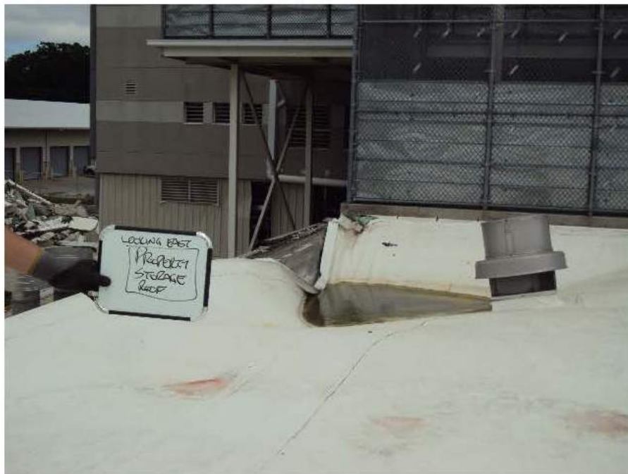
Photo 2: 1 st Floor Roof –Between col lines D and E & 7 and 8 – Looking East - Collapsed portion of roof
