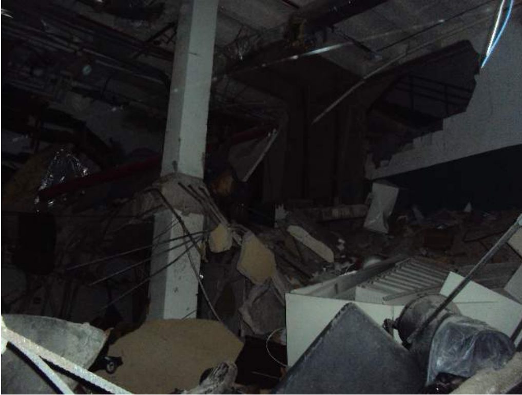
Photo 154: Basement –Room 132– Between col lines K.2 and M & 3 and 6 – Looking South– Collapsed CMU walls and floor slabs
