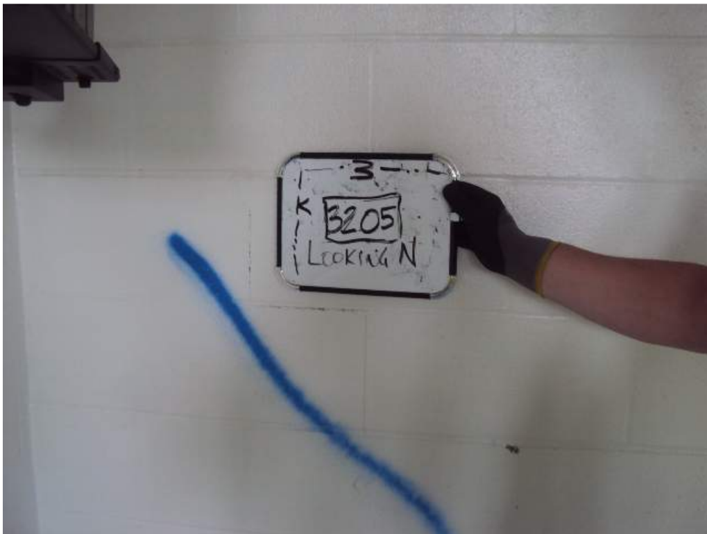
Photo 32: 3 rd Floor – Room 3205 – Along col line 3 and K – Looking North – Stair step crack in CMU wall
