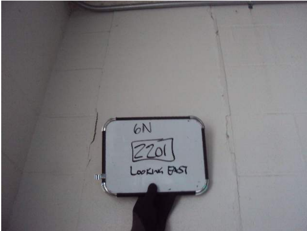
Photo 60: 2 nd Floor – Room 2201-East Dormitory –At col line 6N - Looking East – Vertical cracks between concrete column and CMU walls
