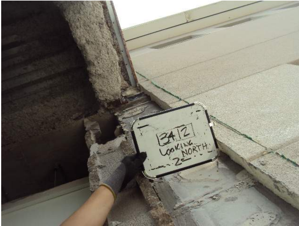
Photo 49: 3 rd Floor – Room 3412 – At col line K2 – Damaged bolt connecting beam to col
