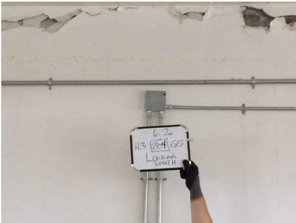
Photo 14: 4 th Floor – Room 204 –Along col Line 6.2 between G.5 & H.3 – Looking South – Horizontal crack @ top of CMU wall
