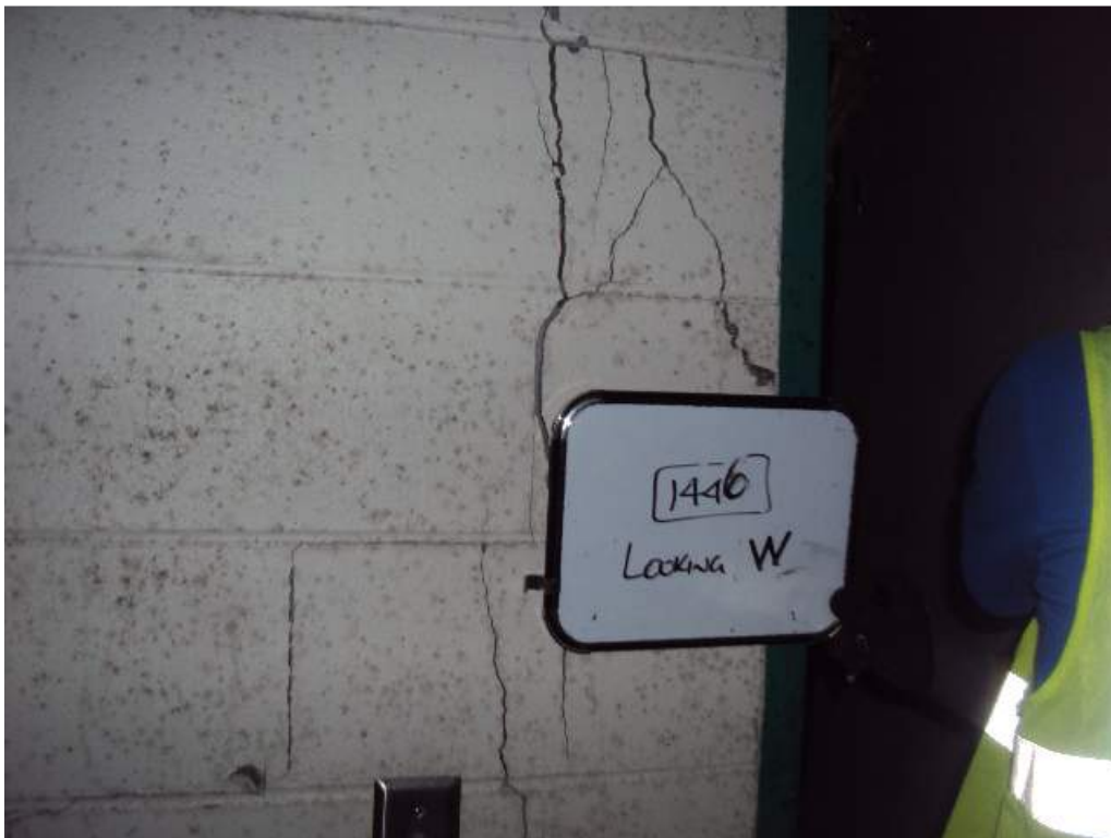
Photo 139: 1 st Floor –Room 1446 – Between column lines G and H & 5 and 5.5 – Looking West– Severe map cracking in CMU wall
