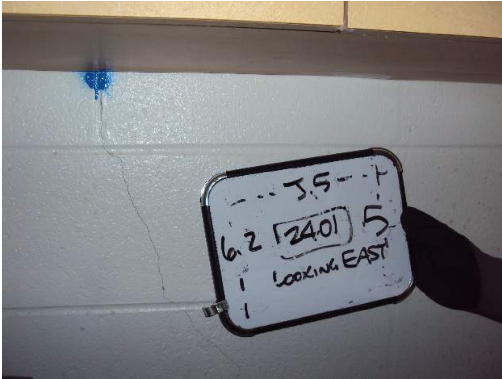
Photo 86: 2 nd Floor – Room 2401– Along col line J.5 between col lines 5 and 6.2 – Looking East –Stair step/vertical crack in CMU wall
