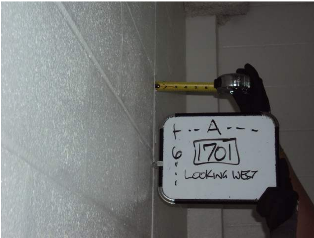
Photo 121: 1 st Floor – Room 1701– Along col line 6 adjacent to A – Looking West– Displaced CMU wall
