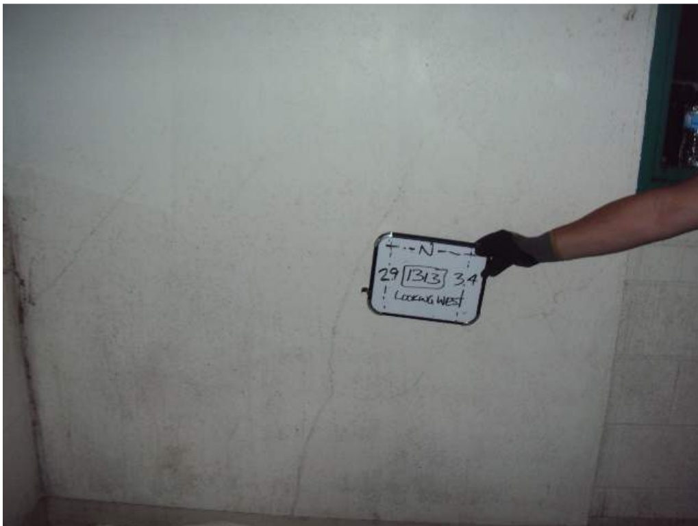
Photo 103: 1 st Floor – Room 1313– Adjacent to col lines N and 2.9 and 3.4 – Looking West – Map cracking in wall
