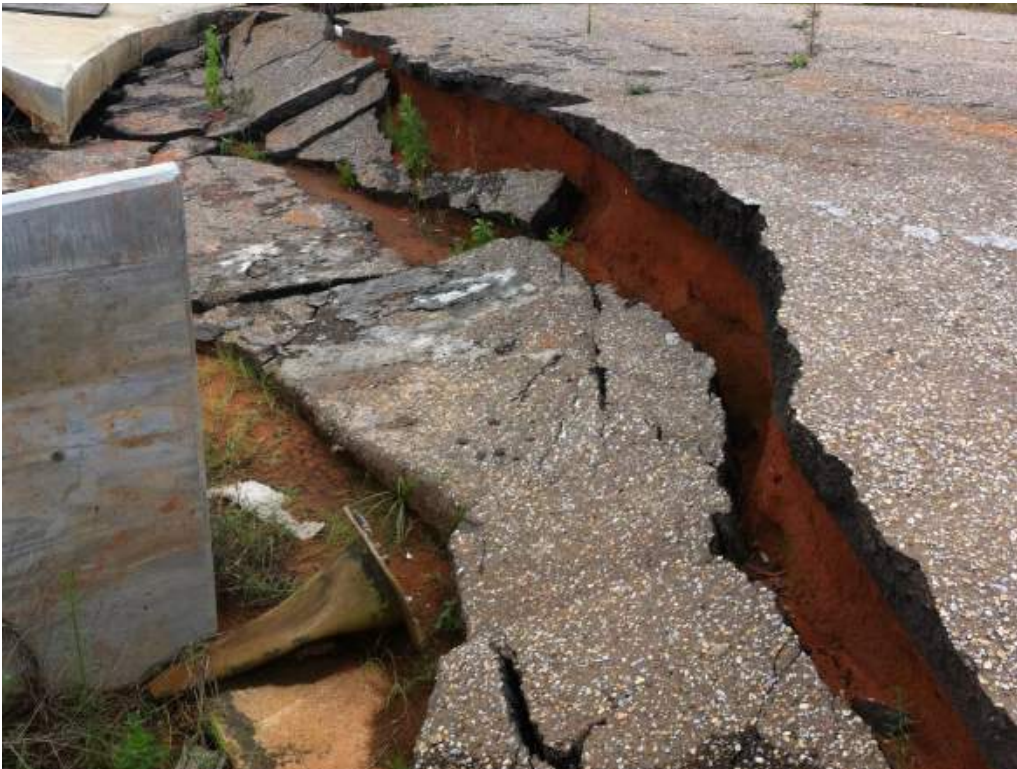
Photo 14: Northwest Access Road Erosion- Looking Northwest
