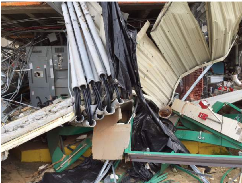
Basement view looking north. Electric Boiler feeders with main distribution switchboard in background.
