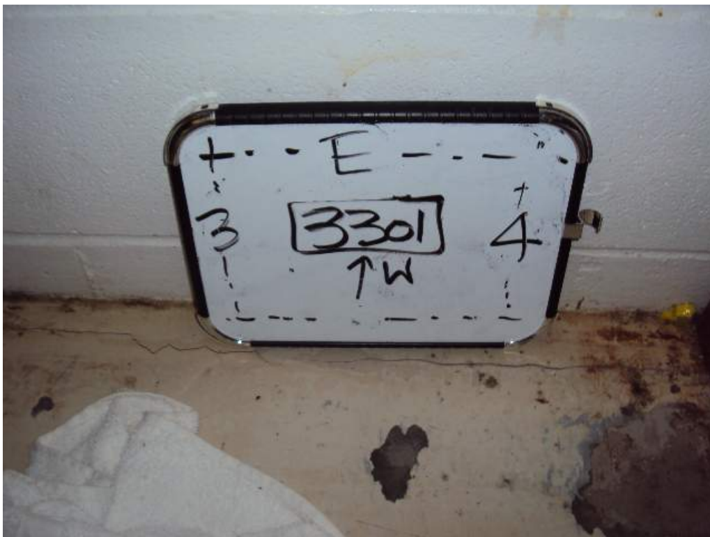
Photo 42: 3 rd Floor – Room 3301 – Along col line E between col lines 3 and 4 –Cracks in floor slab
