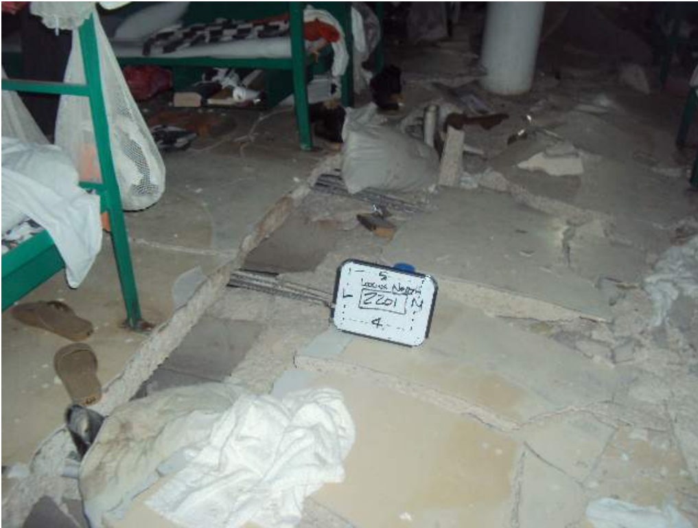
Photo 58: 2 nd Floor – Room 2201-East Dormitory –Between column lines 4 and 5 & L and M - Looking North - Buckled, collapsed and sheared floor slab
