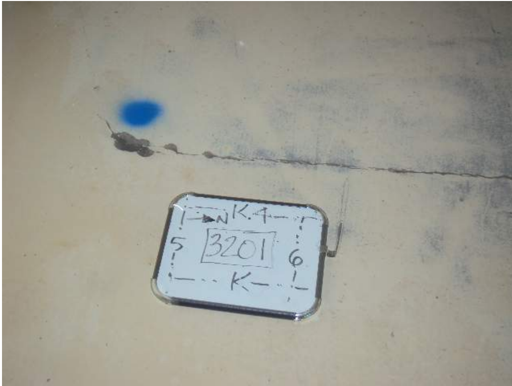
Photo 27: 3 rd Floor- Room 3201 – Between col lines K and K.4 & 5 and 6- Crack in the floor slab
