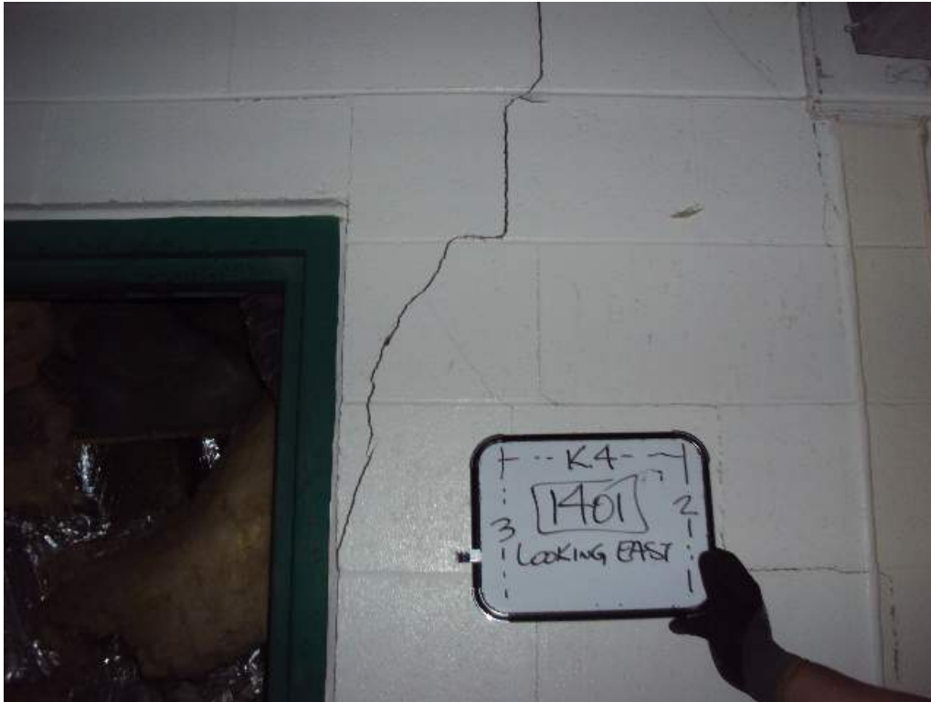
Photo 116: 1 st Floor – Room 1401– Along col line K4 between col lines 2 and 3 – Looking East– Stair step crack in CMU wall
