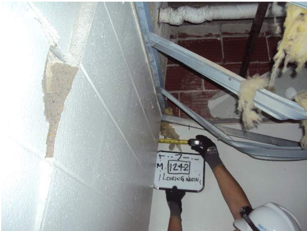
Photo 109: 1 st Floor – Room 1242– Along col line 7 and M – Looking North – Sheared, displaced and partially collapsed CMU wall
