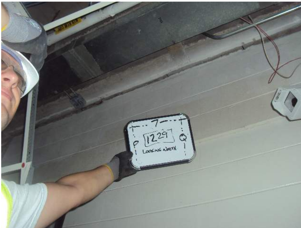
Photo 95: 1 st Floor – Room 1229– Along col line 7 between col lines P and Q– Looking North–Displaced CMU wall between col lines P and Q
