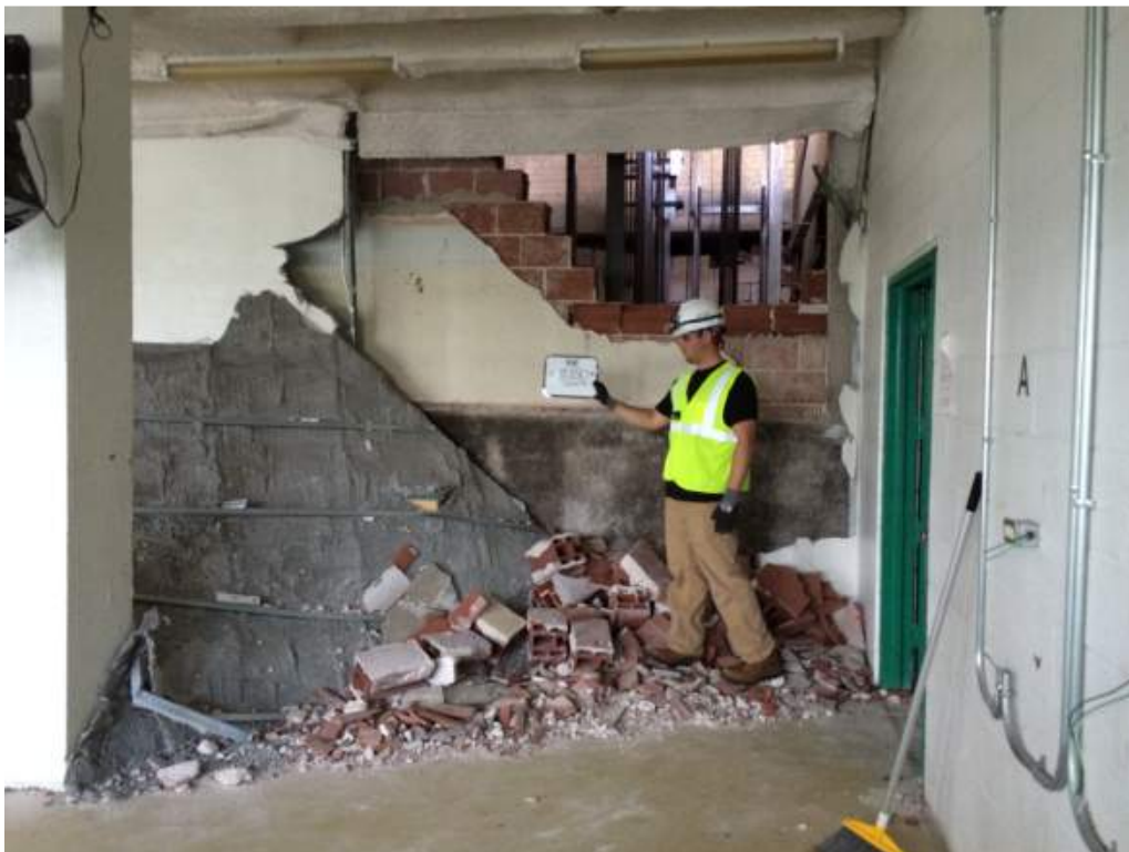
Photo 20: 4 th Floor – Room 4201 – Along col line 4.5 between J.4 and K – Looking South – Demolished elevator CMU wall
