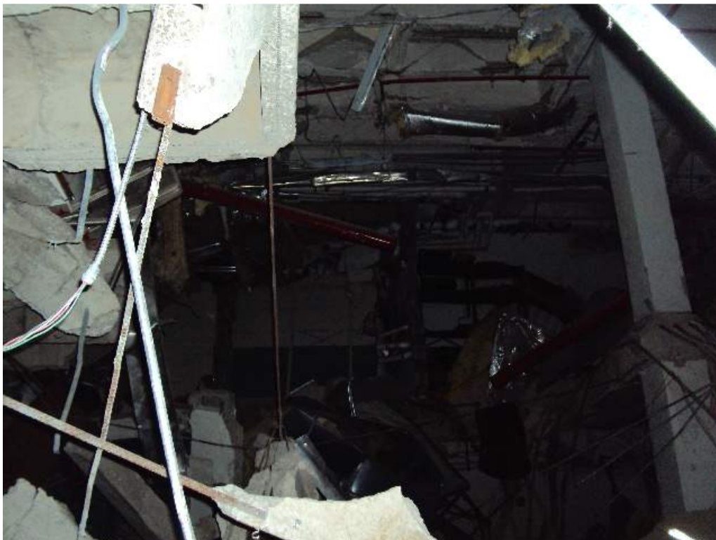
Photo 153: Basement –Room 132– Between col lines K.2 and M & 3 and 6 – Looking South– Collapsed CMU walls and floor slabs
