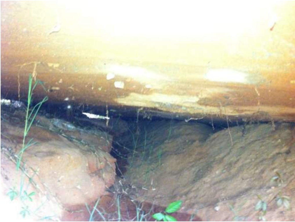
Photo 13: Northwest Concrete Slab Complete Undermining- Looking East
