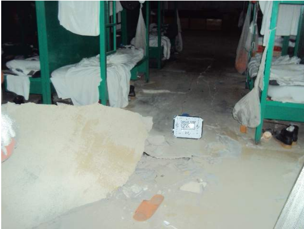
Photo 56: 2 nd Floor – Room 2201-East Dormitory –Between column lines 5 and 6 & L and M - Looking West - Buckled, collapsed and sheared floor slab
