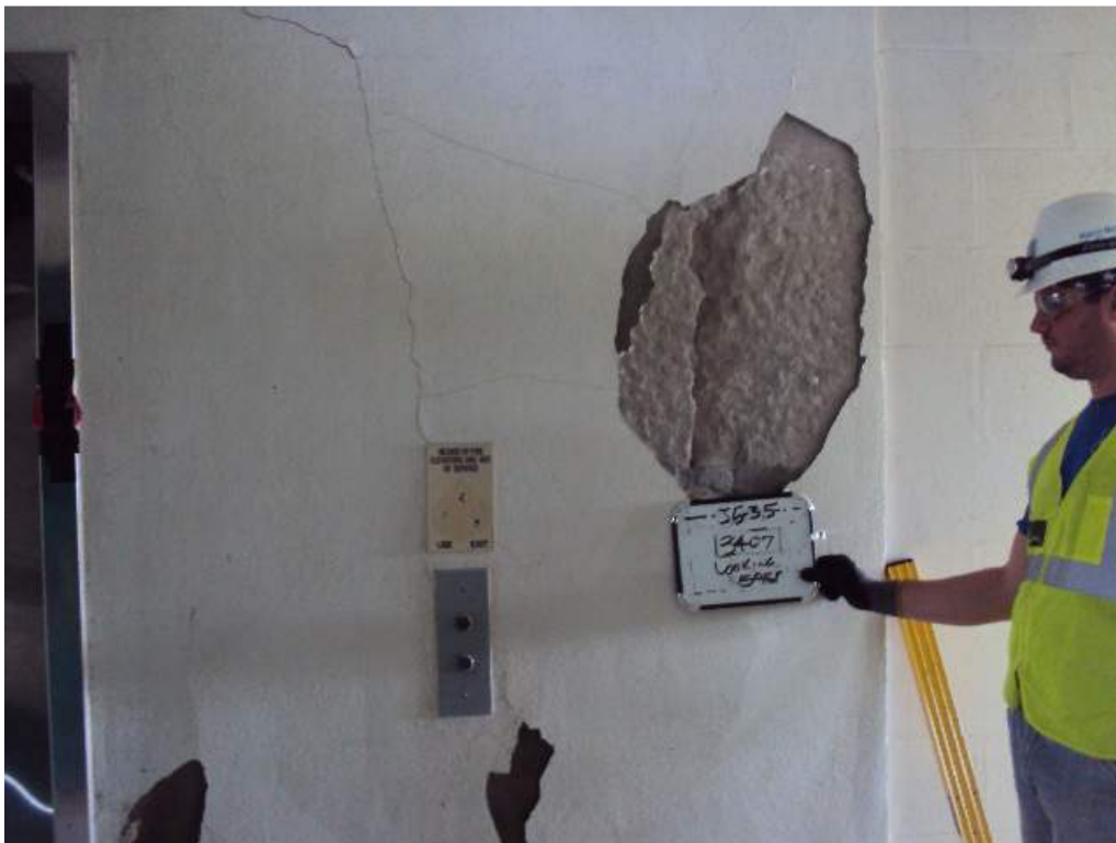
Photo 46: 3 rd Floor – Room 3407 – Adjacent to col line J.5 and 3.5 – Looking East – Map cracking in elevator CMU wall
