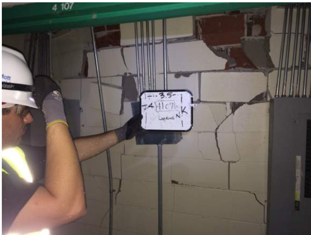
Photo 24: 4 th Floor – Room 4107 – Along col line 3.5 between J.4 and K – Looking North – Collapsed elevator CMU wall
