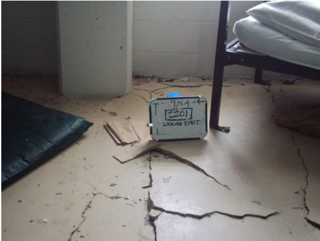
Photo 84: 2 nd Floor – Room 2201 North Dormitory – At col line 9 and J4 – Looking East – Buckled, Cracked and Shear floor slabs
