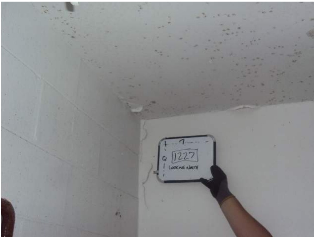
Photo 93: 1 st Floor – Room 1227– Adjacent to col line 7Q– Looking North–Vertical cracks at CMU wall corner
