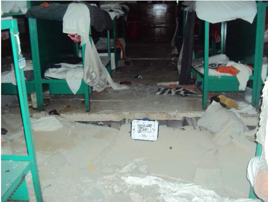
Photo 54: 2 nd Floor – Room 2201-East Dormitory –Between column lines 4 and 5 & L and M - Looking West - Buckled, collapsed and sheared floor slab
