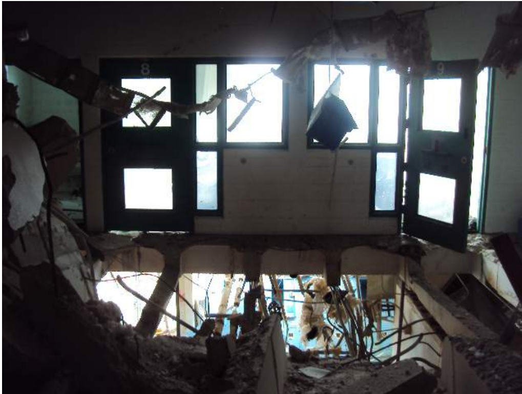
Photo 144: 1 st Floor –Room 1902 – Between column lines J.5 and L & 6.6 and 8 – Looking North– Collapsed concrete floor
