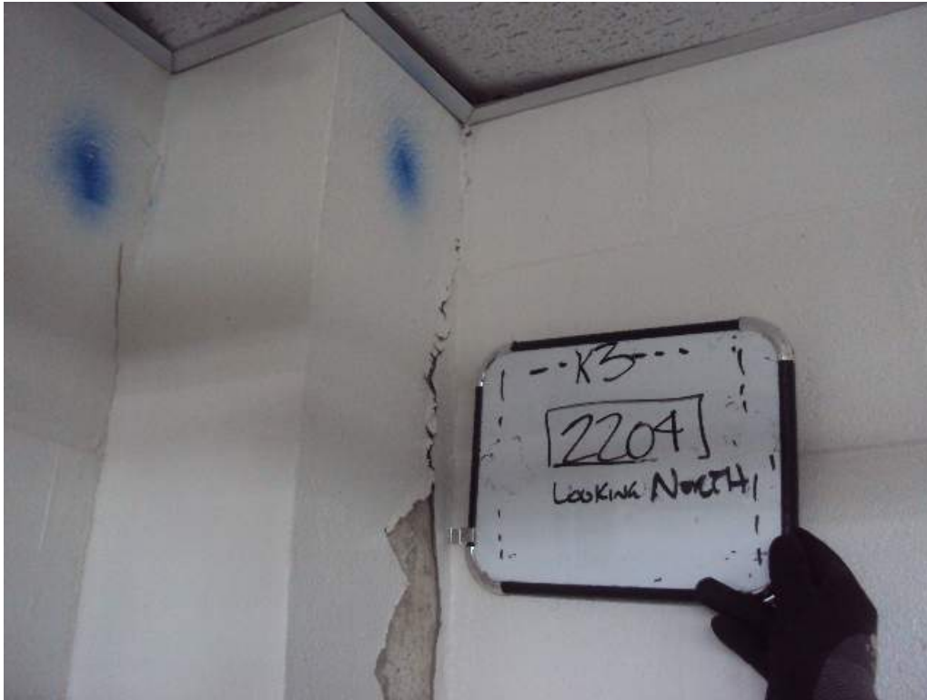
Photo 70: 2 nd Floor – Room 2204 – At col line 3K-Looking North –Vertical crack between concrete col and CMU wall
