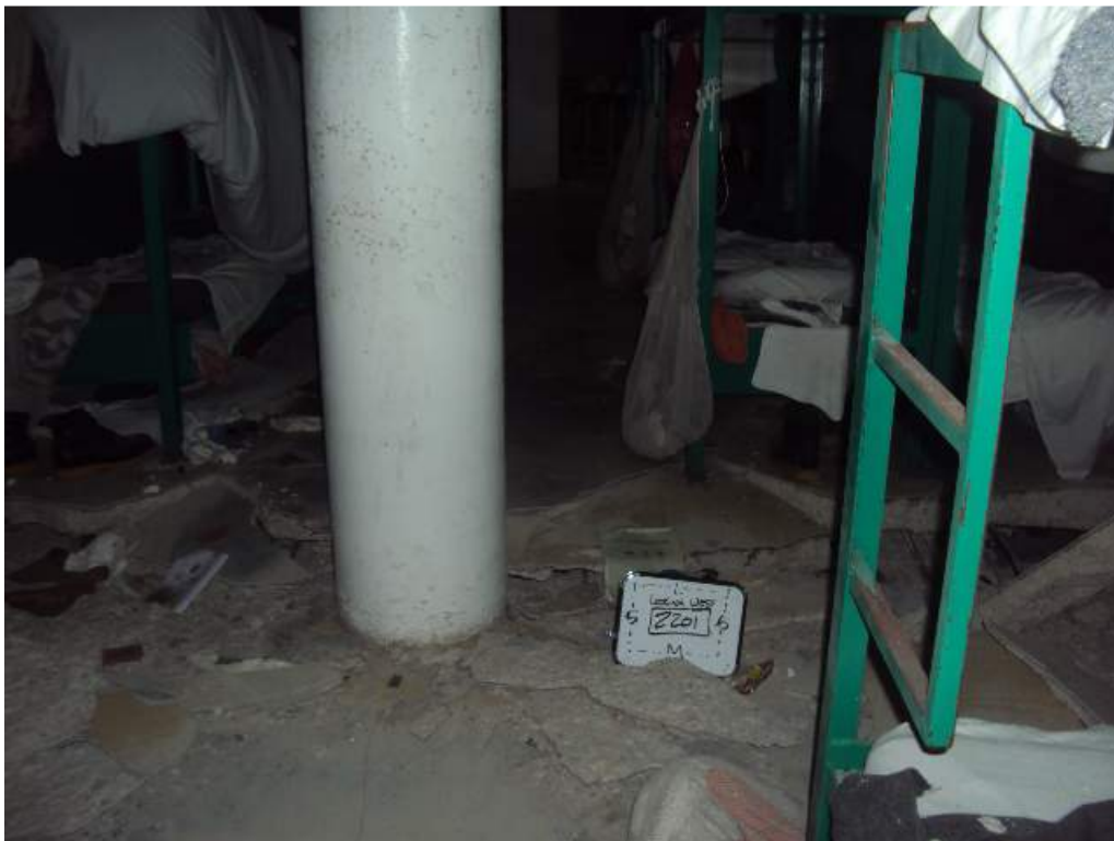
Photo 55: 2 nd Floor – Room 2201-East Dormitory –Between column lines 4 and 5 & L and M - Looking West - Buckled, collapsed and sheared floor slab
