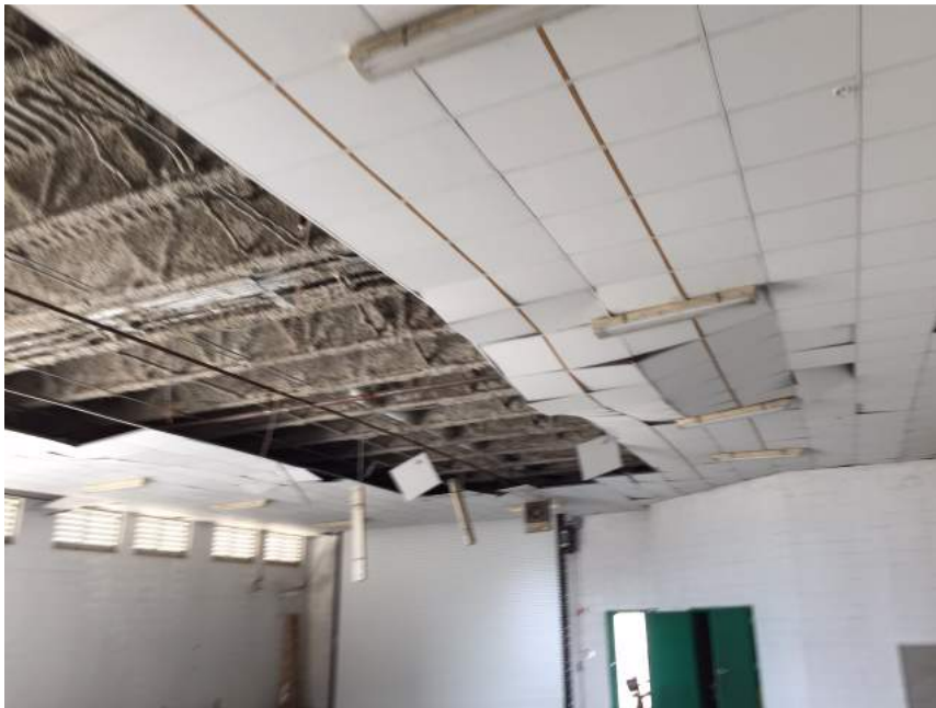
Vehicle gally port lighting fixture damage.
