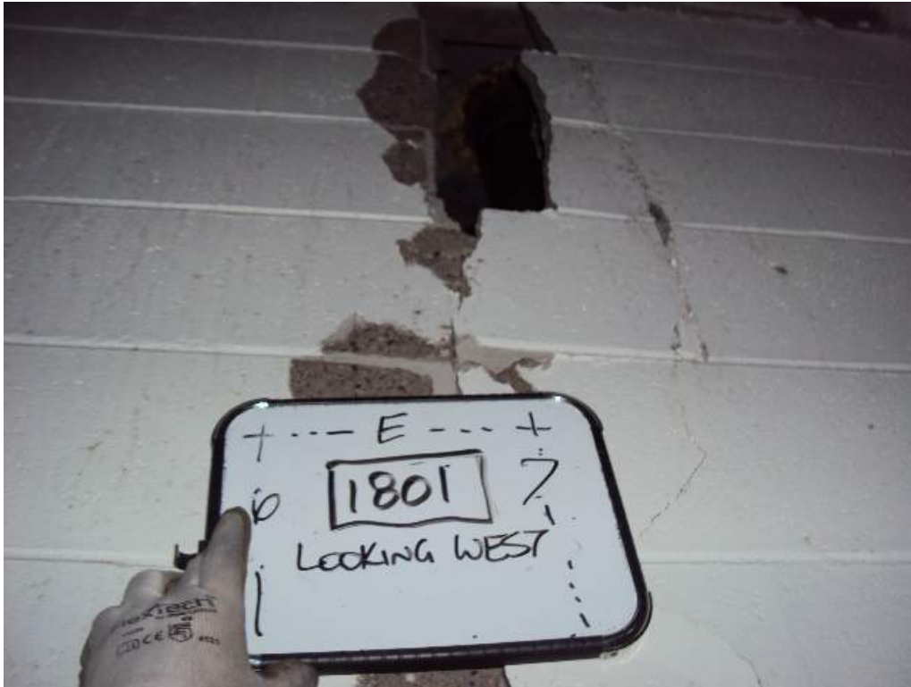
Photo 124: 1 st Floor – Room 1801– Along col line E between 6 and 7– Looking North– Cracked, sheared and partially collapsed CMU wall
