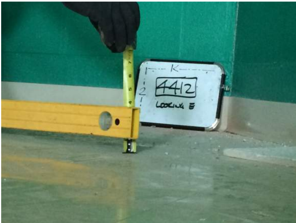
Photo 26: 4 TH Floor-Room 4412-Adjacent to col line 2 and behind col line K – Looking East – Settlement of the concrete floor
