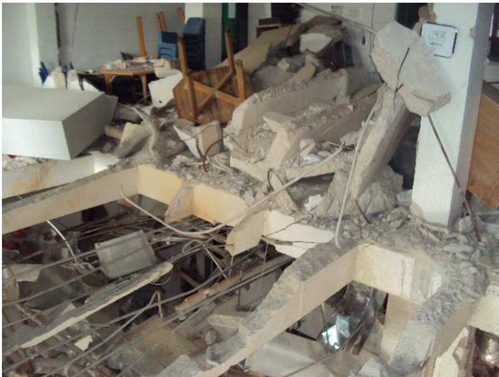
Photo 143: 1 st Floor –Room 1902 – Between column lines J.5 and L & 6.6 and 8 – Looking Southeast– Collapsed concrete floor
