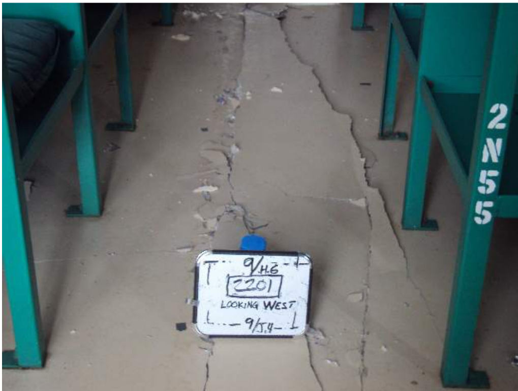
Photo 83: 2 nd Floor – Room 2201 North Dormitory – Along col line 9 between col lines H.6 and J.4 – Looking West –Buckled, Cracked and Shear floor slabs
