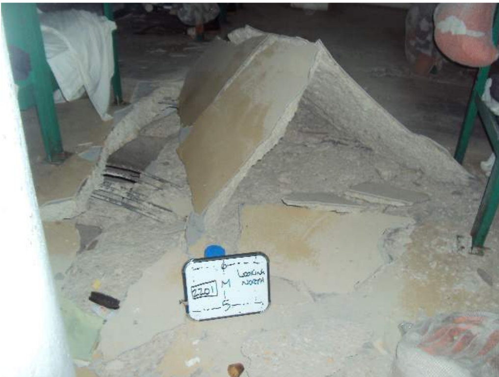
Photo 59: 2 nd Floor – Room 2201-East Dormitory –Along column line M between col lines 5 and 6 - Looking North - Buckled, collapsed and sheared floor slab
