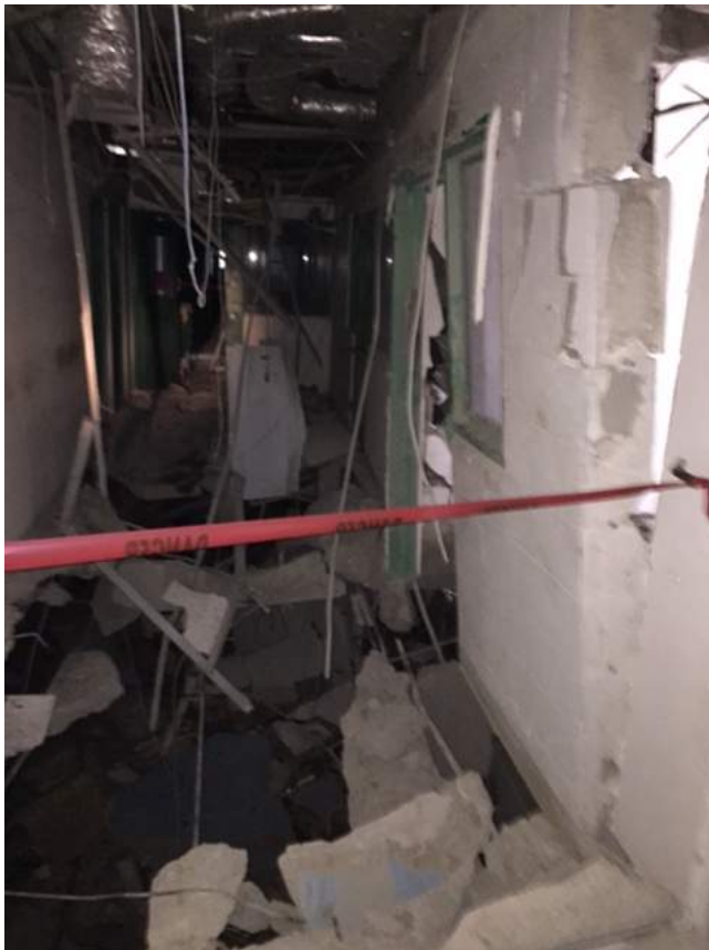
First floor corridor indicating branch circuit damage.
