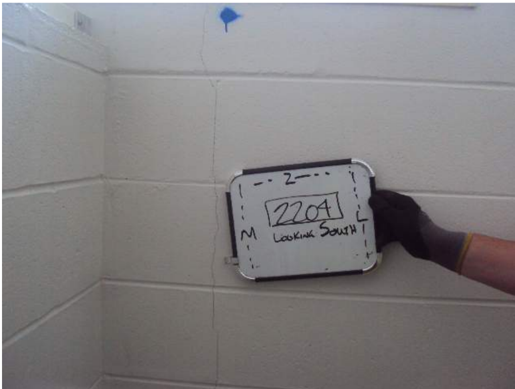
Photo 67: 2 nd Floor – Room 2204 – Along col line 2 between col lines L and M -looking South –Vertical crack in CMU wall
