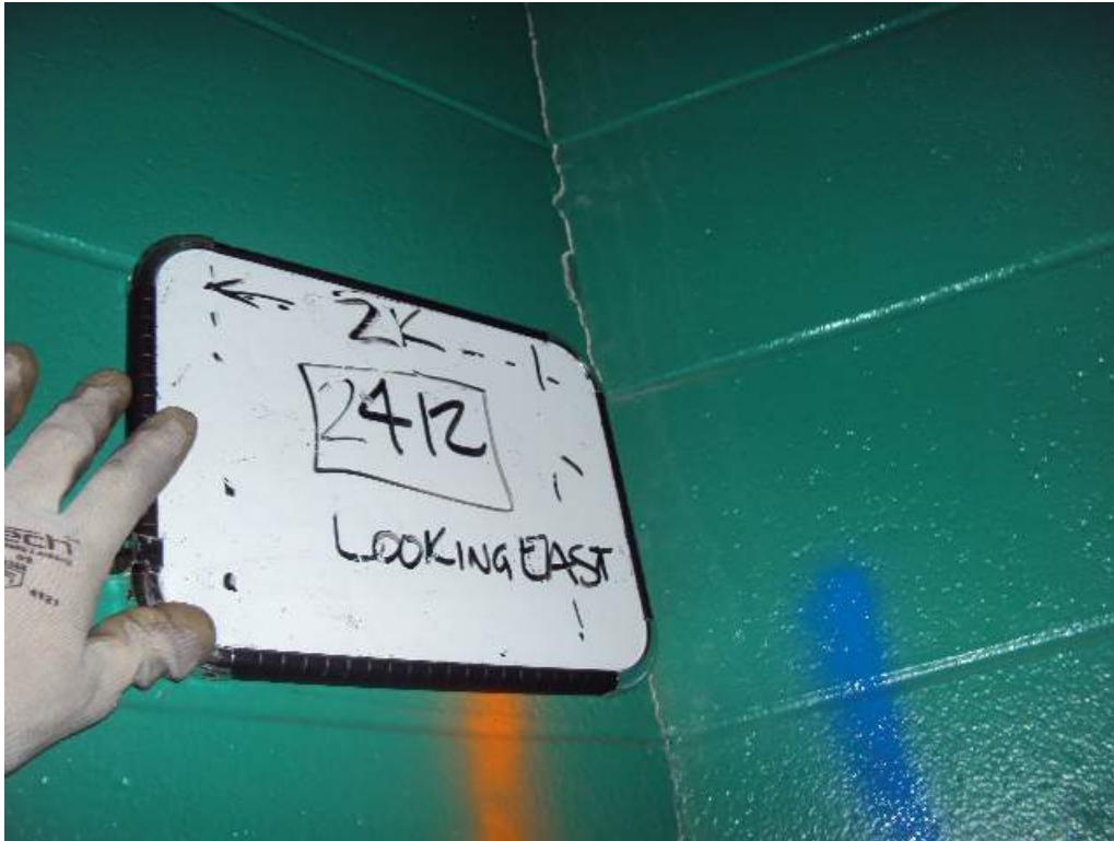
Photo 90: 2 nd Floor – Room 2412– Adjacent to col line 2K – Looking East –Vertical crack at CMU wall intersection
