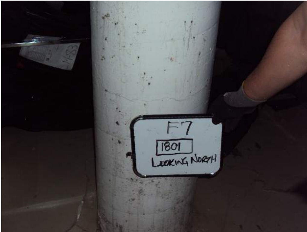
Photo 130: 1 st Floor –Room 1801 – At col line F7 – Looking North – Cracked columns
