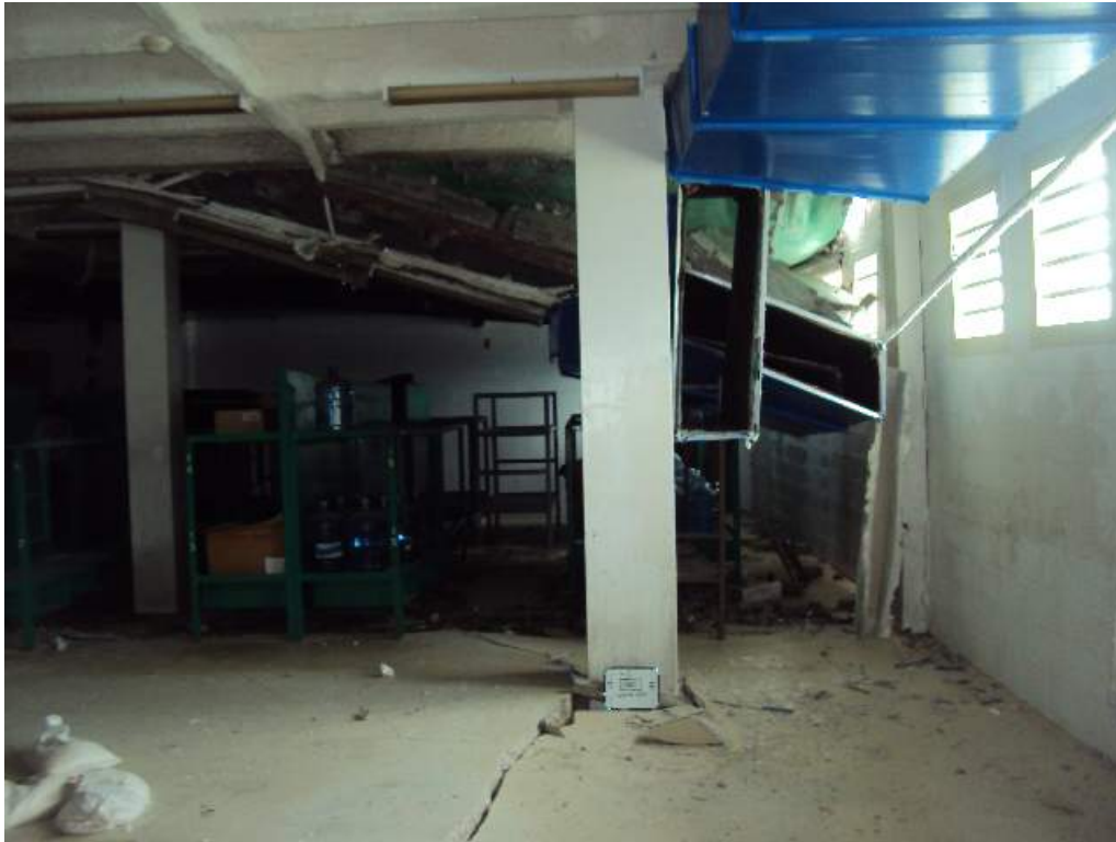
Photo 126: 1 st Floor –Room 1801 – Between col lines D and E & 7 and 8 – Looking West – Collapsed roof
