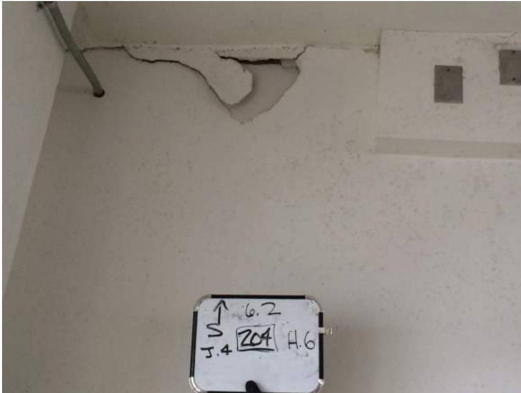
Photo 15: 4 th Floor – Room 204 – Along col Line 6.2 between H.6 & J.4-Looking South – Horizontal crack @ top of CMU wall
