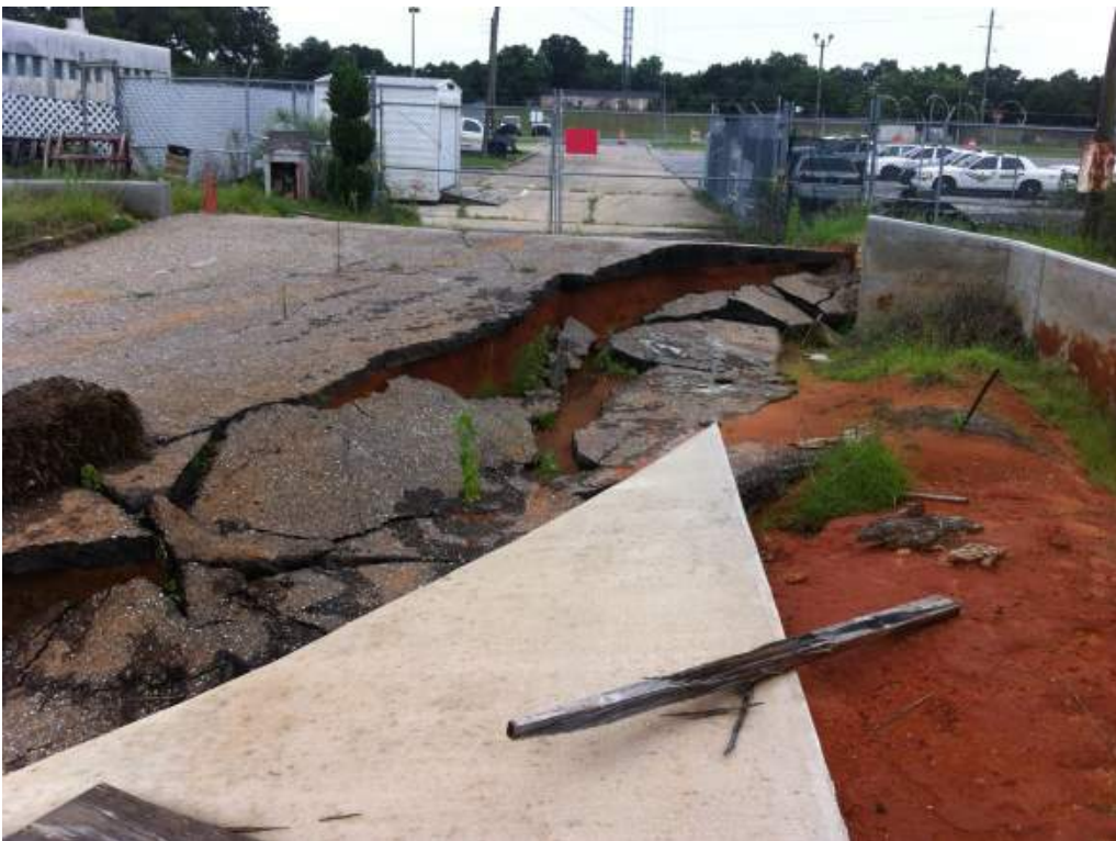
Photo 8: Northwest Access Road Erosion- Looking South
