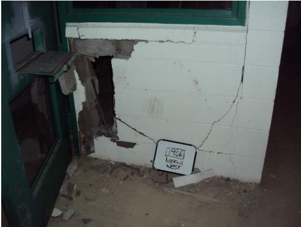
Photo 148: 1 st Floor –Room 1906 – Between col lines H.5 and J.5 & 7 and 7.3 – Looking West– Partially collapsed CMU walls
