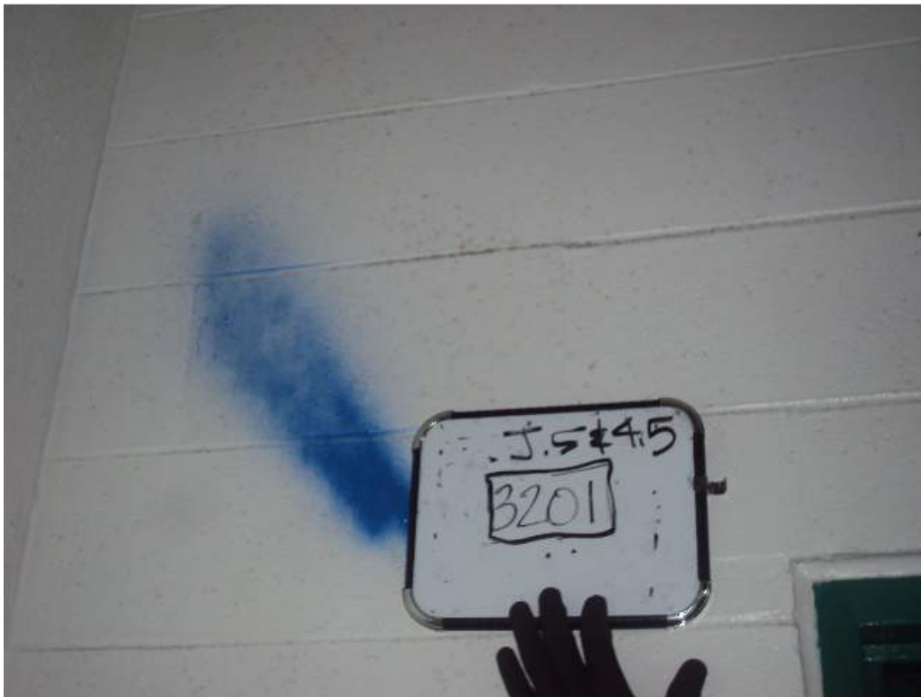
Photo 28: 3 rd Floor – Room 3201 – Adjacent to J.5 and 4.5 – Looking West - Diagonal cracking in CMU walls
