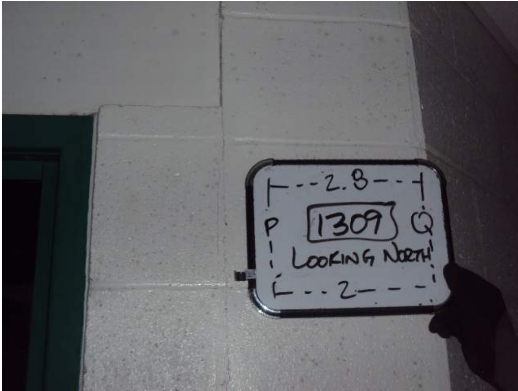
Photo 100: 1 st Floor – Room 1309– Between col lines 2 and 2.8 & P and Q – Looking North – Stair step crack and vertical crack in CMU wall
