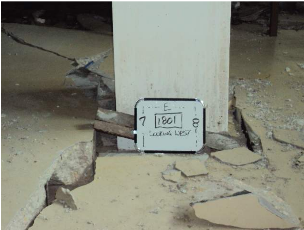
Photo 127: 1 st Floor –Room 1801 – Along col line E between 7 and 8 – Looking West – Collapsed roof
