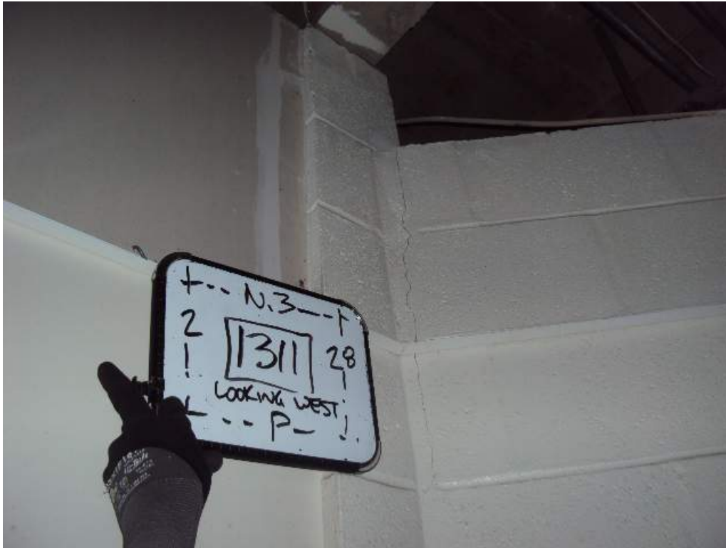
Photo 102: 1 st Floor – Room 1311– Between col lines N.3 and P & 2 and 2.8 – Looking West – Vertical crack in CMU column and wall
