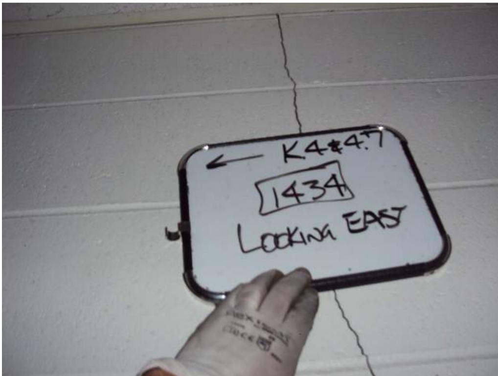
Photo 119: 1 st Floor – Room 1434– Adjacent to col line K4 and 4.7 – Looking East– Vertical crack in CMU wall
