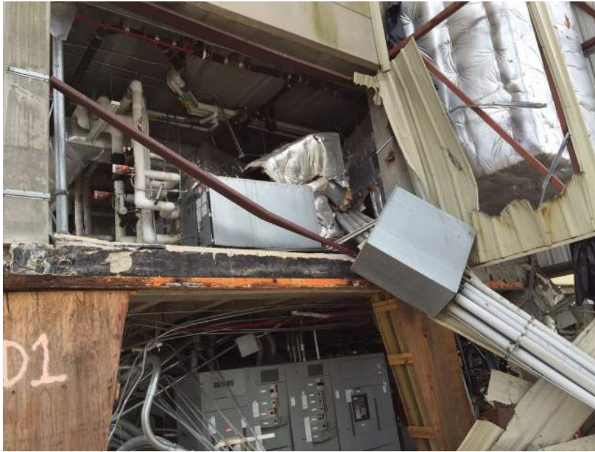
Basement/1 st floor view looking north. Electric boiler feeder and main distribution switchboard.
