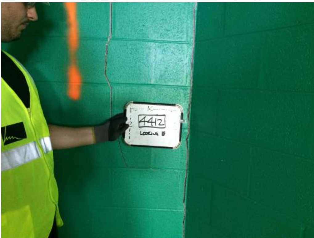
Photo 25: 4 TH Floor-Room 4412-Adjacent to col line 2 and behind col line K – Looking East – Vertical cracks in CMU wall
