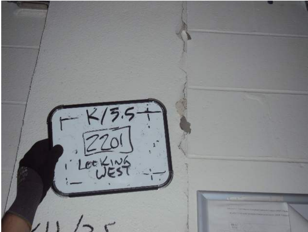
Photo 64: 2 nd Floor – Room 2201 – East Dormitory – At column line 3.5&K- Looking West-Vertical cracks between a concrete column and CMU wall
