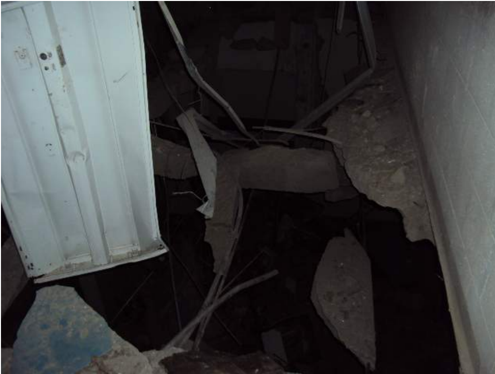
Photo 150: 1 st Floor –Room 1226 – Between col lines L and M & 5.5 and 6 – Looking West– Collapsed floor slabs
