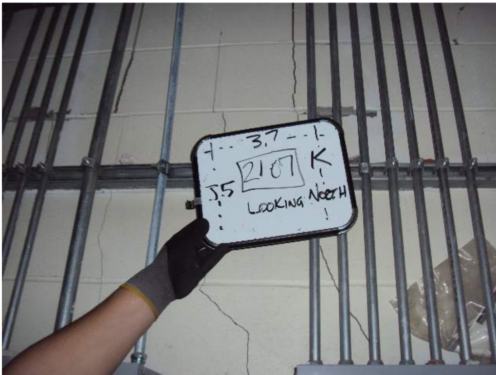
Photo 89: 2 nd Floor – Room 2107– Adjacent to col line 3.7 between col lines J.5 and K – Looking North – Collapsed elevator CMU wall
