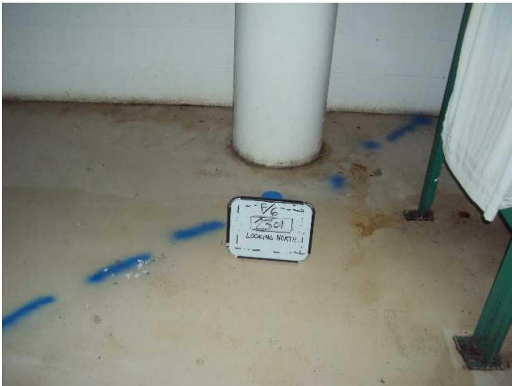
Photo 77: 2 nd Floor – Room 2301 – At col line F6-Looking North –Crack in the floor slab
