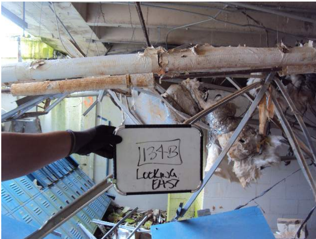
Photo 152: Basement –Room 134B– Between col lines K.2 and L & 7 and 8 – Looking East– Collapsed CMU walls
