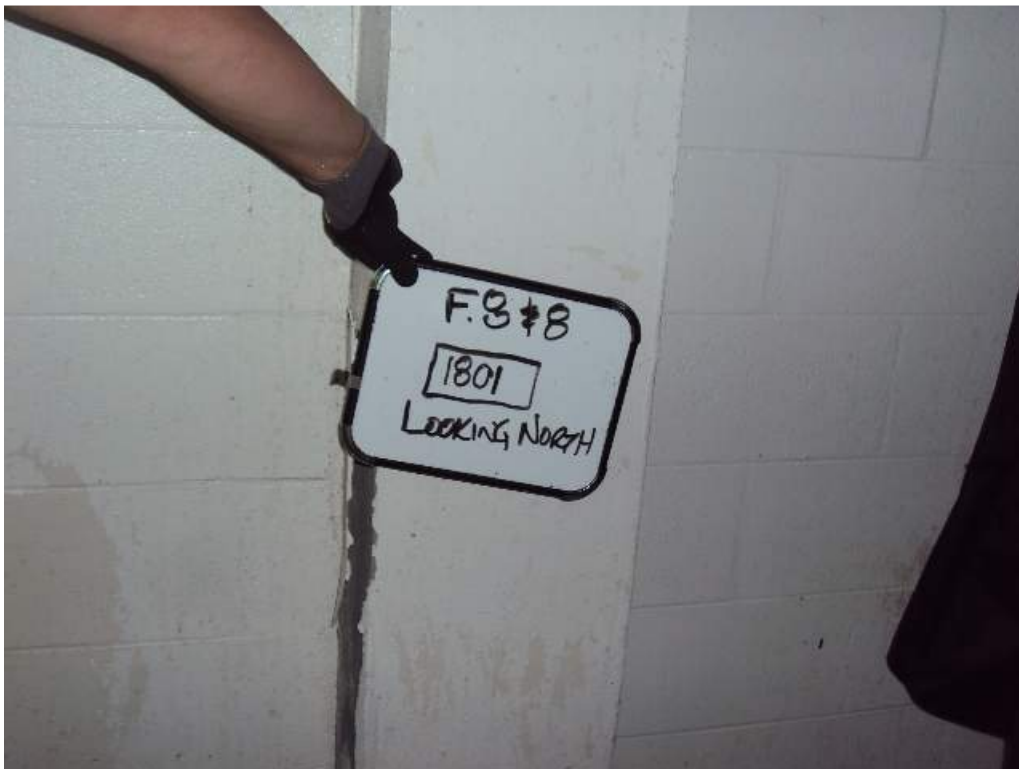
Photo 129: 1 st Floor –Room 1801 – At col line F.8 & 8 – Looking North – Vertical crack between concrete col and CMU wall
