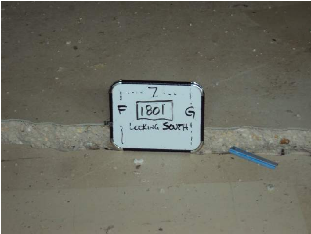
Photo 128: 1 st Floor –Room 1801 – Along col line 7 between F and G – Looking South – Sheared concrete slab
