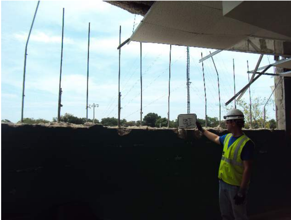
Photo 47: 3 rd Floor – Room 3412 – Col line 1.8 north of photo – Looking South – Missing portions of CMU wall with exposed reinforcement
