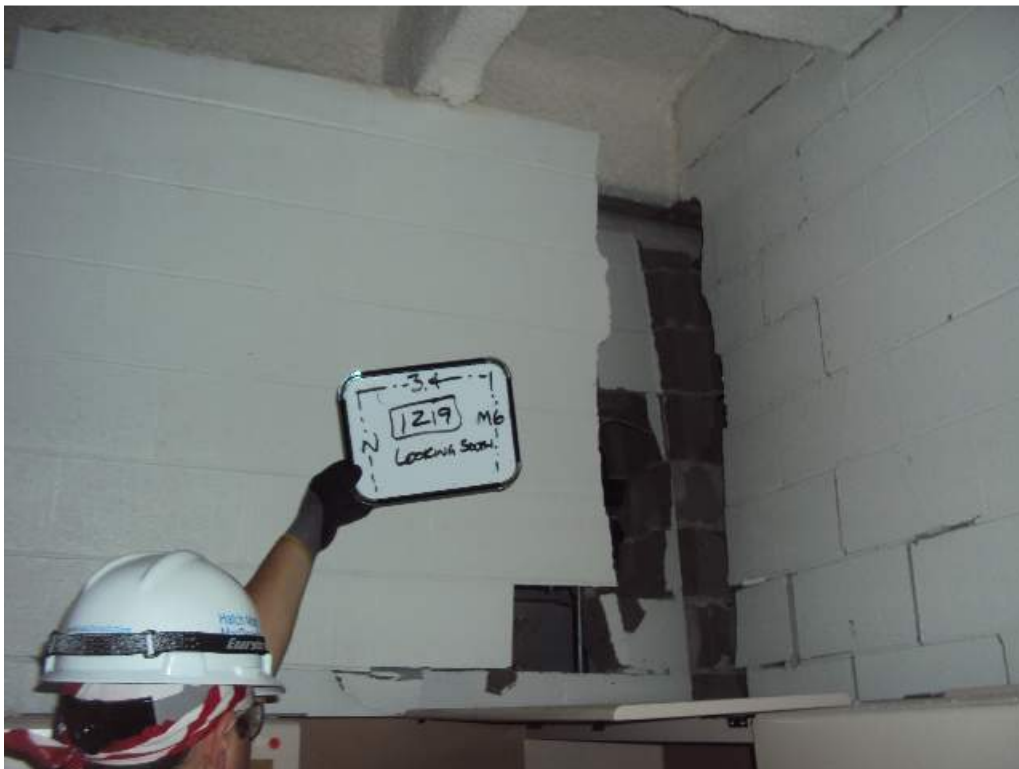
Photo 97: 1 st Floor – Room 1219– Along col line 3.4 between col lines M.6 and N– Looking South– Partially collapsed CMU wall
