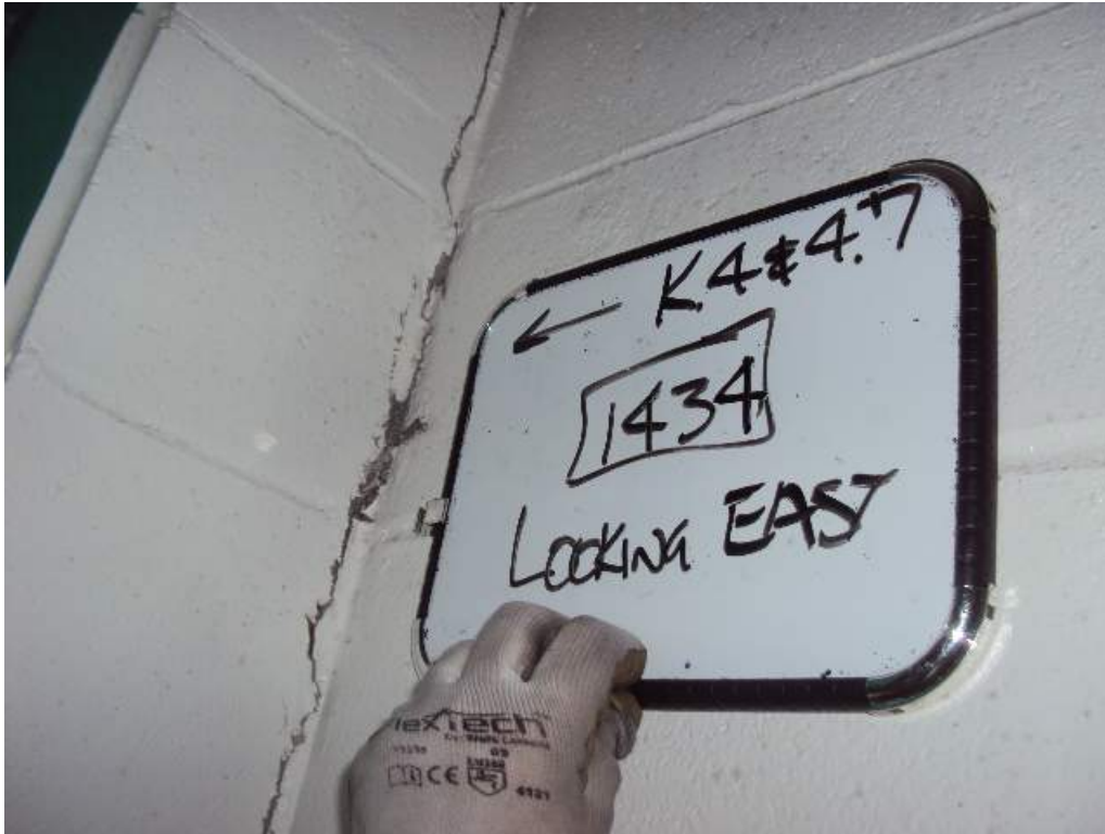
Photo 118: 1 st Floor – Room 1434– Adjacent to col line K4 and 4.7 – Looking East– Vertical crack at CMU wall corner
