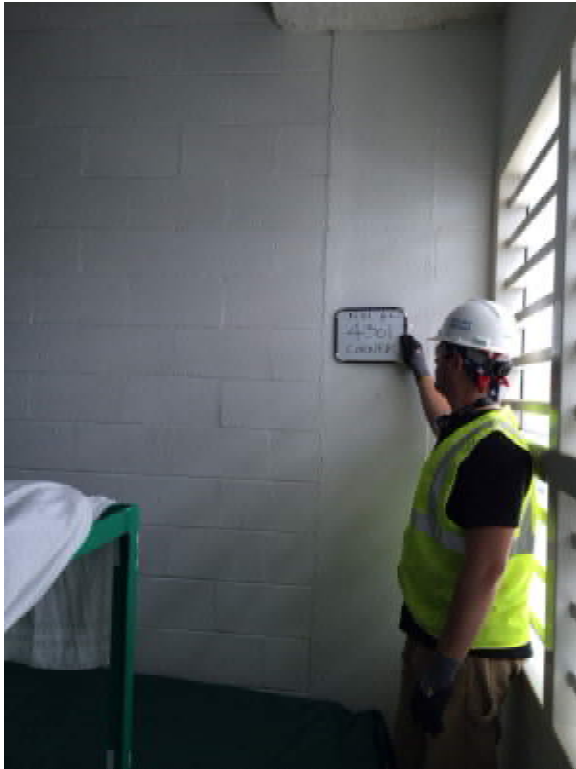
Photo 13: 4 th Floor – Room 4301 – Col line 6/E2 – Looking West - Vertical crack between the concrete column and CMU wall
