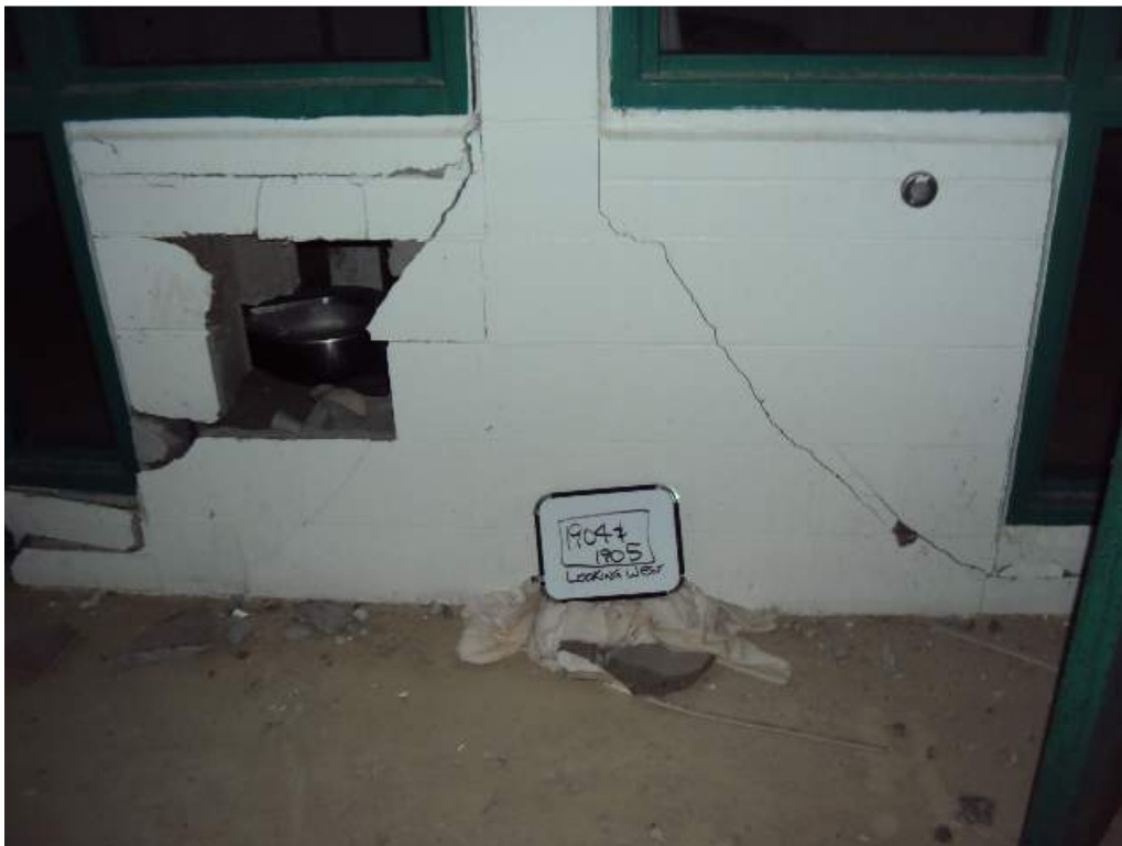
Photo 149: 1 st Floor –Room 1904 and 1905 – Between col lines H.5 and J.5 & 6 and 7 – Looking West– Partially collapsed CMU walls
