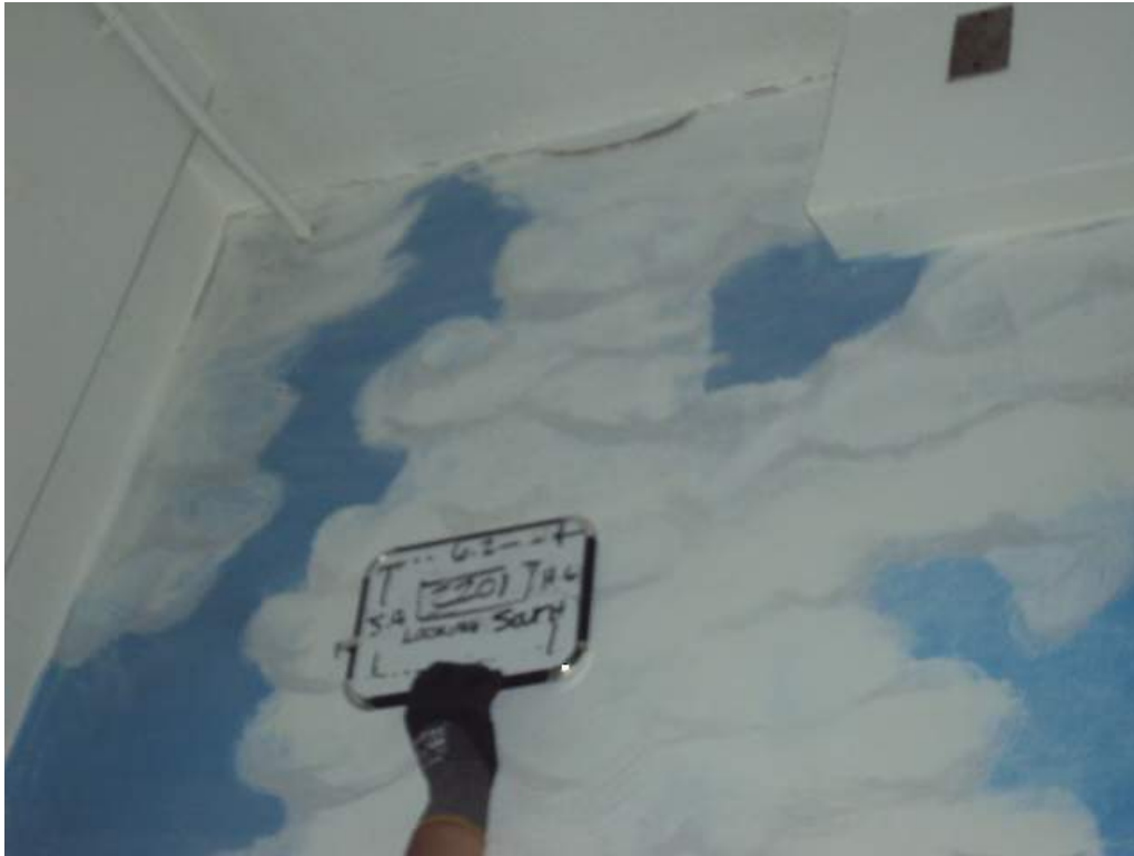
Photo 80: 2 nd Floor – Room 2201 North Dormitory – Along col line 6.2 between col lines J.4 and H.6 – Looking South –Horizontal crack @ top of CMU wall
