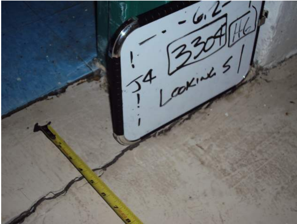
Photo 39: 3 rd Floor – Room 3304 – Along col line 6.2 between col lines H.6 and J.4 –Crack in floor slab
