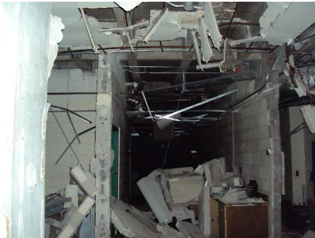
Photo 135: 1 st Floor –Room 1501– Between col lines F and G & 4.3 and 5.5 – Looking South – Collapsed CMU walls
