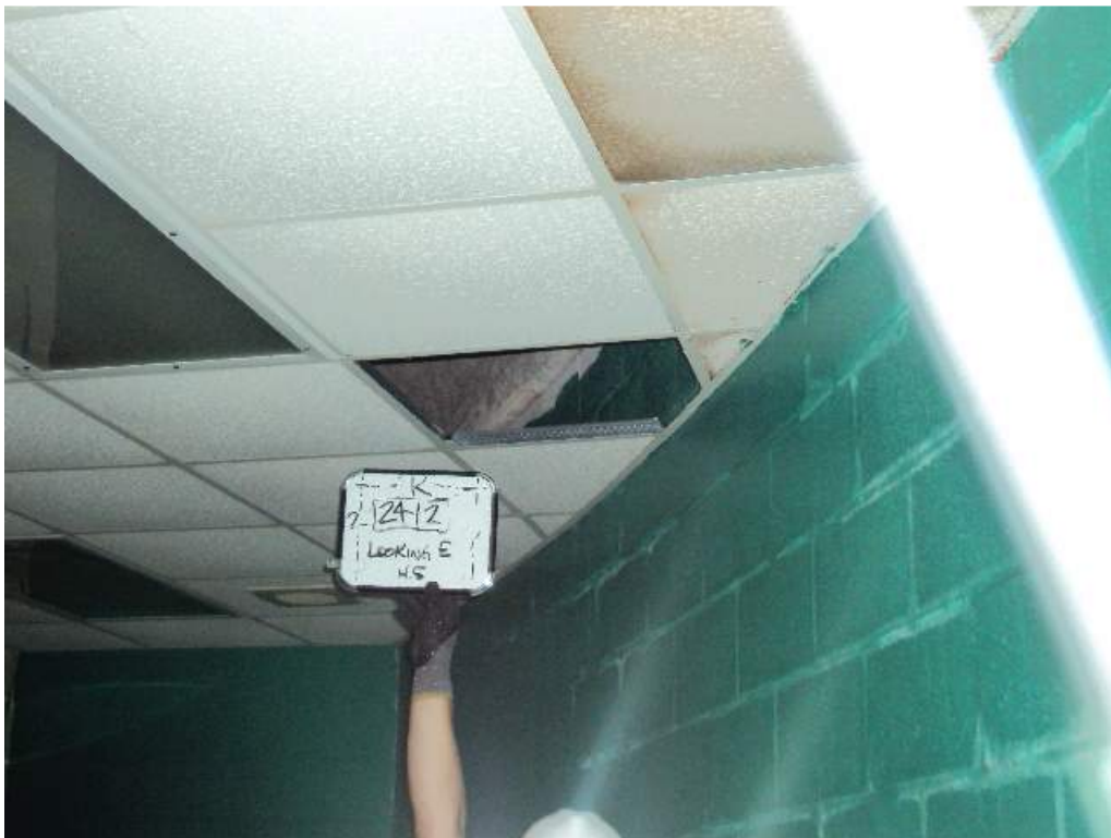
Photo 91: 2 nd Floor – Room 2412– Adjacent to col line 2K – Looking East –Collapsed portion of CMU wall below 3 rd floor slab
