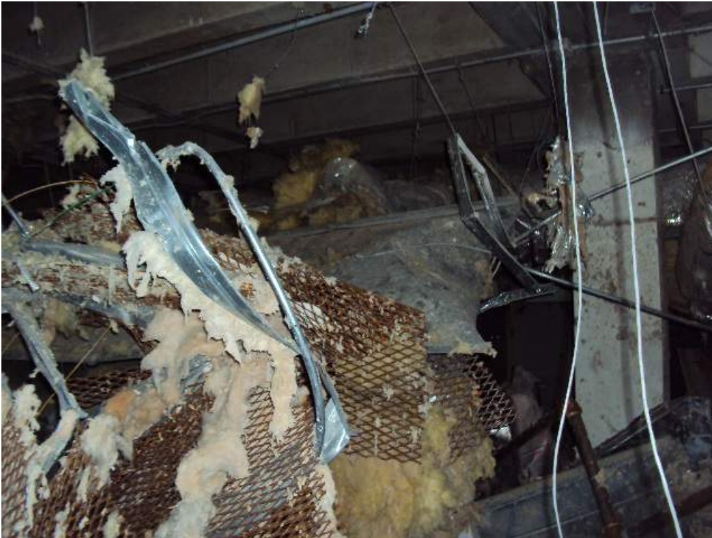
Photo 156: Basement –Room 102, 103, 104 & 127– Between col lines H.3 and K.2 & 3 and 4 – Looking South– Collapsed ceiling structure
