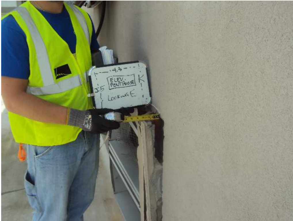
Photo 11: Elevator Penthouse –Along col line 4.3 between col lines J.5 and K – Looking East - Damaged exhaust vent and wall section at the elevator shaft
