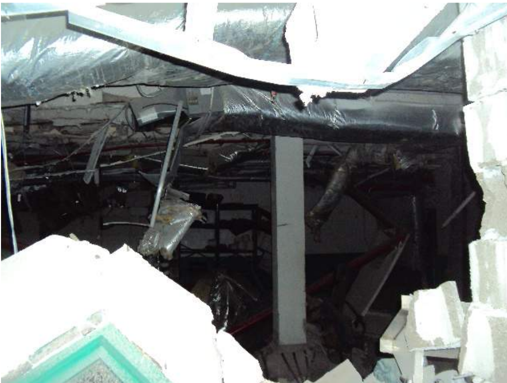
Photo 151: 1 st Floor –Room 1250 to 1252– Between col lines K.4 and M & 3 and 5.5 – Looking South– Collapsed CMU walls and floor slabs
