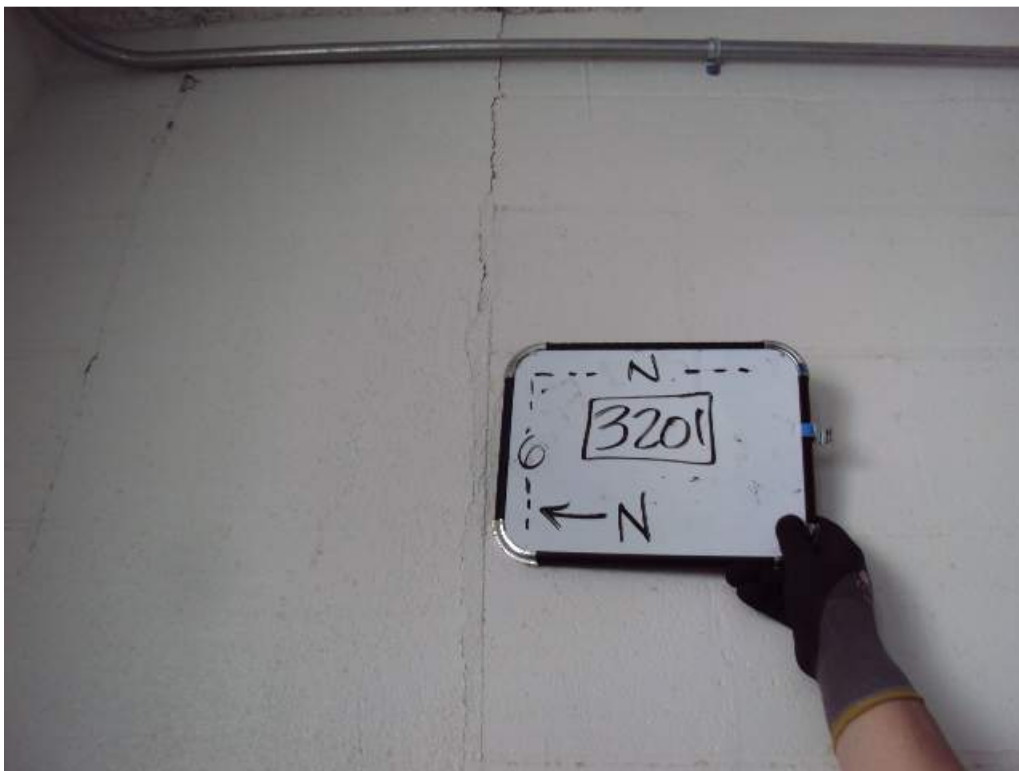
Photo 34: 3 rd Floor – Room 3201 – At col line N6 – Looking East – Vertical cracks between the concrete column and the CMU wall
