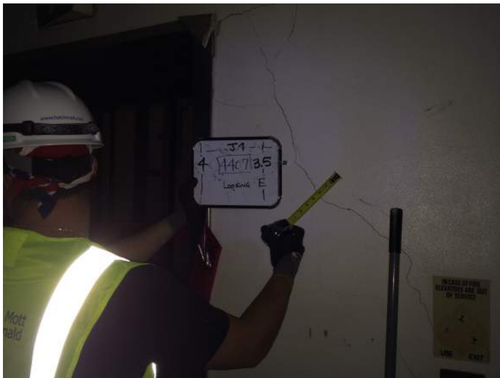
Photo 23: 4 th Floor- Room 4407-Along col line J.4 between 3.5 and 4 – Looking East – Map cracking in elevator CMU wall
