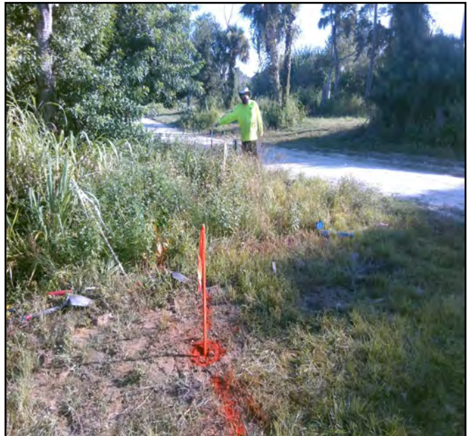
Tie 02 (From Test Hole): NORTH VALVE, WATER
