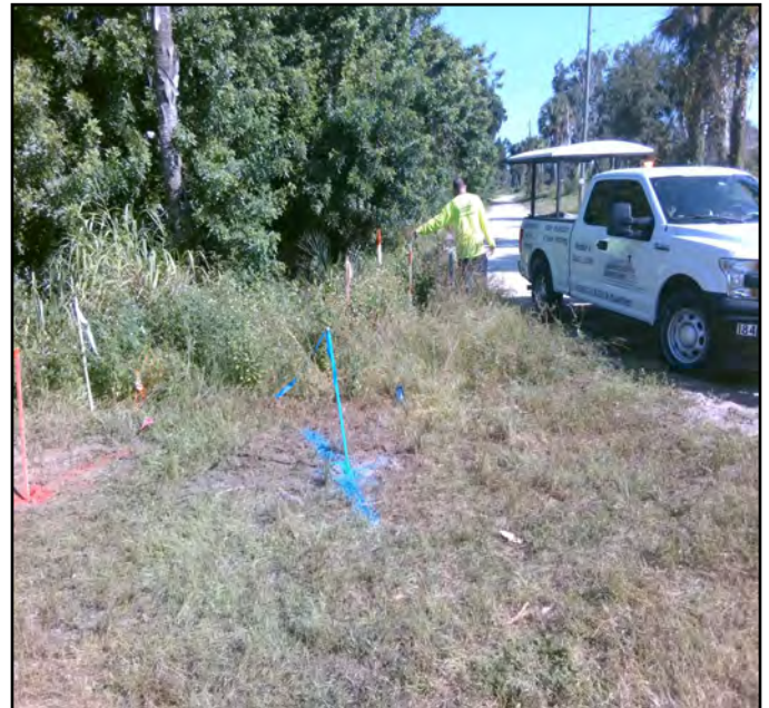
Tie 02 (From Test Hole): NORTH VALVE, WATER
