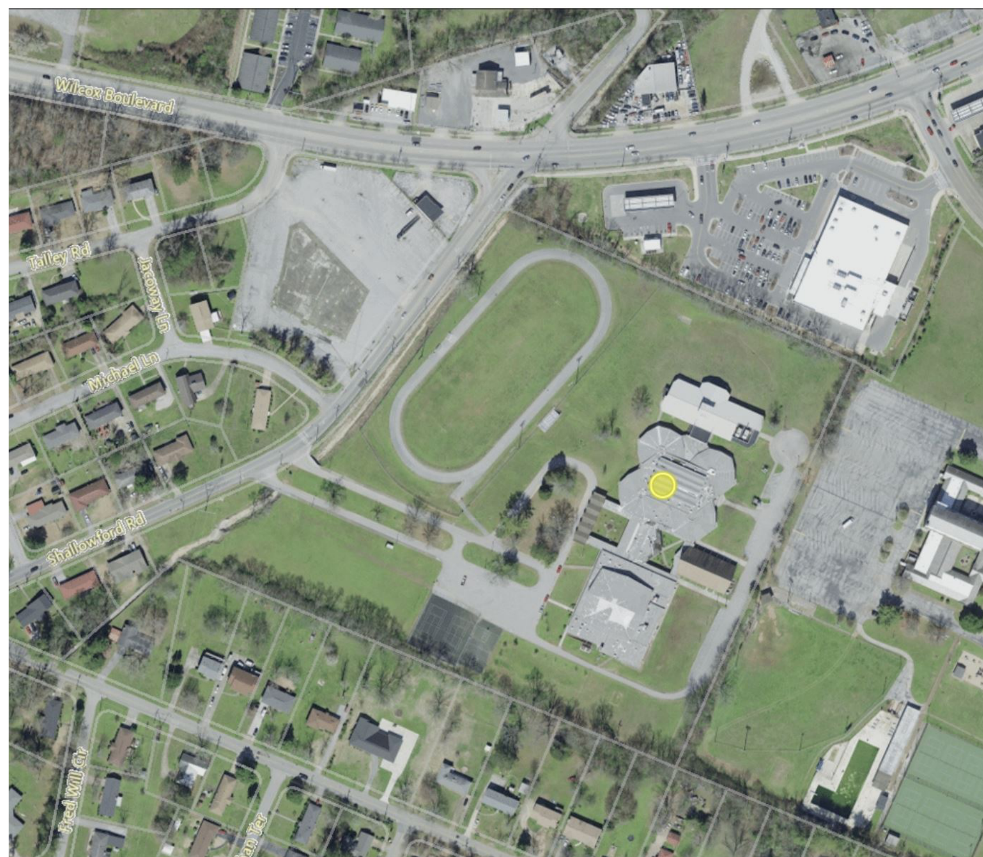
Aerial View of Dalewood Middle School
