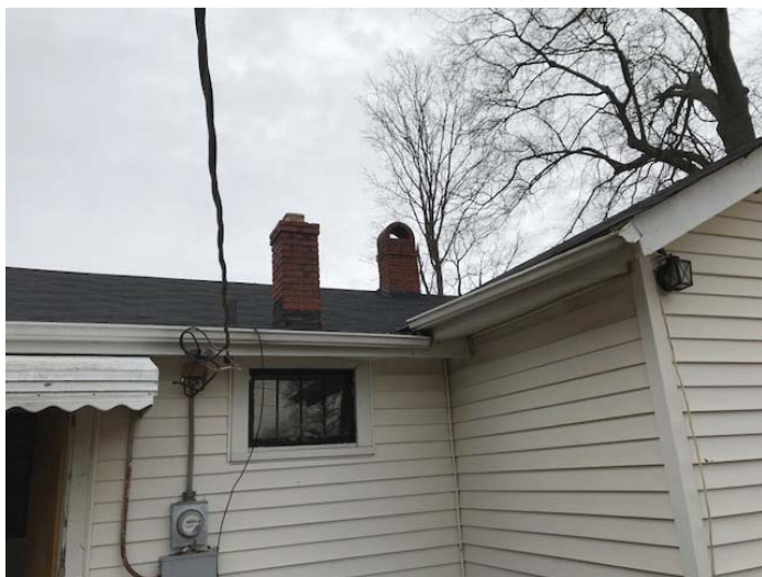
Photo 4 – 2 chimneys with mastic/tar – assumed positive & roof shingles & felt
