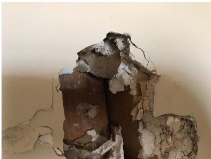
Photo 2 – Plaster with finish over unfinished drywall throughout
