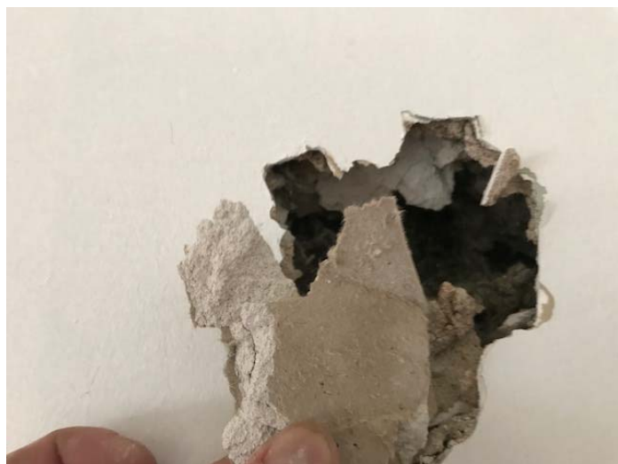
Photo 7 – Plaster with finish over unfinished drywall throughout
