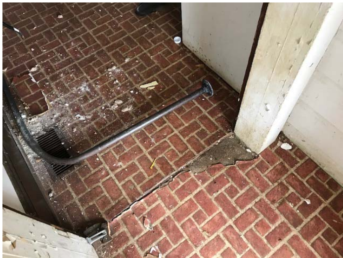
Photo 5 – Brick pattern roll vinyl & mastic over 9" x 9" tan floor tile & mastic in the kitchen
