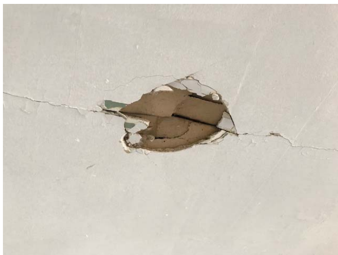
Photo 8 – Plaster with finish over unfinished drywall throughout
