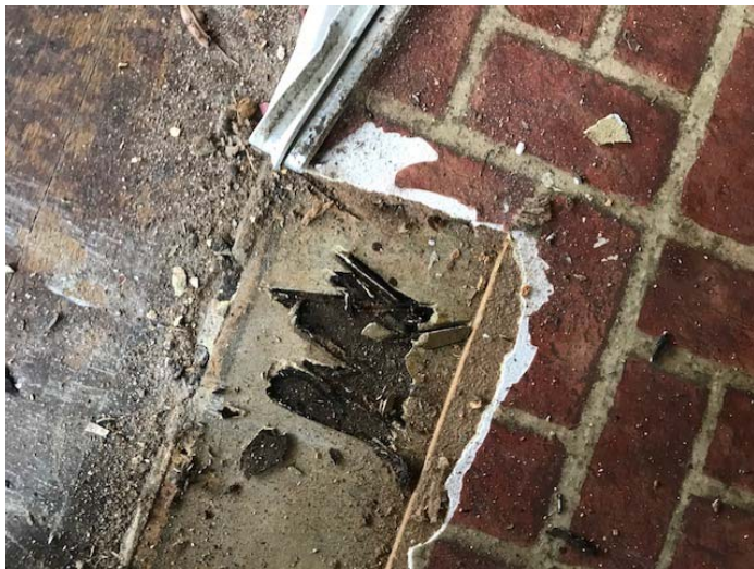
Photo 6 – Brick pattern roll vinyl & mastic over 9" x 9" tan floor tile & mastic in the kitchen
