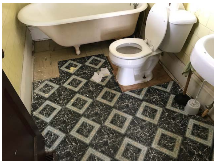
Photo 9 – Black/grey self-stick floor tile & mastic over 9" x 9" yellow floor tile & mastic & wooden pattern self-stick floor tile & mastic in the bathroom
