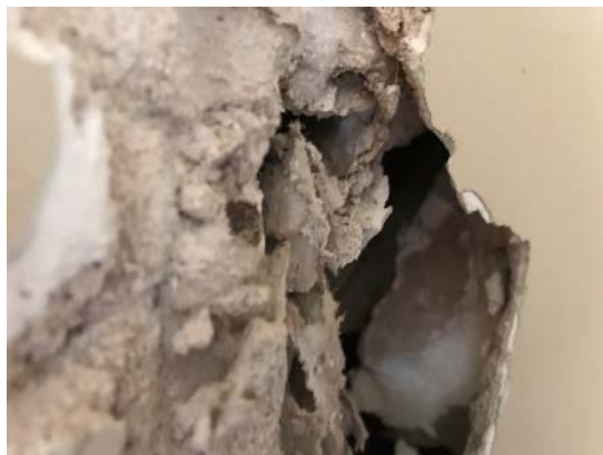
Photo 5 – Plaster over unfinished drywall walls.
