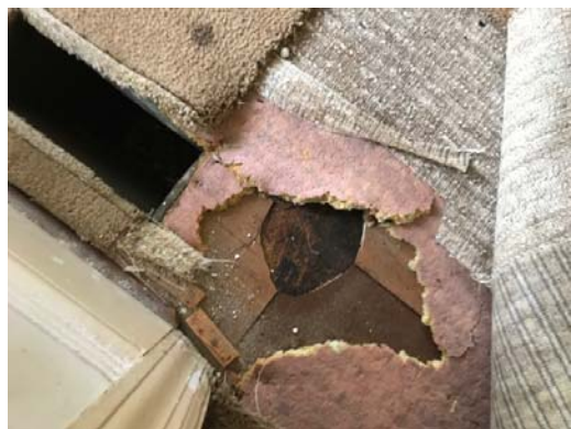
Photo 6 – Two colors of vinyl tile and mastic under carpet in living room.
