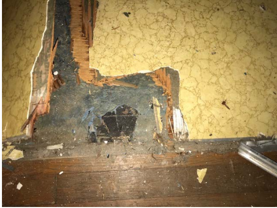
Photo 7 – Bathroom roll vinyl over wood over vinyl tile with mastic.
