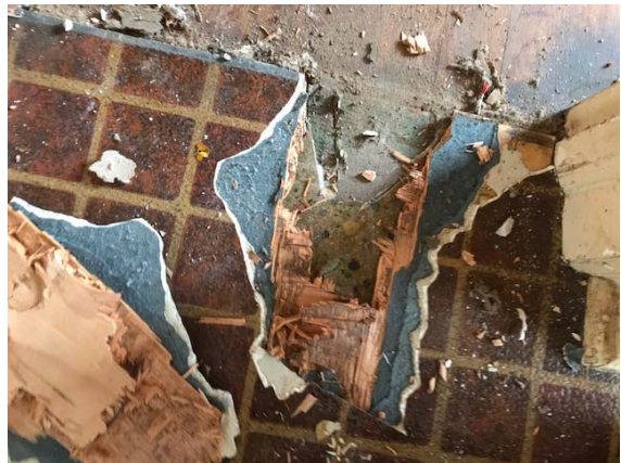
Photo 4 – Kitchen 3 layers of flooring, 3 rd under layer of wood.
