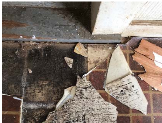
Photo 3 – Two layers of flooring and mastic in utility room.
