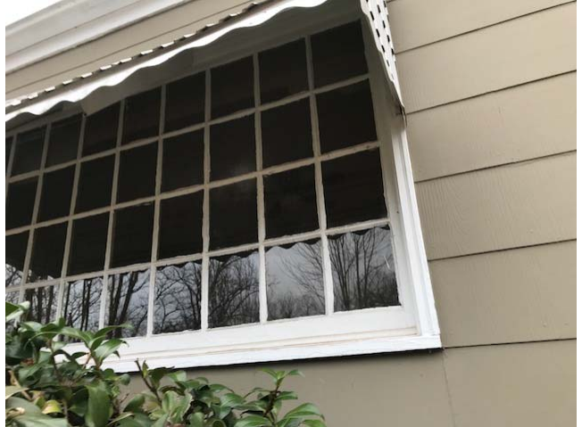
Photo 2 – Transite siding and window glaze.
