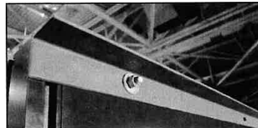
Figure 2 • Angle attached to slim cabinet mounting bolt.
