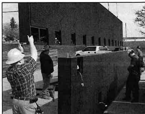
Figure 1 • Top section being placed onto lower section.
