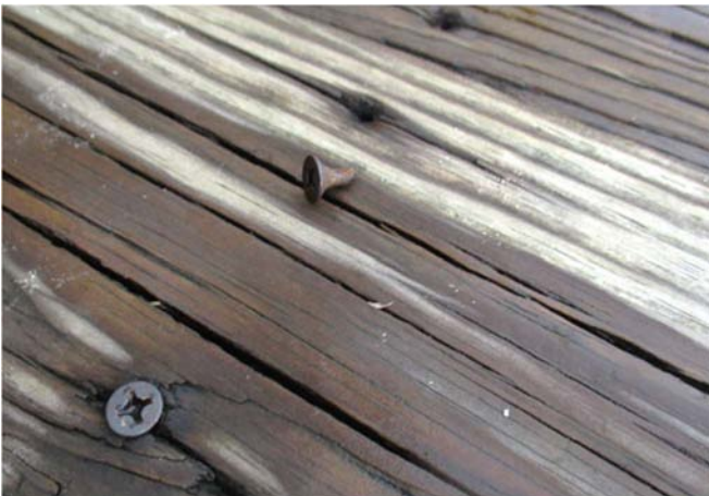
Photo 8 & 9 – Metal connector (screw) corrosion failure and wood deterioration of deck boards
