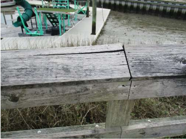
Photo 46 – Typical Cap rail damage in Phase 3B
