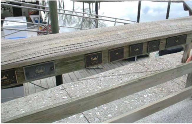
Photos 26 & 27 – Typical top cap of replaced guardrail with material defects (knots, splitting/checking)
