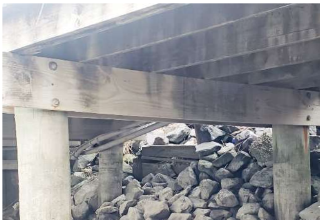
Photo 52 - Piles, pile caps and joists at Phase 3C
