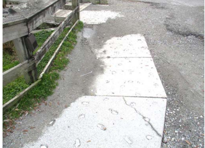
Photo 49 – Cracked concrete and trapped sediment
