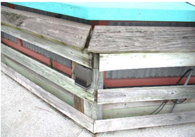
Photos 30 & 31 – Inside guardrail joint separation at corners showing damaged ends and connectors
