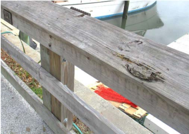
Photo 14 – Top rail deterioration due to knots
