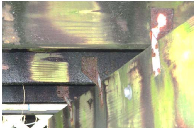
Photo 10 & 11 – Metal connector (screw) corrosion failure and wood deterioration of deck boards
