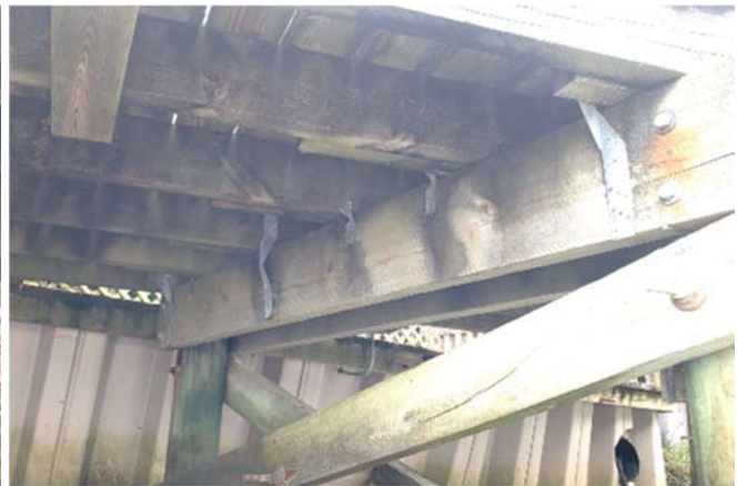
Photos 36 & 37 – Phase 2 framing of piles, pile caps, joists and metal connectors
