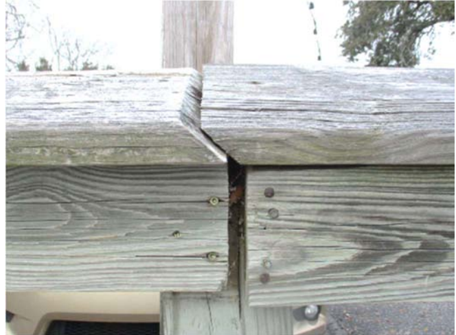
Photo 17 – Joint separation at post from shrinkage
