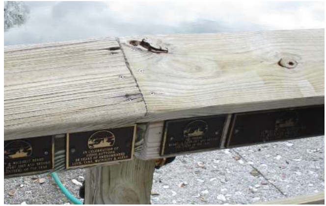
Photos 26 & 27 – Typical top cap of replaced guardrail with material defects (knots, splitting/checking)
