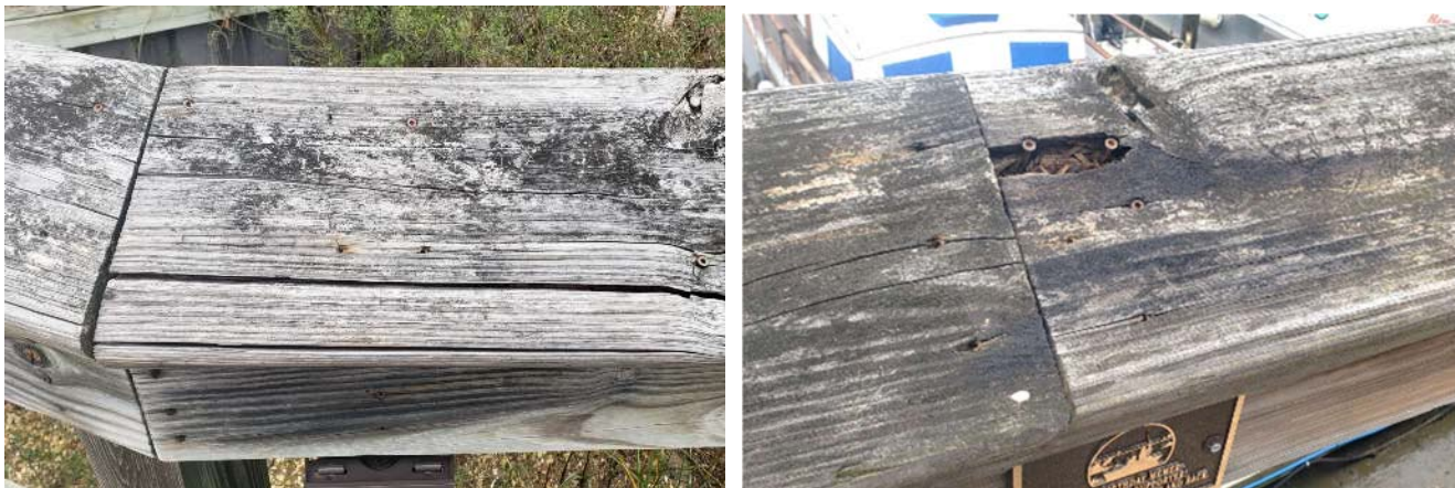
Photos 38 & 39 – Guardrail damage included missing, split and broken boards due to age and moisture
