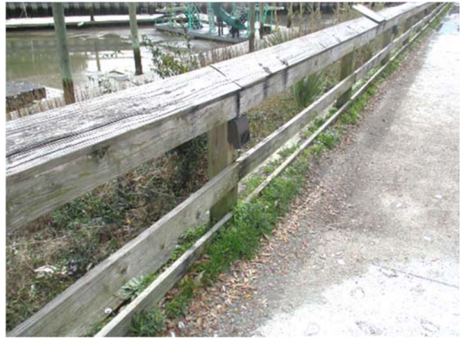
Photo 47 – Bottom rail mounted too close to ground
