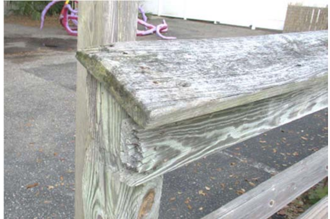
Photo 13 – Inside Guardrail cap deterioration
