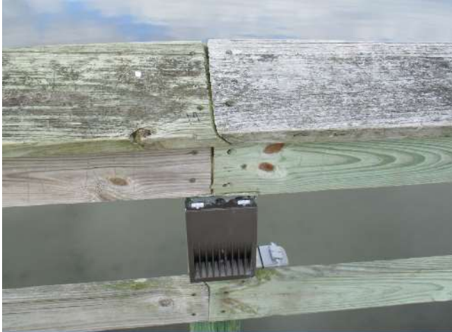
Photos 62 & 63 – Typical wood railing deterioration observed in isolated areas of Phase 4A
