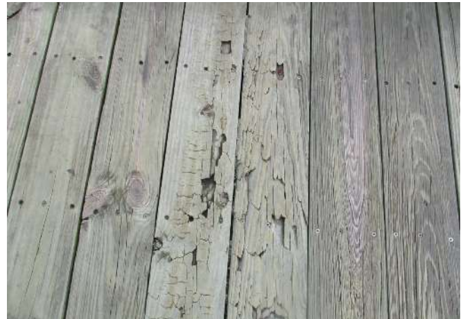
Photos 60 & 61 – Typical wood decking deterioration observed over large portions of Phase 4A
