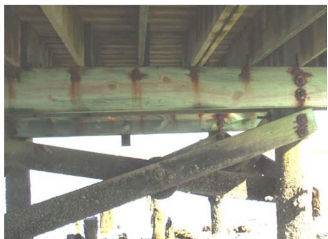
Photo 64 & 65 – Damaged metal connectors and galvanized bolts on Phase 4A to be replaced
