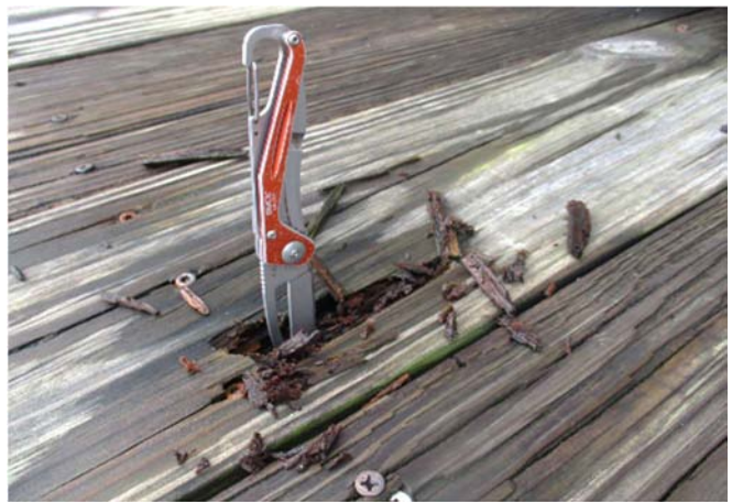
Photo 8 & 9 – Metal connector (screw) corrosion failure and wood deterioration of deck boards
