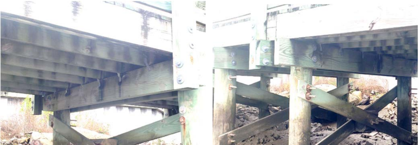
Photo 42 & 43 - Typical pile, pile cap, and joist framing below Ph 3A and connection at Ph 2 boardwalk
