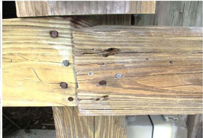
Photo 22 & 23 - Typical deck board and rail damage at ends and corroded/replaced connectors
