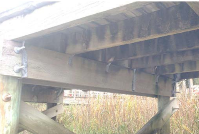
Photos 36 & 37 – Phase 2 framing of piles, pile caps, joists and metal connectors
