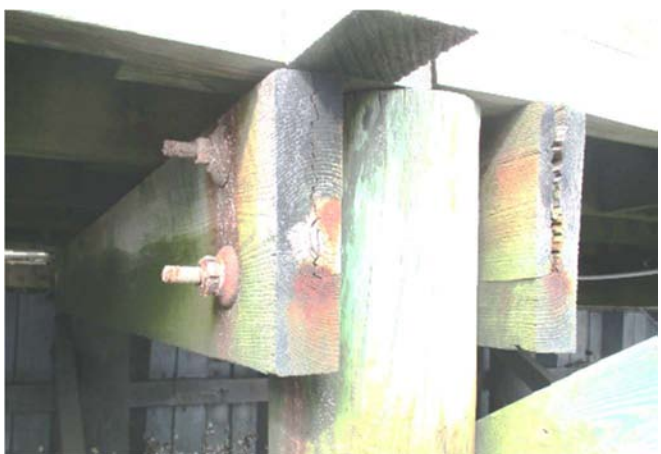
Photos 20 & 21 – Typical framing of WBOW in Phase 1D showing pile caps, joists and bolts
