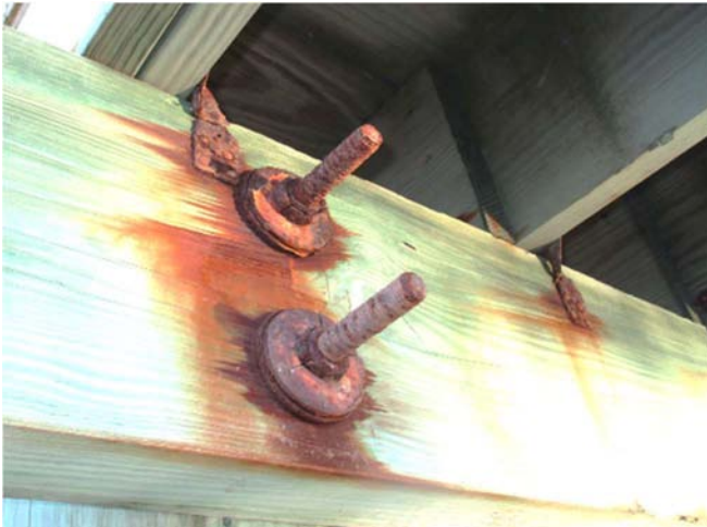
Photo 64 & 65 – Damaged metal connectors and galvanized bolts on Phase 4A to be replaced
