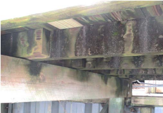
Photos 20 & 21 – Typical framing of WBOW in Phase 1D showing pile caps, joists and bolts
