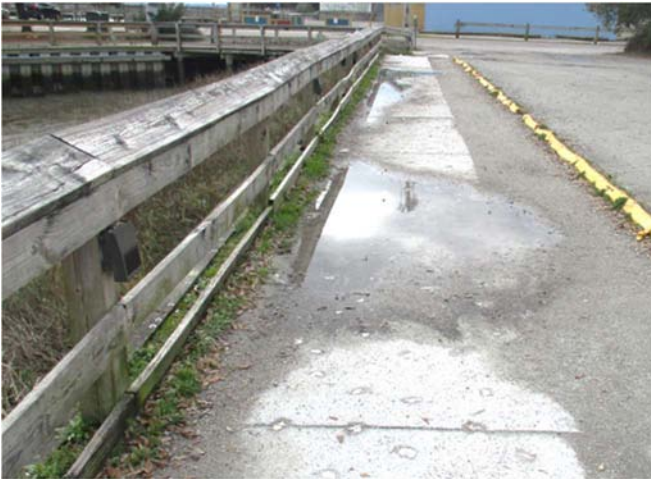
Photo 48 – Standing water due to blockage at rail
