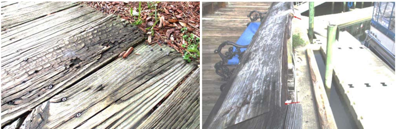
Photo 4 & 5 – Deteriorated wood decking and guardrails in Phase 1A due to age of materials
