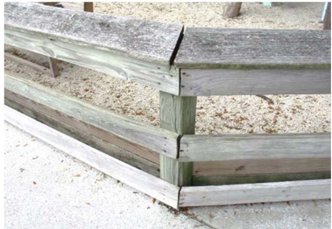
Photos 30 & 31 – Inside guardrail joint separation at corners showing damaged ends and connectors
