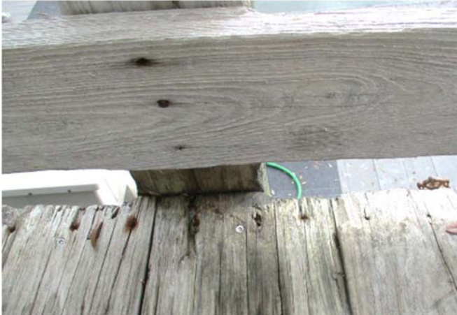
Photo 22 & 23 - Typical deck board and rail damage at ends and corroded/replaced connectors
