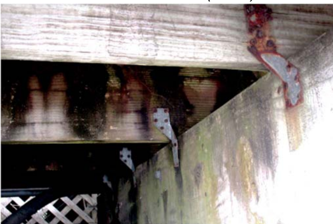
Photo 10 & 11 – Metal connector (screw) corrosion failure and wood deterioration of deck boards
