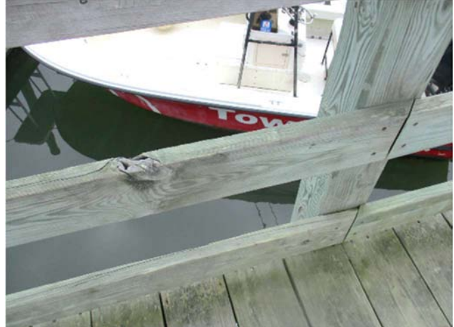
Photos 62 & 63 – Typical wood railing deterioration observed in isolated areas of Phase 4A
