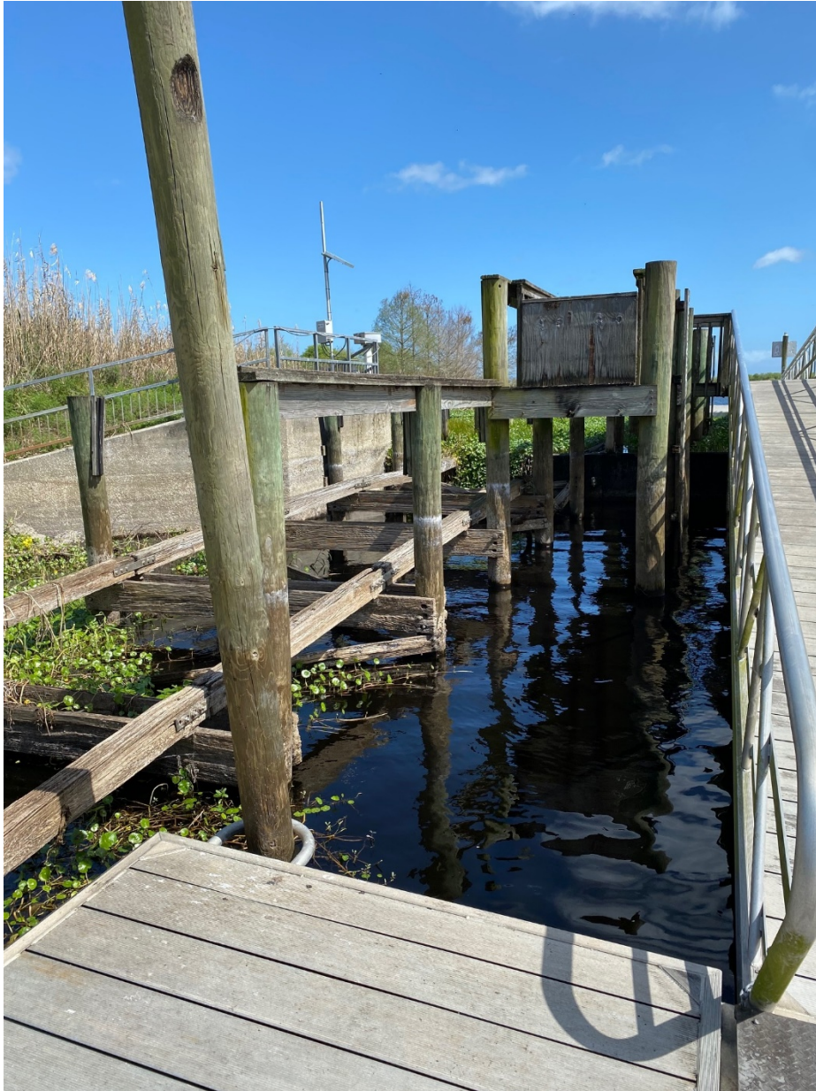
Small Boat Ramp/Operating Platform Looking South
