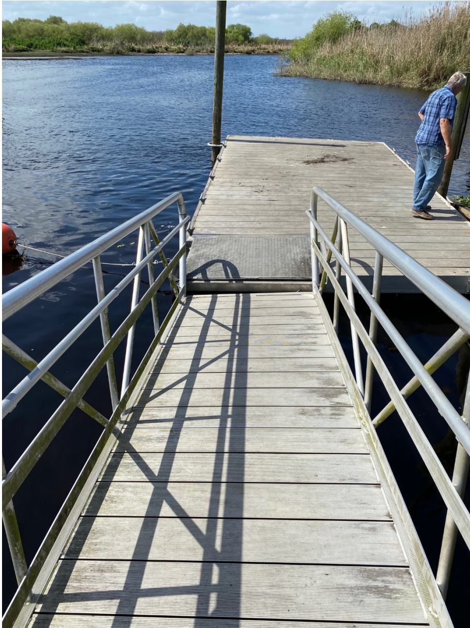
Downstream Gangway/Floating Dock: Platform to be extended, treadplate to be reconnected an extended
