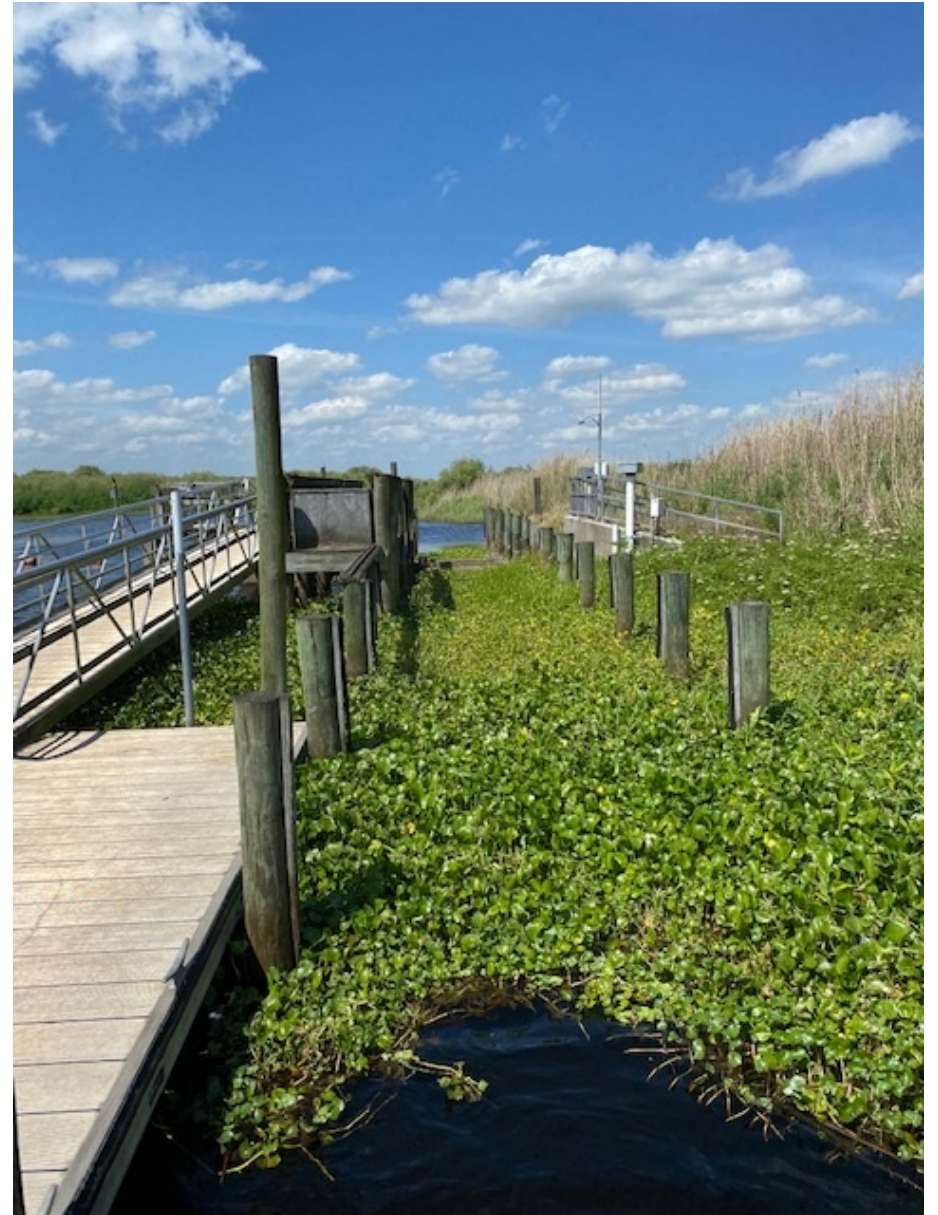
Small Boat Ramp/Operating Platform Looking North
