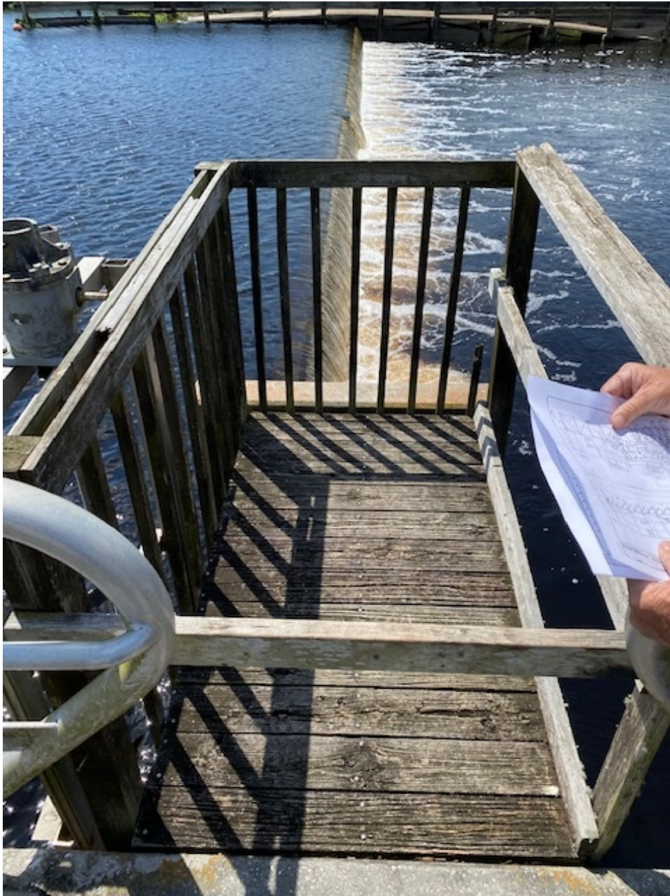
East Observation Deck to be removed, new walkway to be installed
