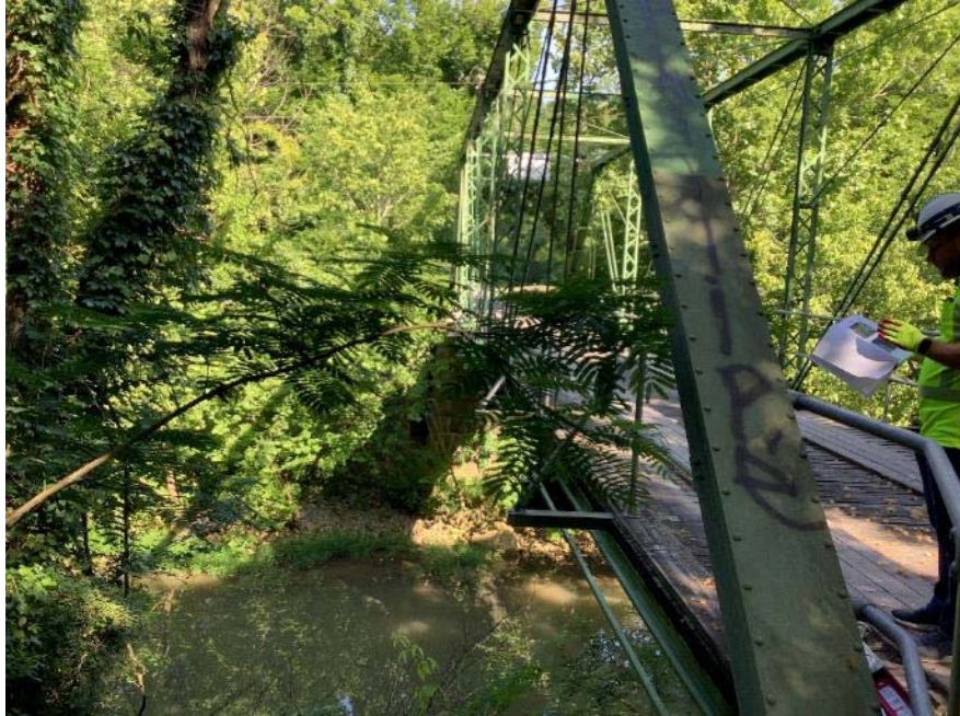
LEFT SIDE VIEW OF BRIDGE
