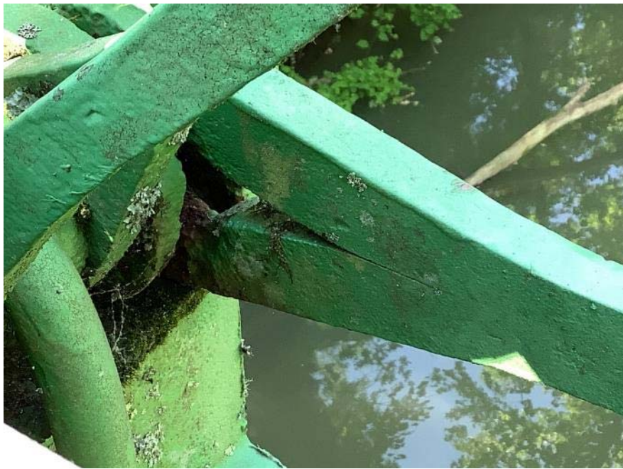
L3-L4 AT L3 CONNECTION LEFT SIDE
