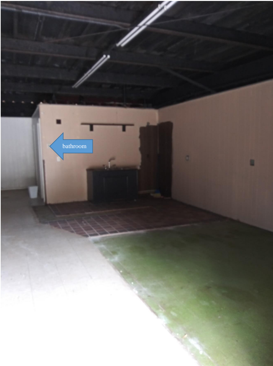
Northeast corner of building has 2 bathroom rough in
