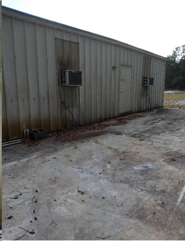
West side of building from a northwest location
