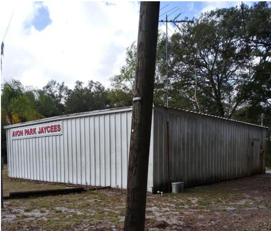
View from north east corner near power pole.
