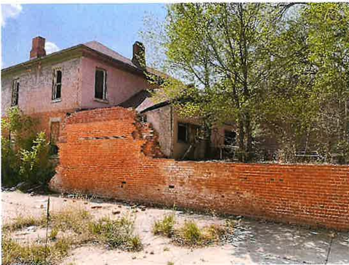
Structure 1 – North & West Elevations
