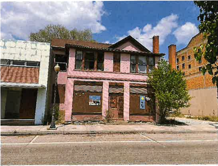
View of Structure 1 From Second Street; East Elevation
