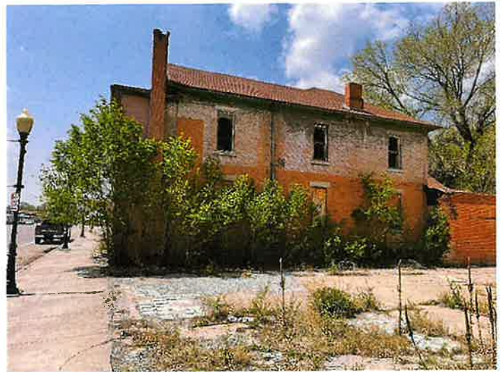
Structure 1 – North Elevation
