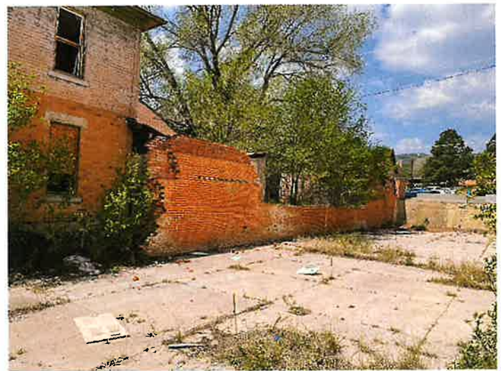
Vacant Lot and Retaining Wall
