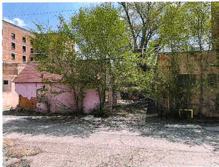
Structure 2 – West Elevation From Alley
