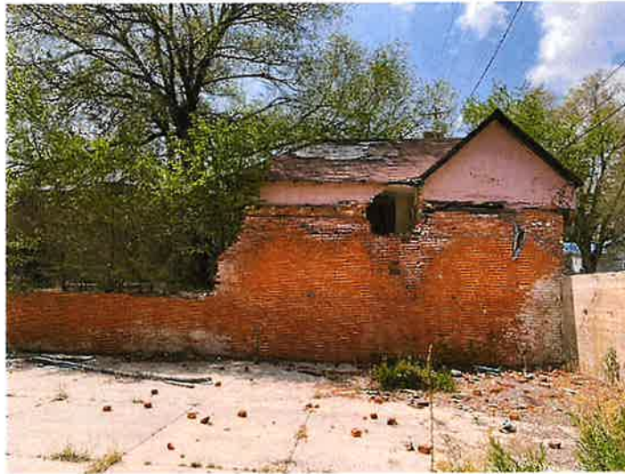
View of Structure 2 North Elevation
