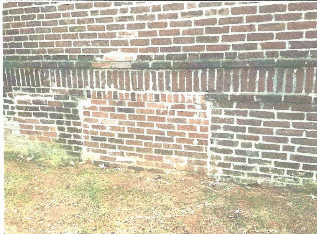
Remove and replace brick to provide access to the basement
