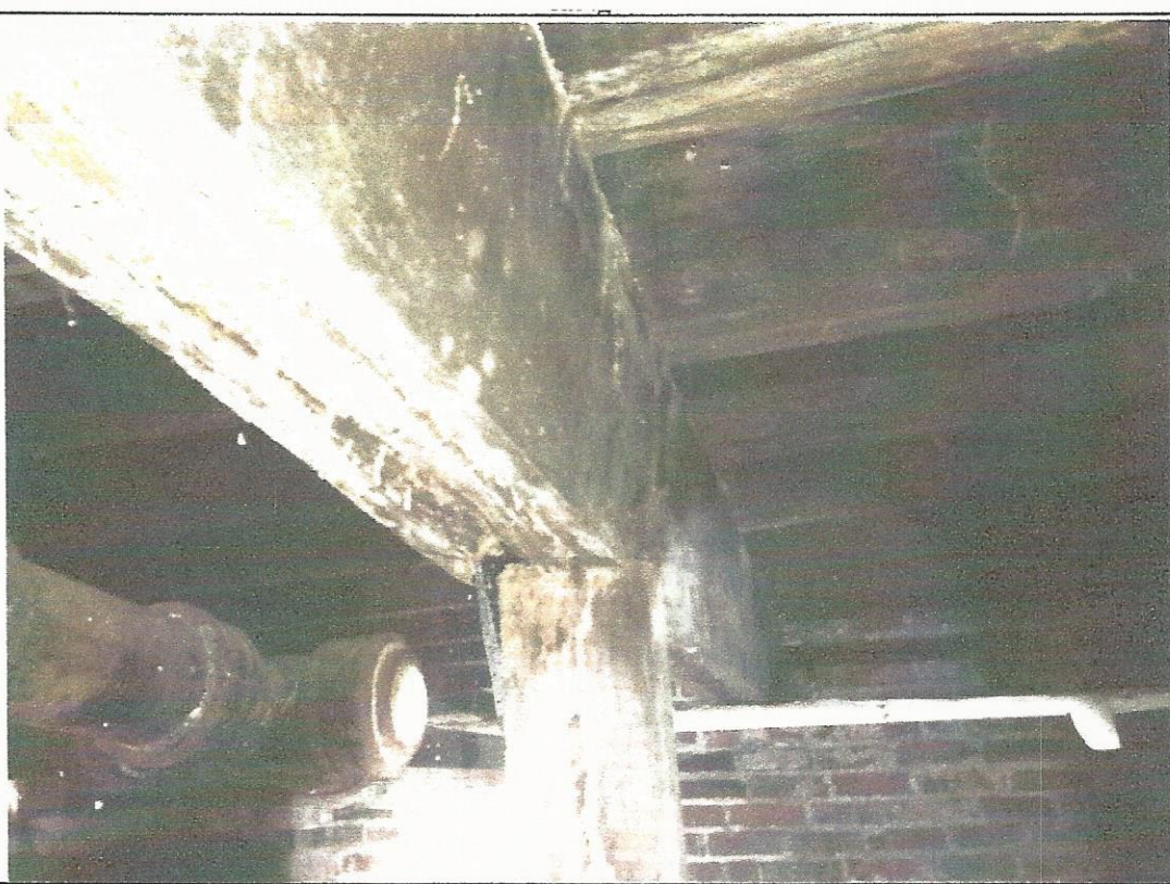
Install new beam alongside damaged, rotating beam
