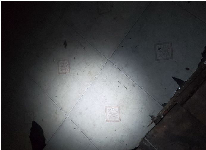
Photo 5 – 12x12 white self-stick flooring with diamond pattern located in room with fireplace.
