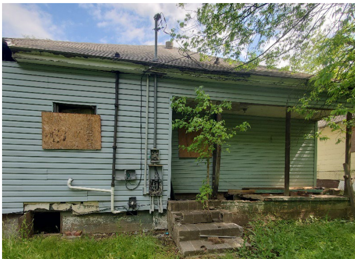
Photo 3 – Rear view of 1010 Carson Avenue.
