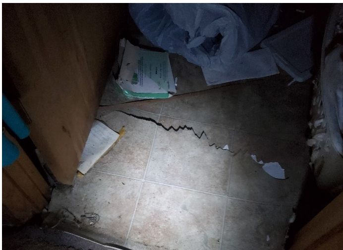
Photo 7 – Tan roll vinyl located within master bathroom.
