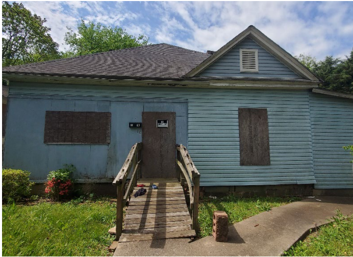
Photo 1 – 1010 Carson Avenue located in Spartanburg, South Carolina 29306
