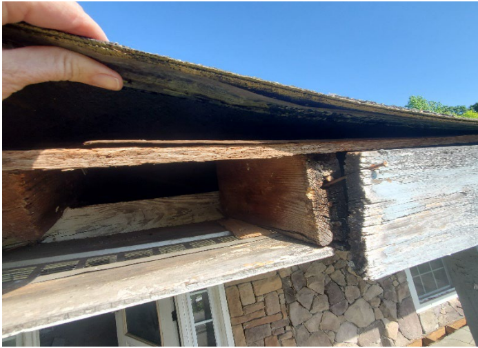
Photo 11 – Layer of shingles with one layer of felt located on the roof.
