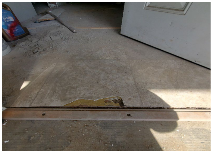
Photo 6 – White/gray roll vinyl flooring located in hallway entry.
