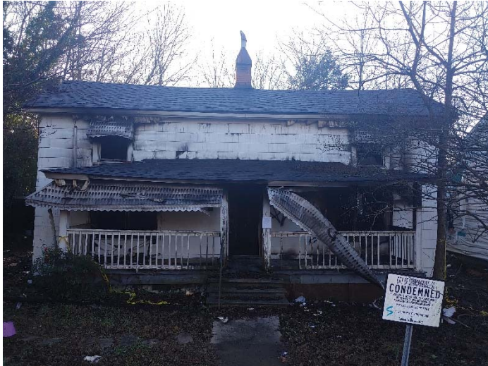
Photo 1 – 645 Isom Street located in Spartanburg, South Carolina 29303
