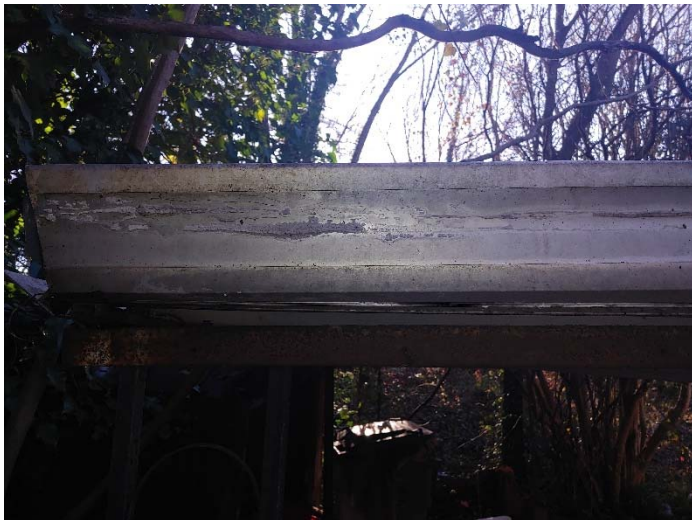
Photo 3 – Exterior carport/canopy with hard white caulk on the front side of the roof
