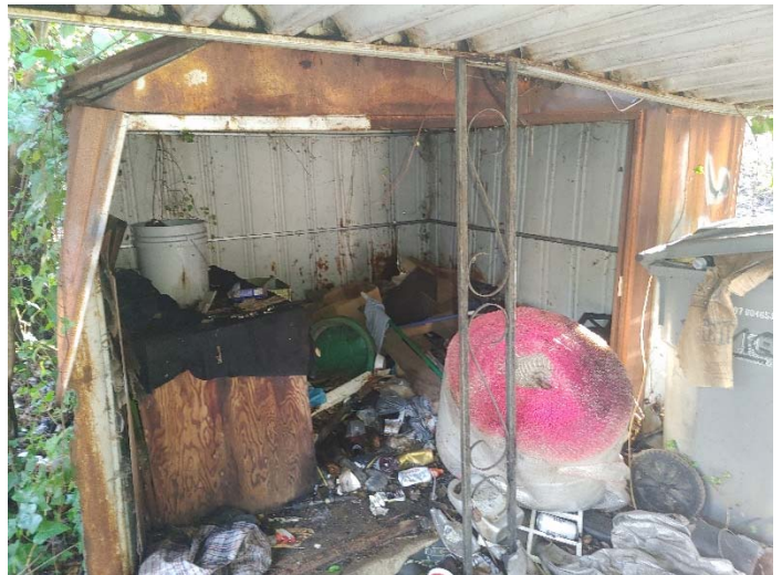
Photo 4 – Exterior metal shed with no suspect ACM identified
