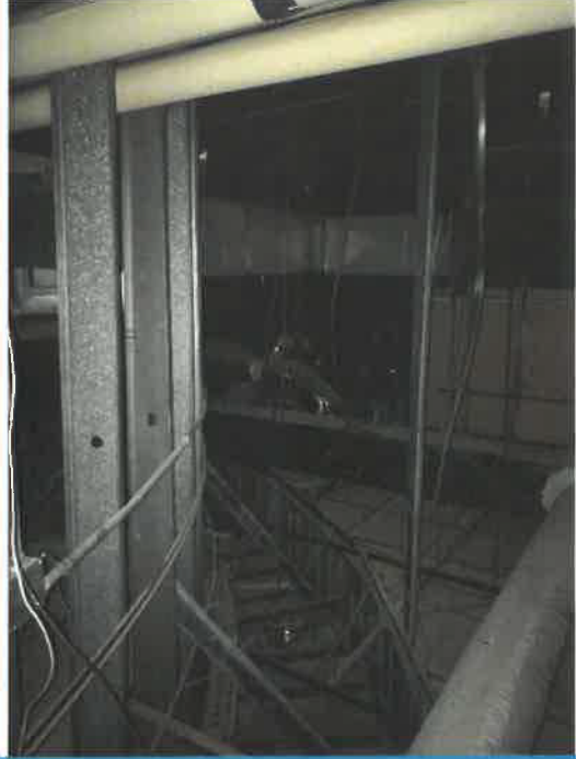
HVAC system and insulation piping above ceiling tiles in public lobby
