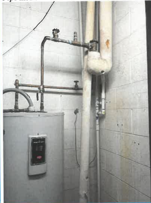
Pipe insulation elbows
