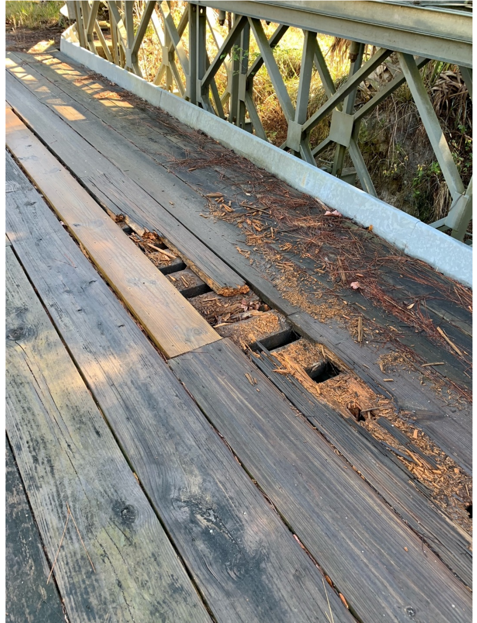
View of Stringers beneath Decking
