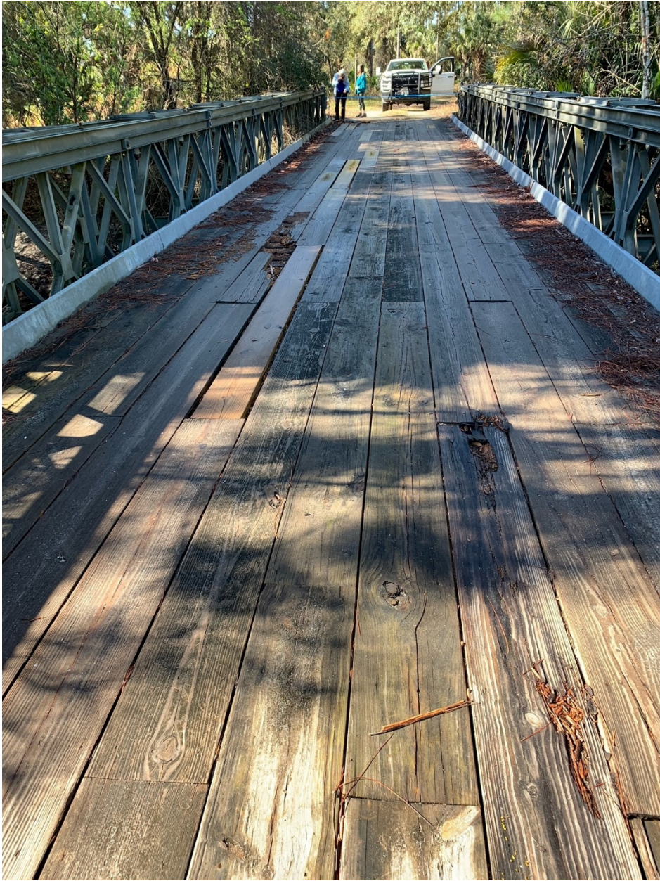
Existing Bridge Decking
