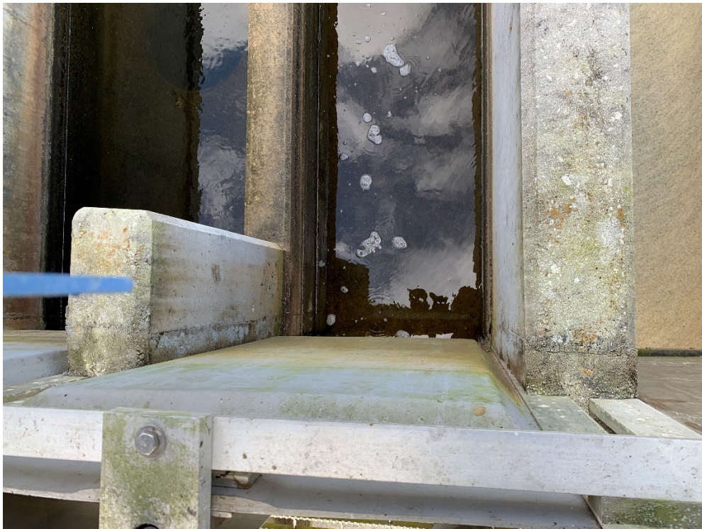
LOOKING DOWN ON SLIDE GATE #2 (NORTH SIDE)
