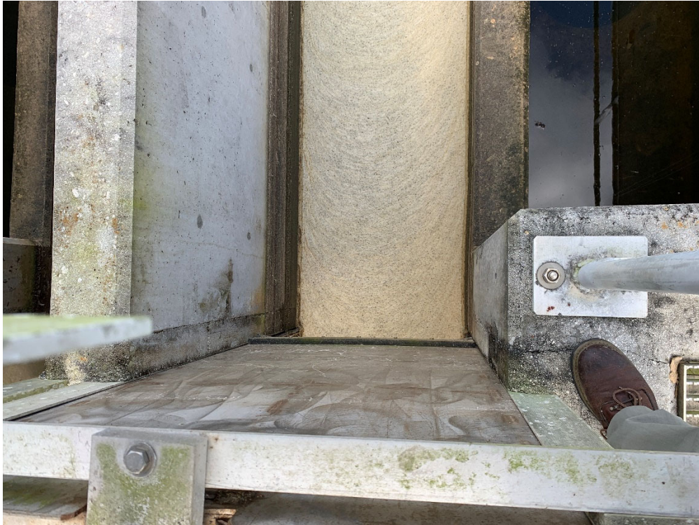
LOOKING DOWN ON SLIDE GATE #1 (NORTH SIDE)
