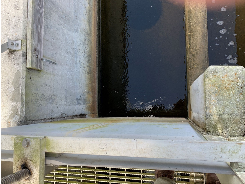
LOOKING DOWN ON SLIDE GATE #3 (NORTH SIDE)
