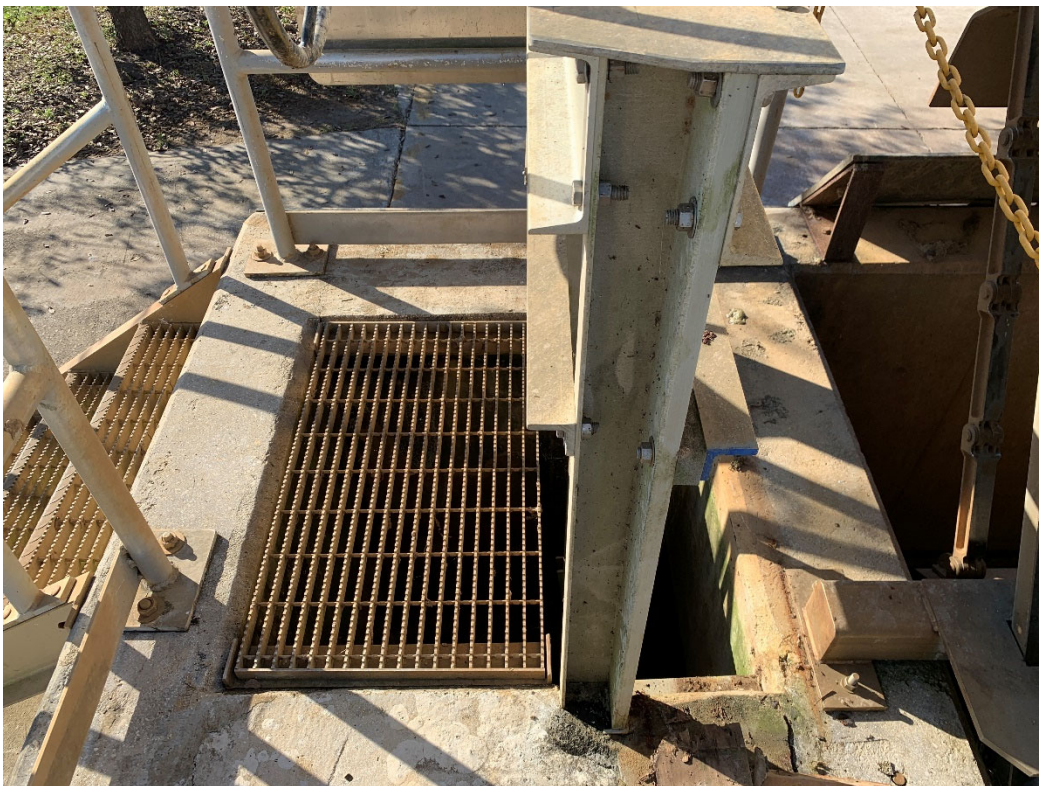
SLIDE GATE #4 SIDE VIEW (LOOKING SOUTH)
