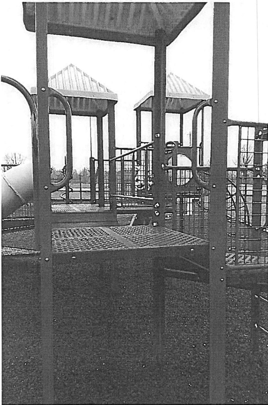
15. TPES- Missing barrier on 54.5" tall open platform
