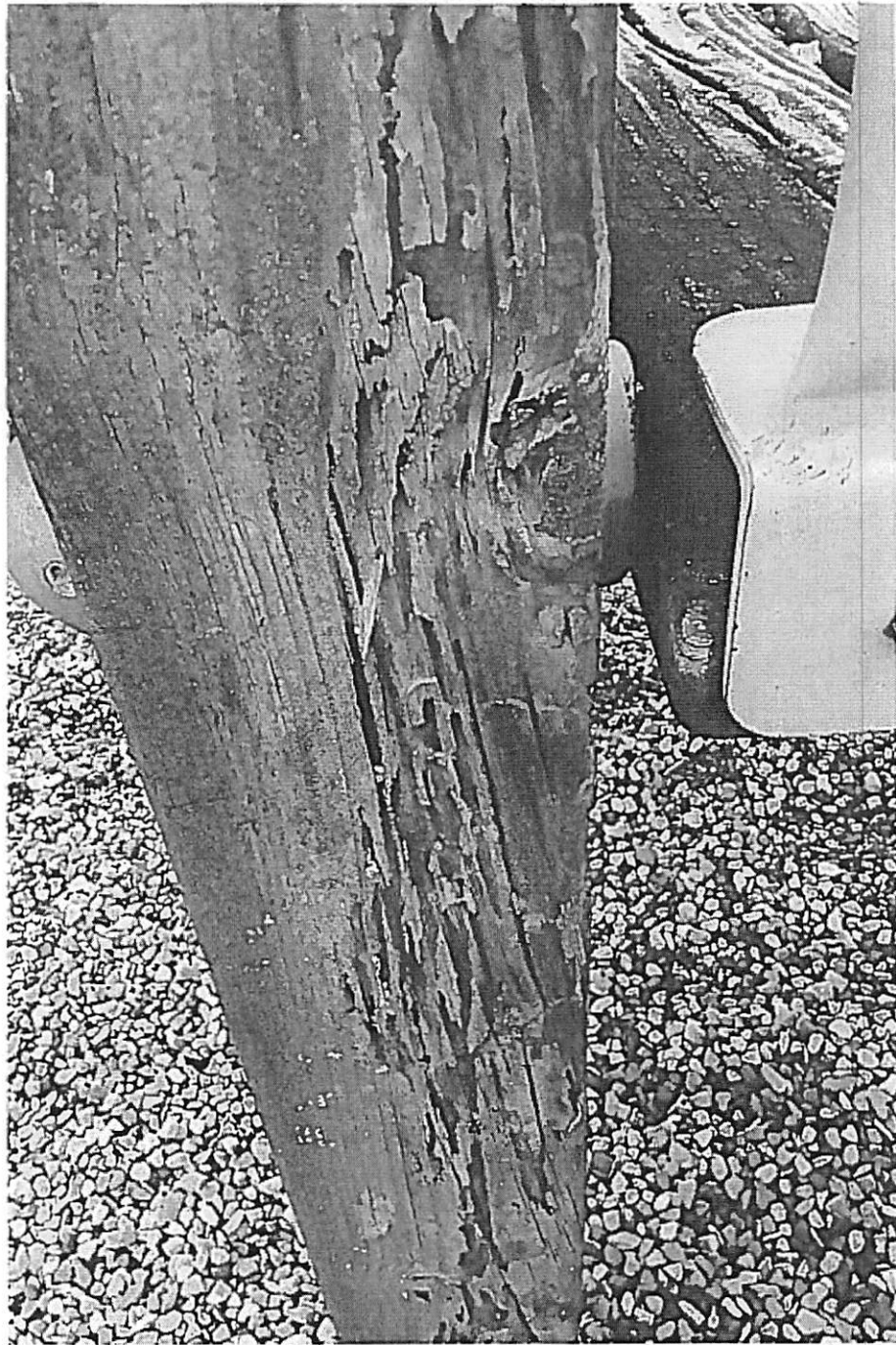
28. VES- Insect damage of wooden structure in pre-kindergarten area
