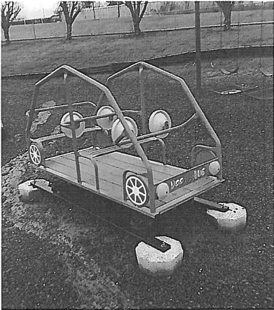
13. Tellico Plains Elementary School (TPES)- Pipe style car with no surfacing and exposed footers
