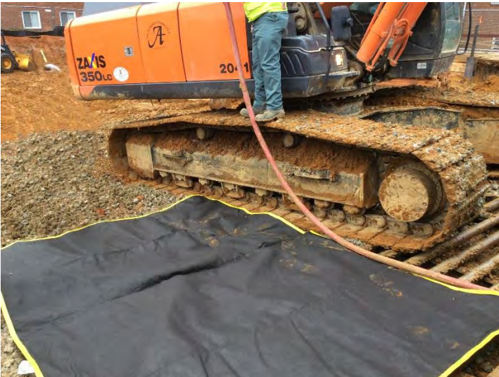
Portable refueling mat example. The mat catches drips that may occur during the fueling process.
