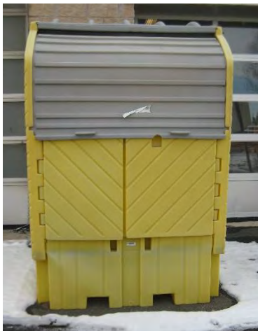
Example of a manufacturer's storage container. Note that the doors are closed and that the area surrounding the container is clean (except for some residual snow).
