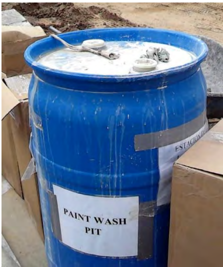
Example paint washout structure.
