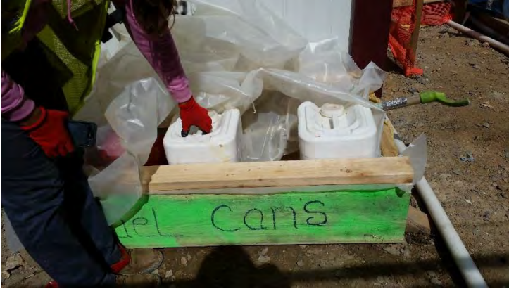
Fuel storage example. Cans are closed and located inside of a lined, secondary containment. The cans are also covered by a plastic liner to protect them from the elements.
