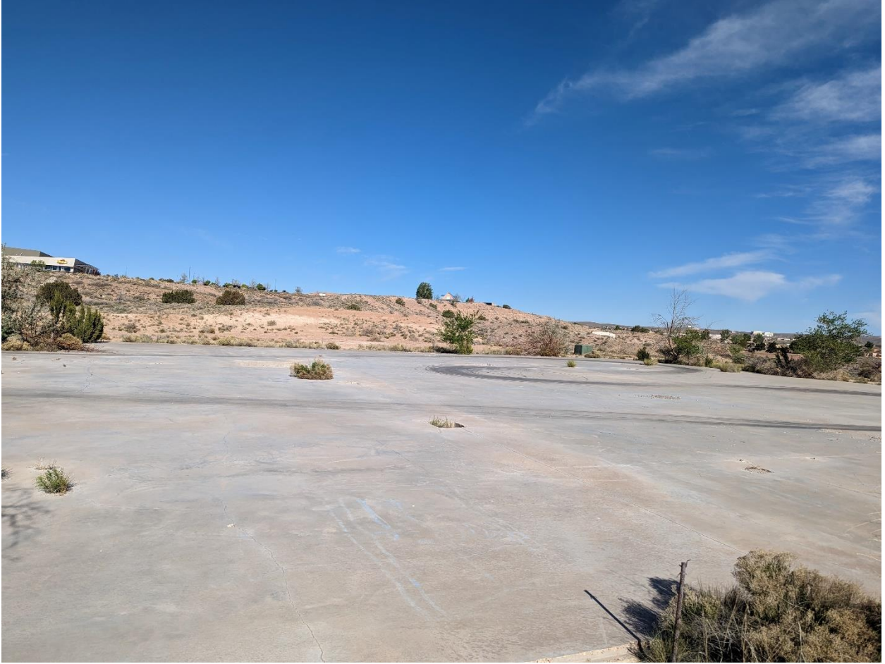
Concrete slab on lot 9A .jpg
