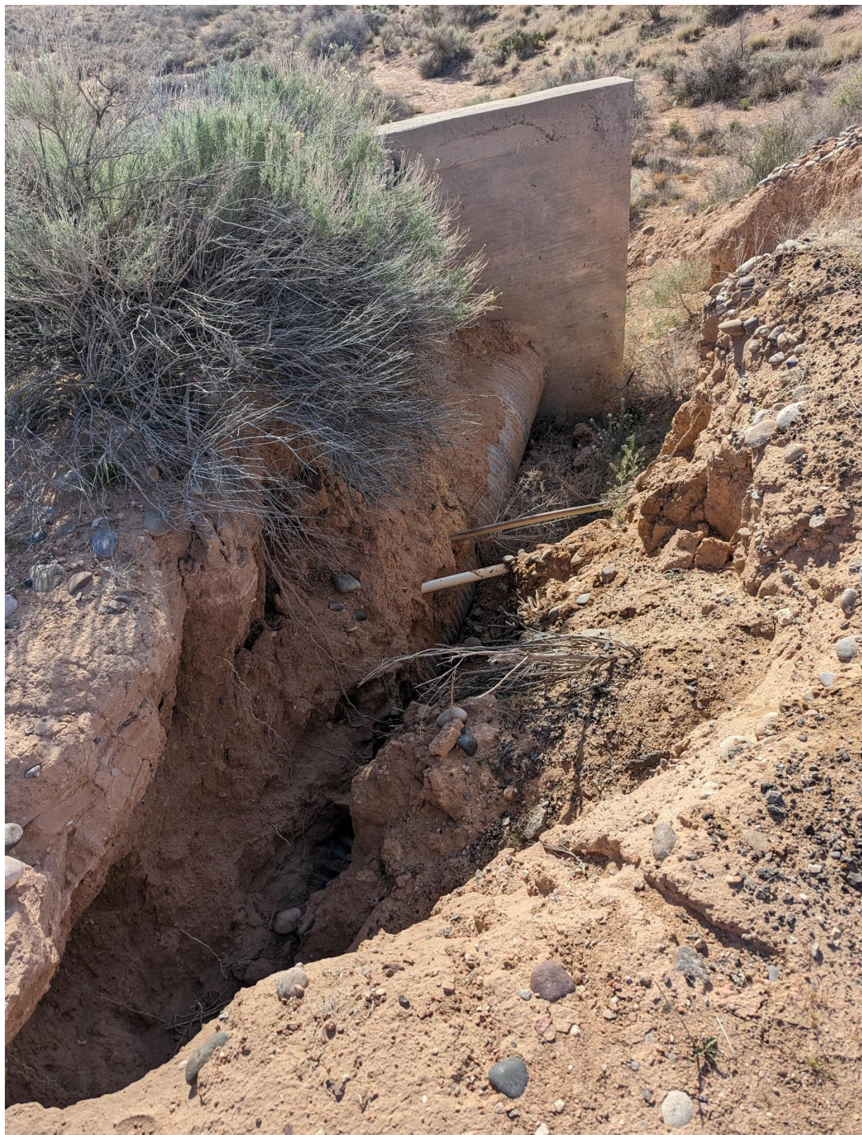
Storm drain on southwest corner of lot 10A pt.2 .jpg
