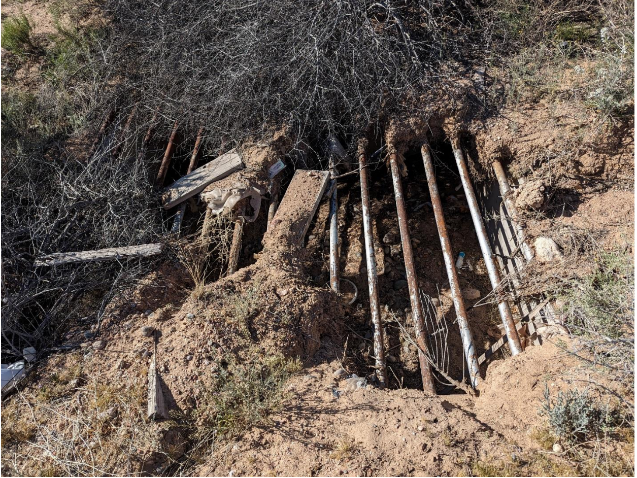
Storm drain south end of lot 10 A.jpg
