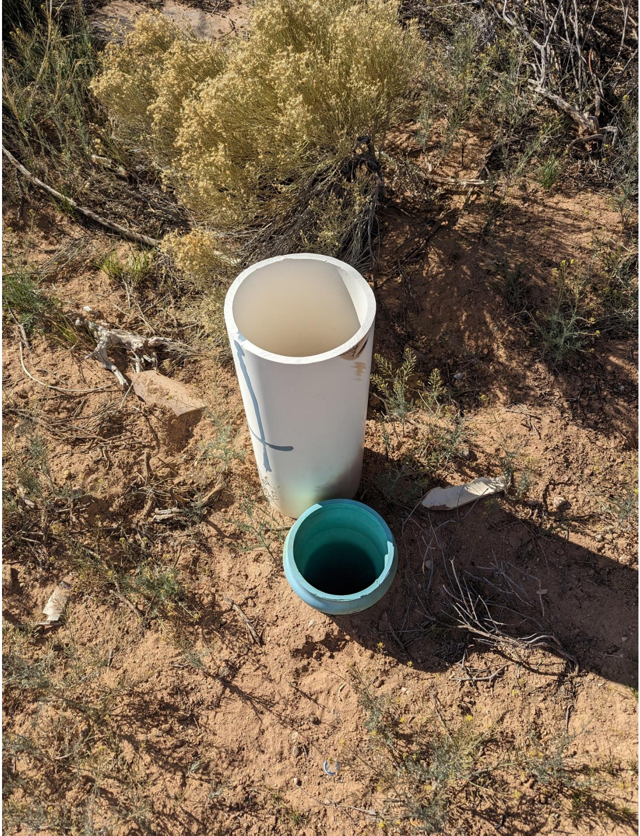
Pipes on lot 9A by concrete slab.jpg
