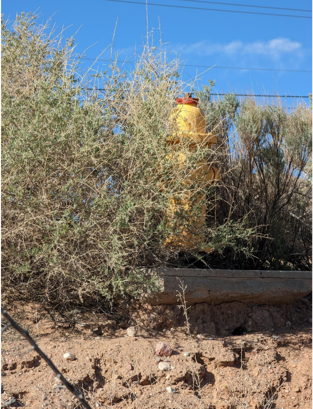
Fire hydrant on northwest corner of lot 9A .jpg
