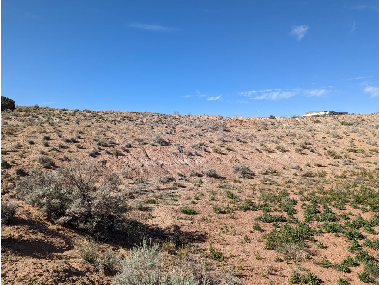
Storm drainage north end of lot 9A pt.2 .jpg
