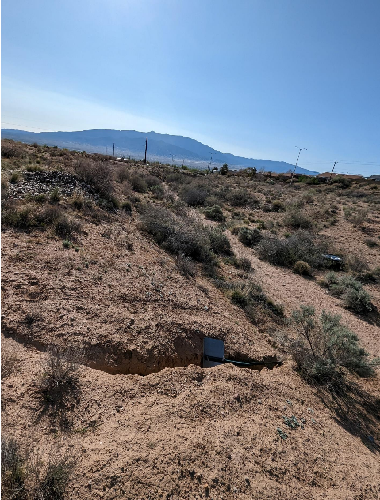
Storm drain channel south end of lot 9A .jpg
