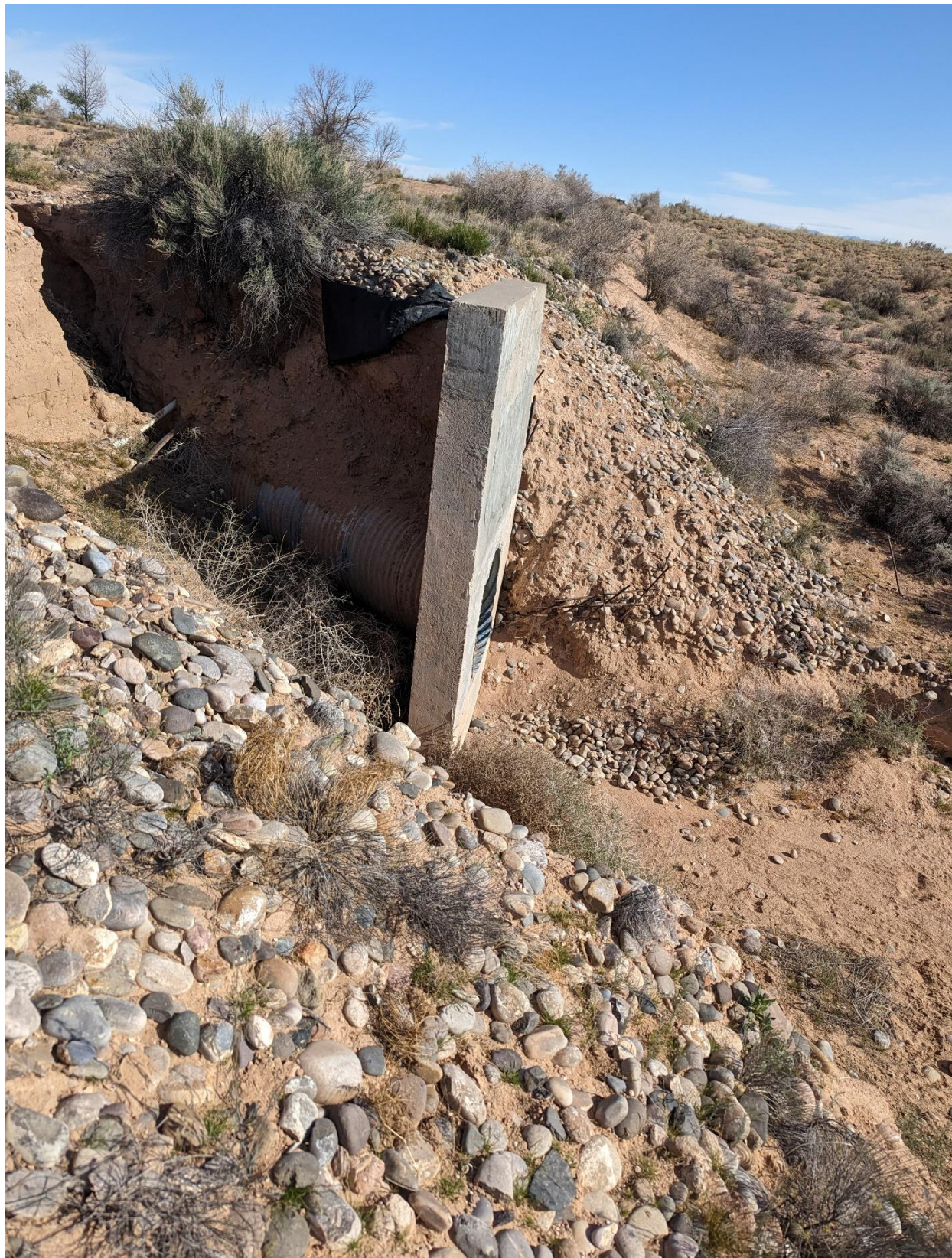
Storm drain on southwest corner of lot 10A pt.1 .jpg
