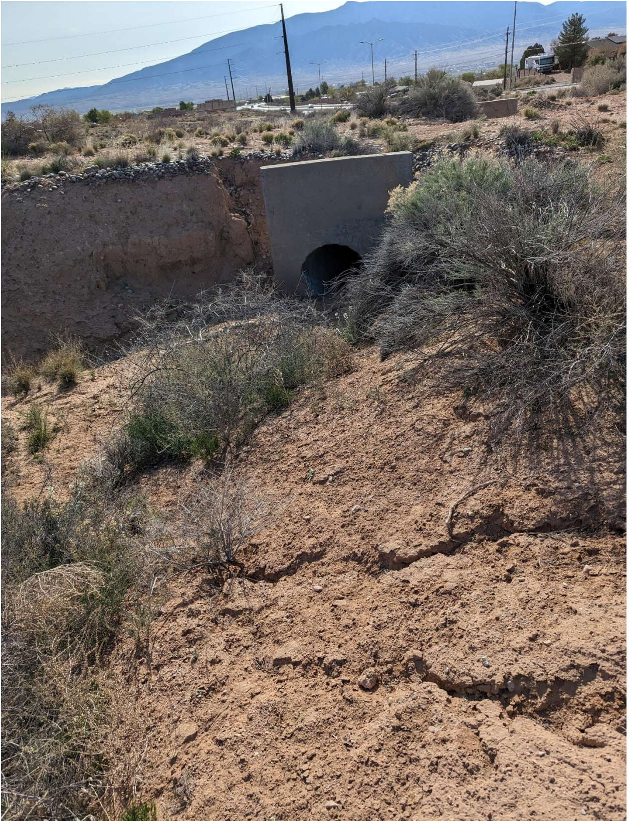
Storm drain on southeast side of lot .jpg
