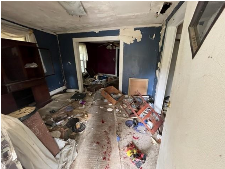
Inside of structure
