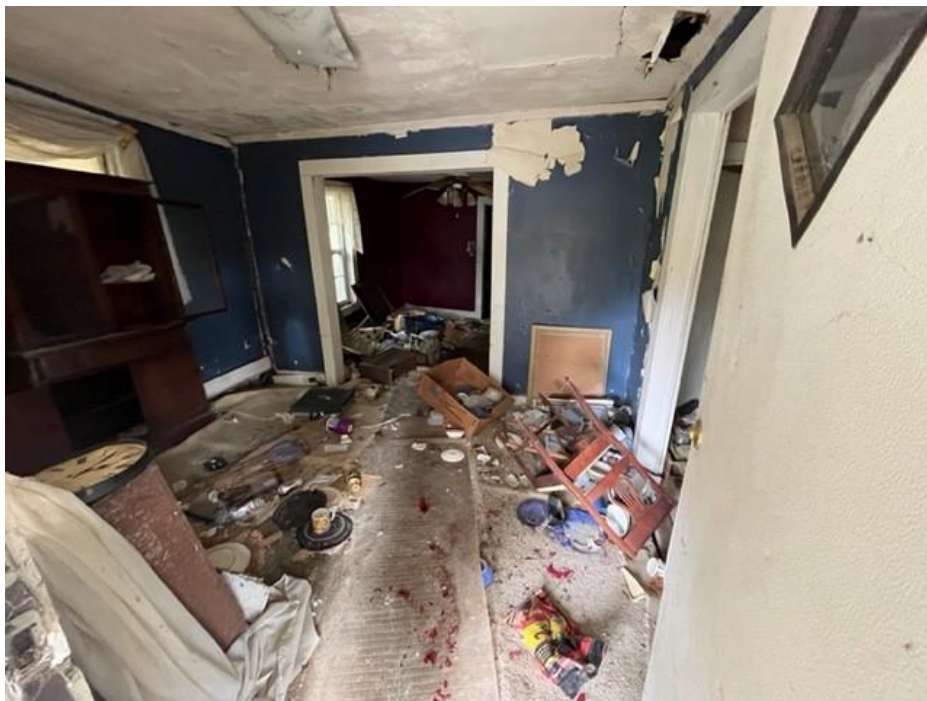
Inside of structure
