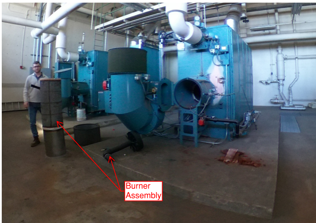
Figure 3. B-2 burner assembly.
