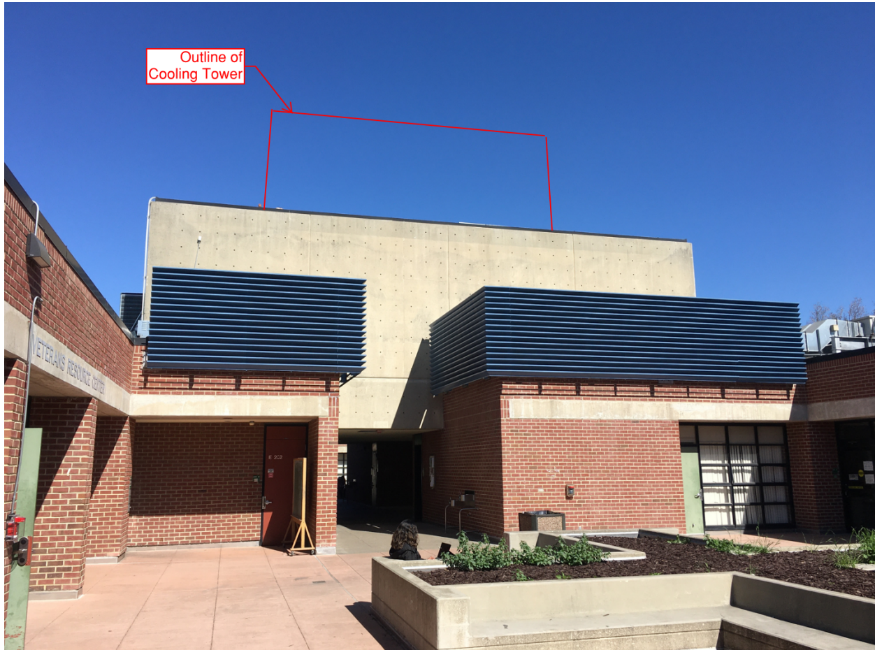
Figure 7. Field image of potential cooling tower on Building E penthouse roof. Location 1.
