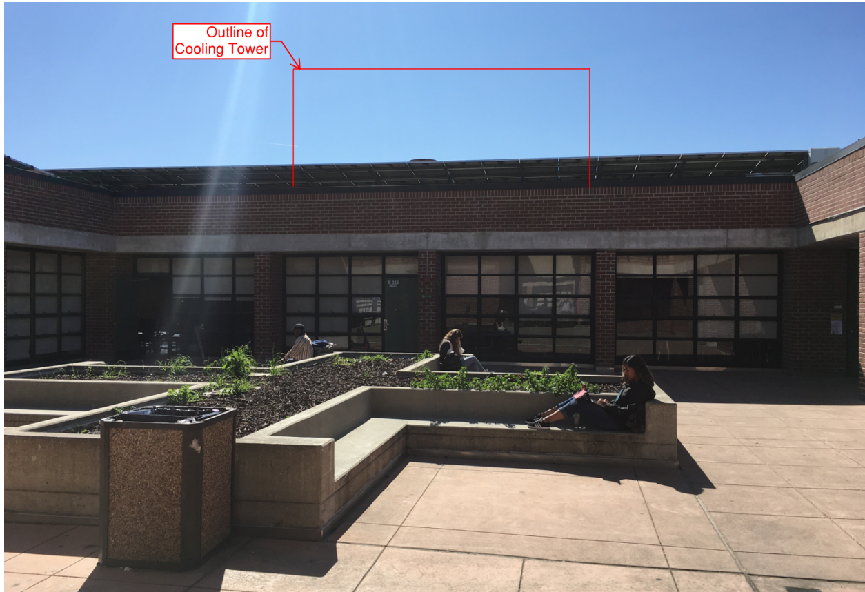
Figure 9. Field image of potential cooling tower location on Building E roof. Location 2.
