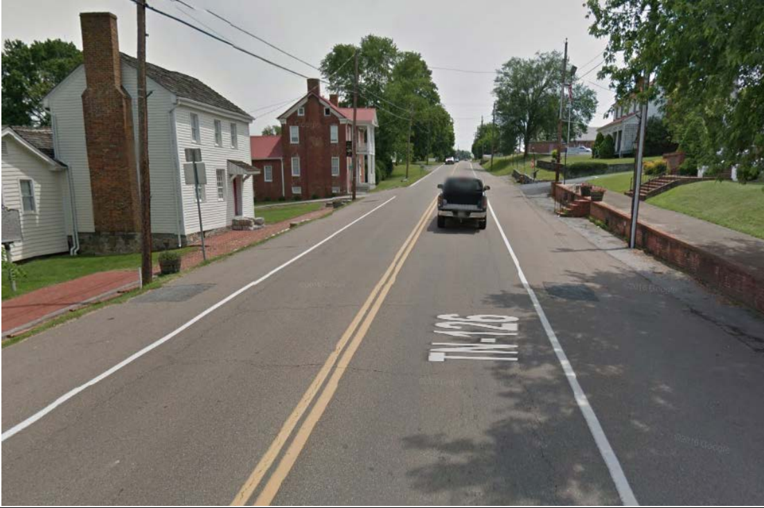
BEGIN PROJECT (SR-126, NEAR SR-394)
