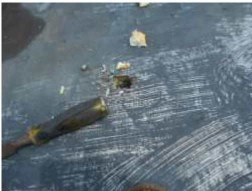
HOMOGENEOUS AREA 05 ROOF CORE (HIGH ROOF)
