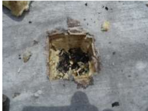
HOMOGENEOUS AREA 04 ROOF FLASHING (HIGH ROOF)
