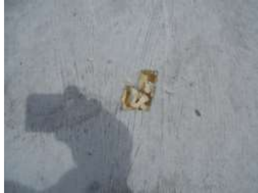
HOMOGENEOUS AREA 02 ROOF CORE (LOW ROOF)
