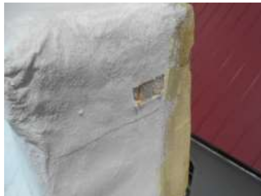
HOMOGENEOUS AREA 06 CLOTH (HIGH ROOF)
