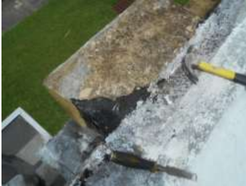
HOMOGENEOUS AREA 01 ROOF FLASHING (LOW ROOF)
