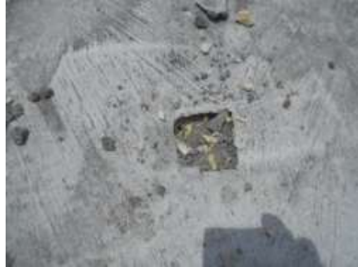
HOMOGENEOUS AREA 08 ROOF CORE (LOW ROOF)
