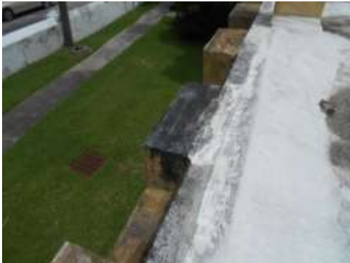
HOMOGENEOUS AREA 03 TAR APPLICATION (LOW ROOF)
