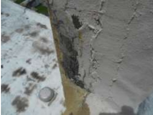
HOMOGENEOUS AREA 07 ROOF FLASHING (LOW ROOF)
