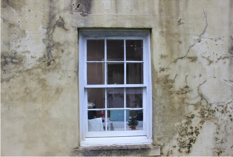
**Figure 158:** Biogrowth is present throughout the masonry opening.
