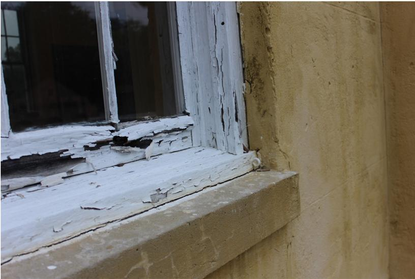
**Figure 36:** The lower sash is completely deteriorated.
