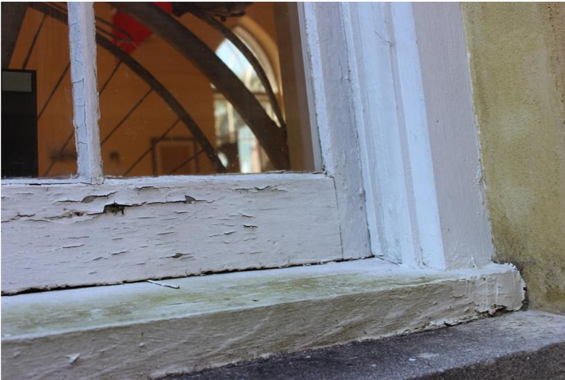
**Figure 108:** The bottom rail of the lower sash is deteriorated.
