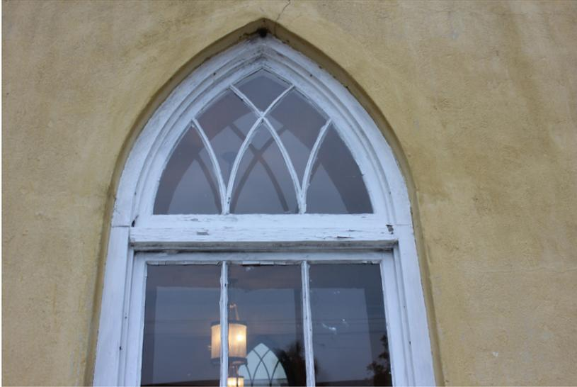
**Figure 47:** The transom bar is heavily weathered.
