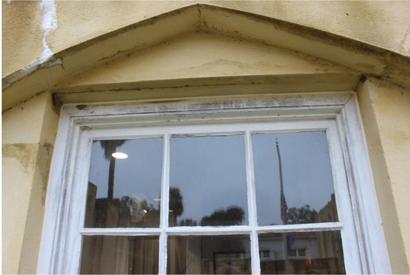
**Figure 56:** The masonry opening is cracked above the head of the window.
