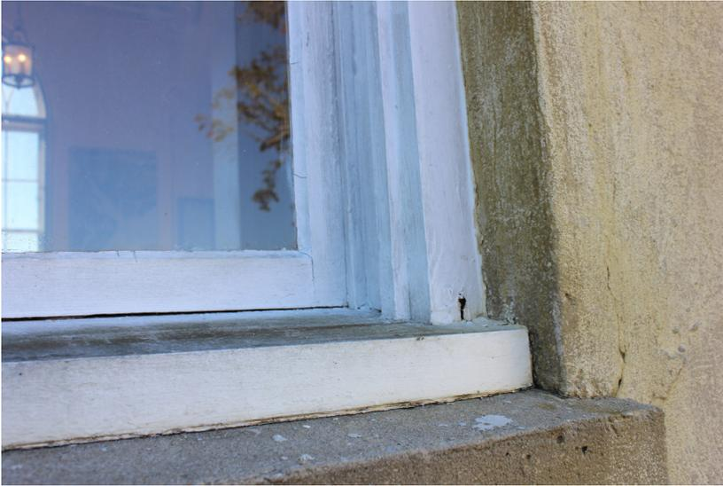
**Figure 92:** Ferrous fasteners within the window are actively corroding.
