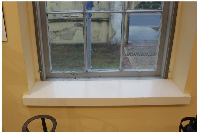
**Figure 37:** The lower sash is completely deteriorated and visible on the interior of the window.
