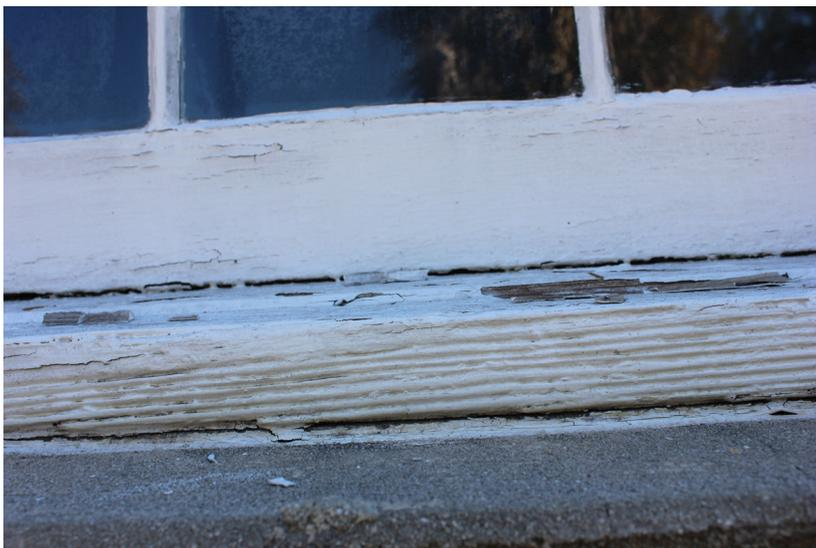
**Figure 144:** The sill is heavily weathered.
