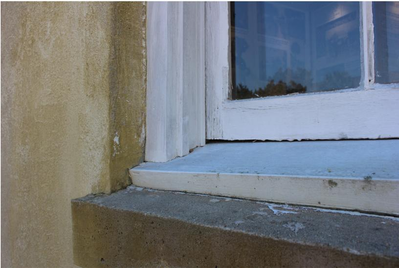
**Figure 88:** The sill is in good condition. There is moderate separation of the joints within the wooden window.
