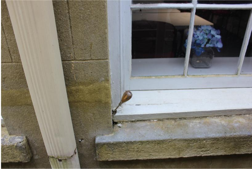
**Figure 139:** The sill is deteriorated on the left hand side.
