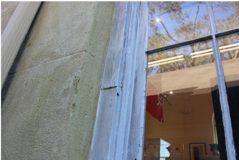
**Figure 6:** Category 2 windows commonly contain dutchman repairs that are actively separating.
