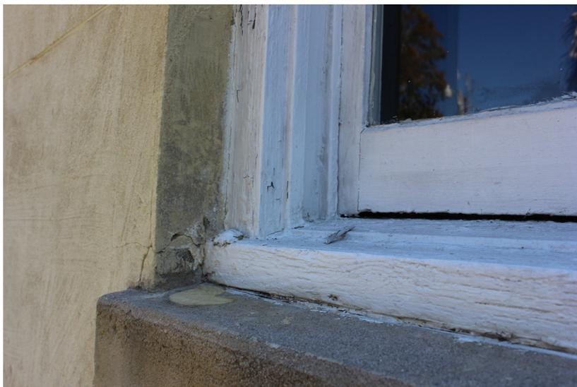
**Figure 148:** The sill is weathered but sound.
