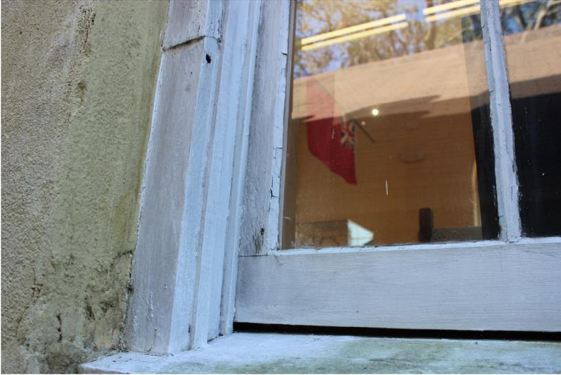
**Figure 111:** Detail of dutchman repair that is separating at the joints.
