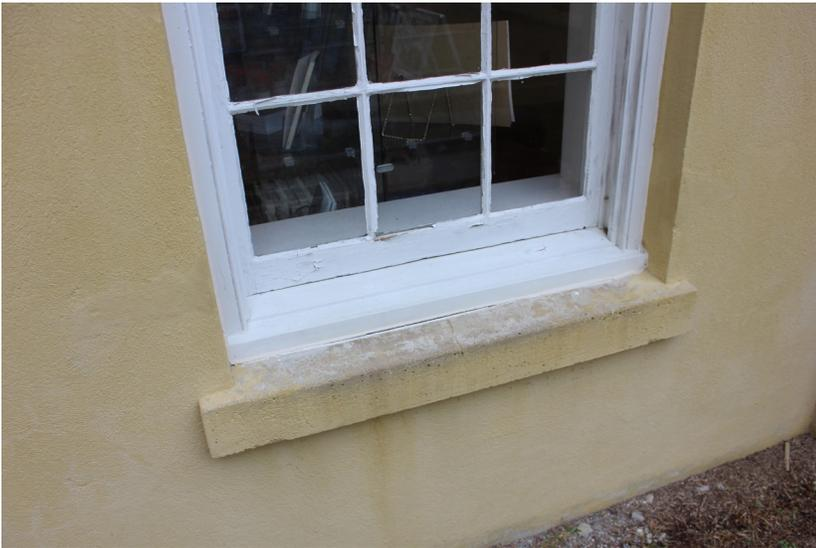
**Figure 68:** The bottom rail of the lower sash is weathered but sound.
