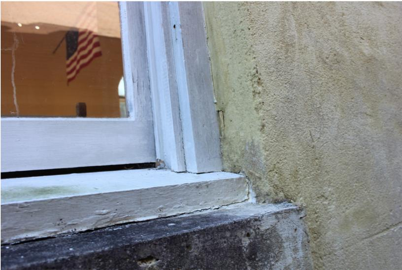
**Figure 112:** A large gap is present between the lower sash and the sill.
