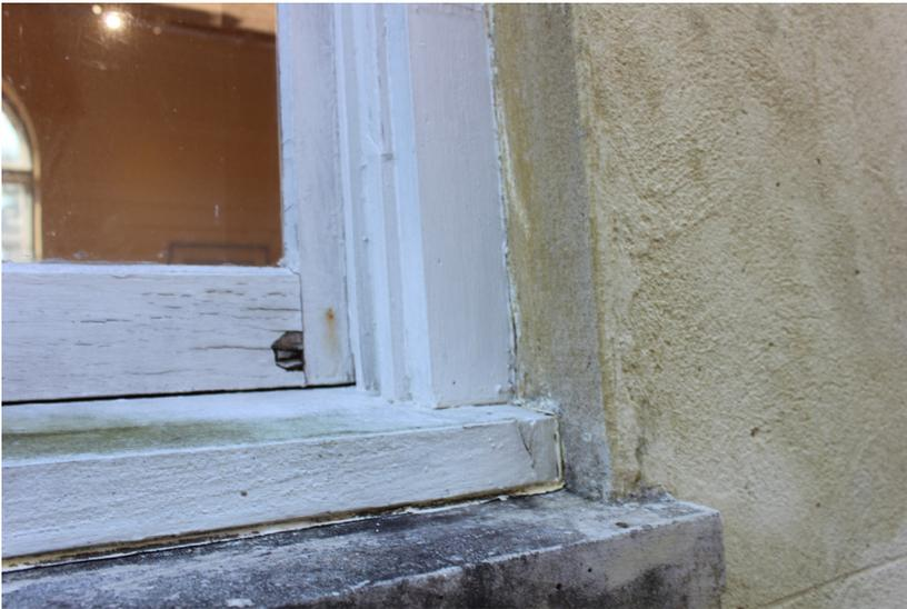
**Figure 120:** Detail of sash deterioration.
