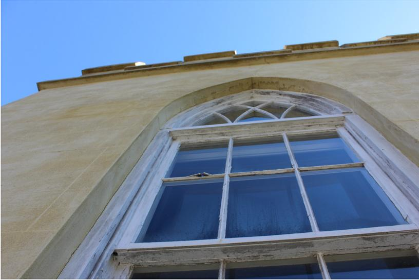
**Figure 142:** A muntin is broken on the upper sash. Select areas of the sill are deteriorated.
