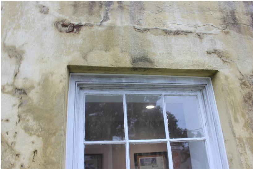
**Figure 163:** Biogrowth is present throughout the window and the masonry opening.
