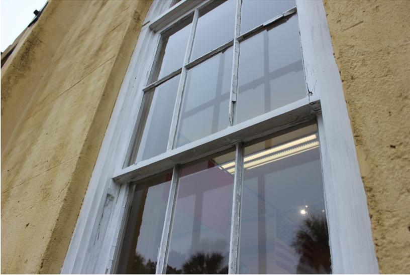
**Figure 31:** The right stile of the upper sash is deteriorated. A broken muntin is also visible within the upper sash.
