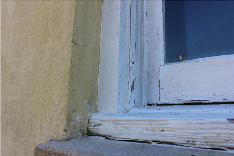
**Figure 143:** Separation was noted within the lower sash.
