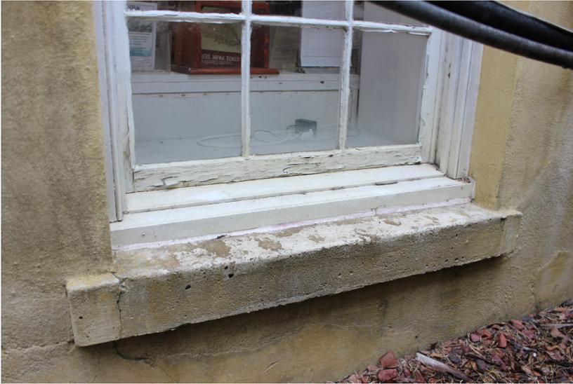
**Figure 80:** Glazing putty and paint failure is present throughout the window.
