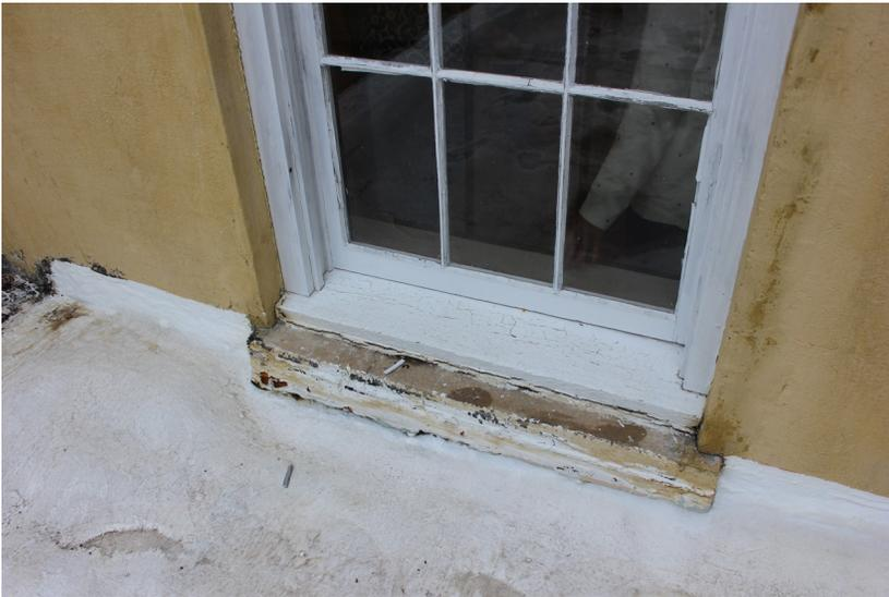
**Figure 48:** The sill is heavily weathered.
