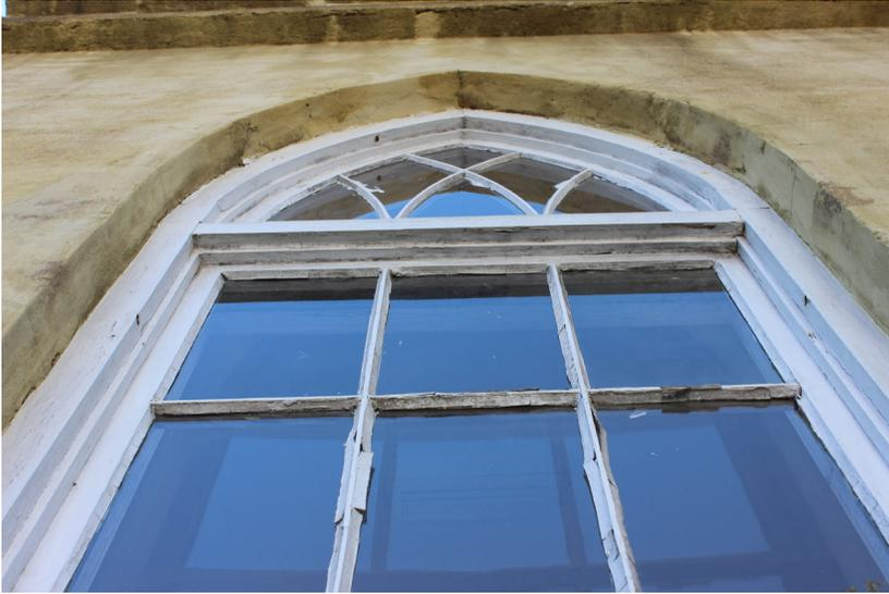
**Figure 99:** A dutchman repair is present within the transom casing.
