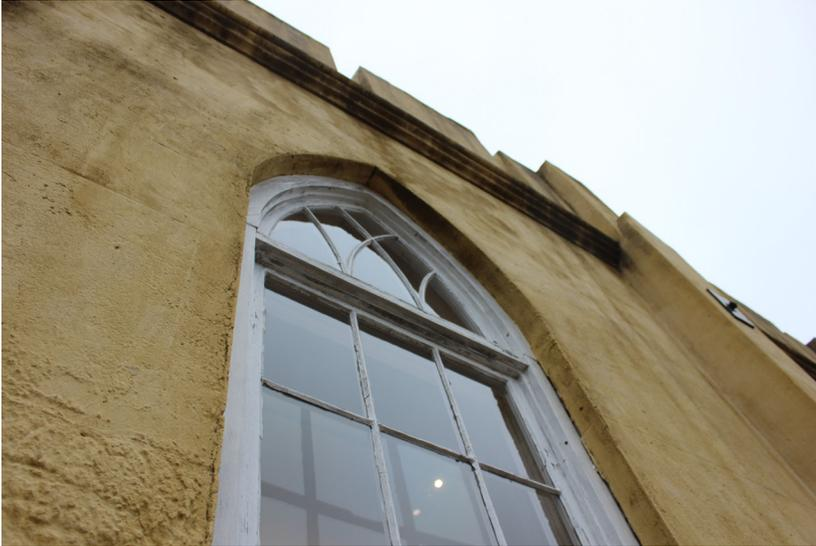
**Figure 35:** The transom casing is proud of the lower window casing.
