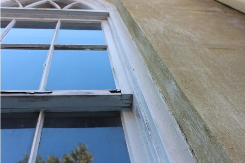
**Figure 127:** The lower rail of the upper sash is deteriorated.
