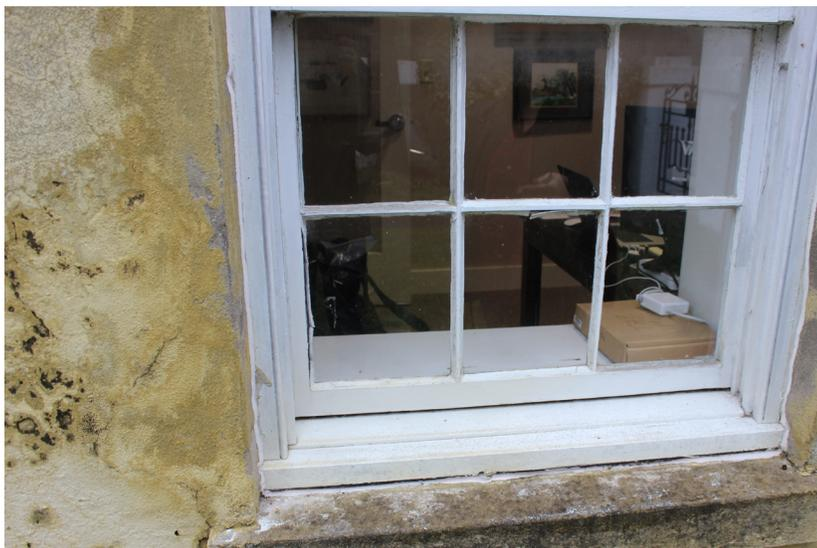
**Figure 164:** Detail of interior conditions at the stool the location of the and gap between sill and lower sash.
