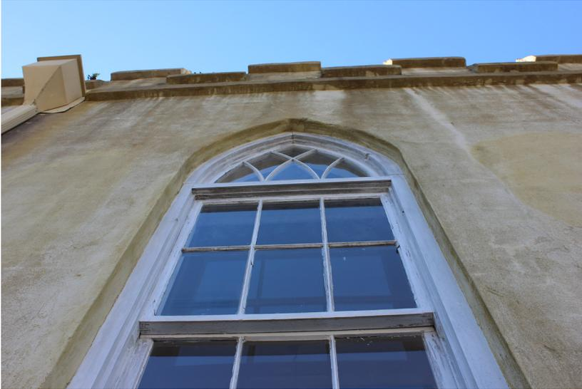
**Figure 87:** There is extensive glazing and paint failure throughout the window.
