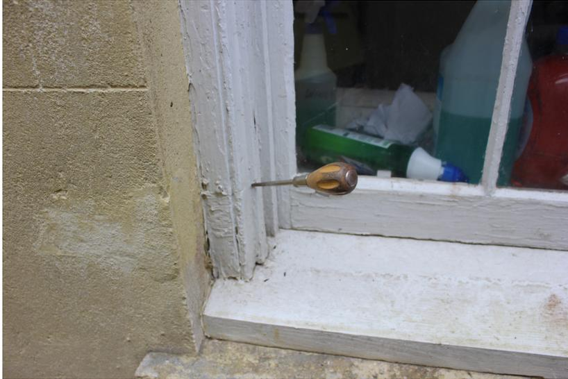
**Figure 131:** The casing and jamb are deteriorated at this location.
