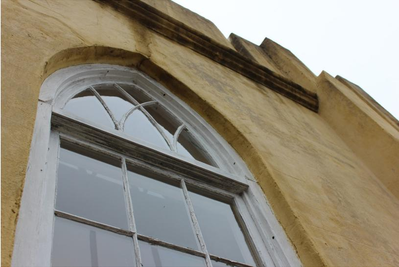
**Figure 43:** The transom casing is slightly proud of the lower window casing. A pane of glass is broken within the transom.
