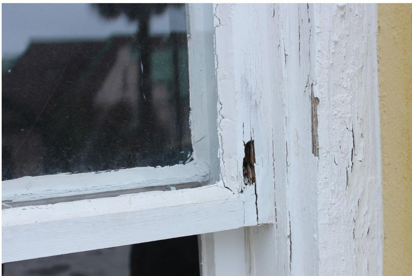
**Figure 13:** The upper sash is deteriorated at the intersection of the right stile and bottom rail.
