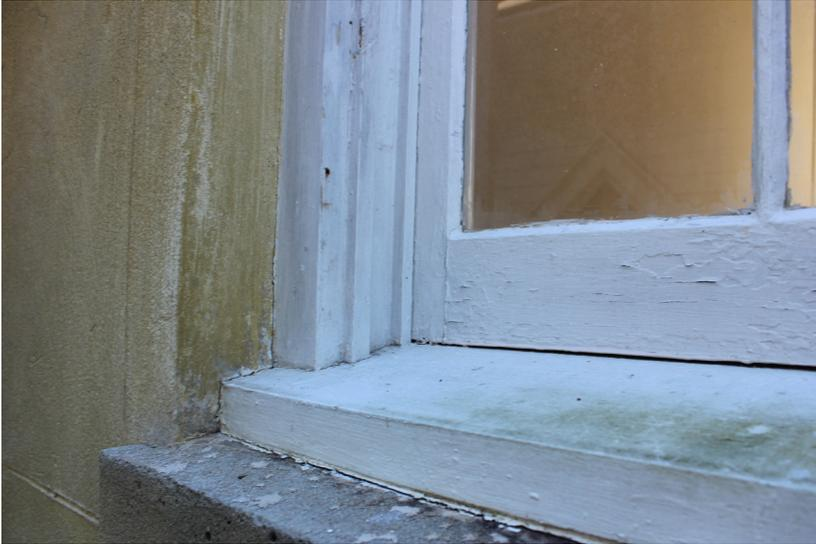
**Figure 123:** The sill is in good condition. Biogrowth is present throughout.
