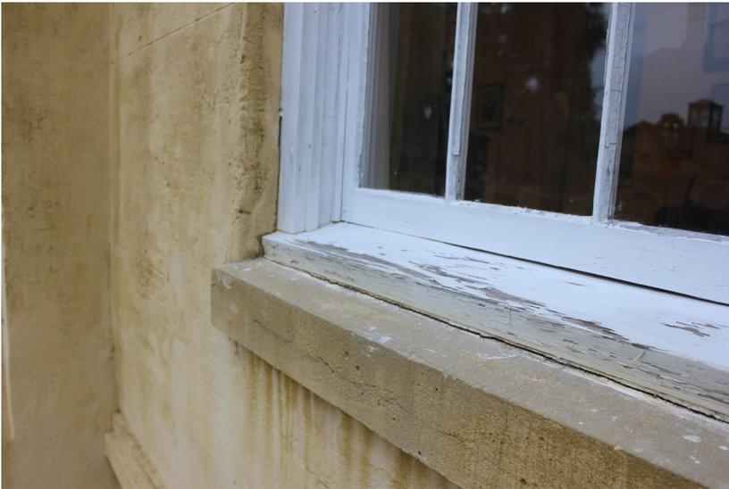
**Figure 32:** The bottom rail of the lower sash is deteriorated and requires replacement.
