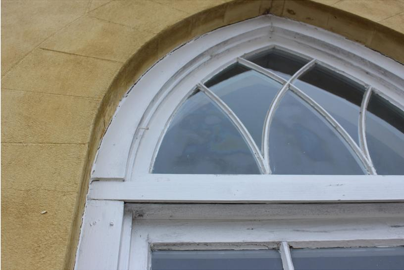
**Figure 11:** The casing of the transom window does not align with the lower casing.
