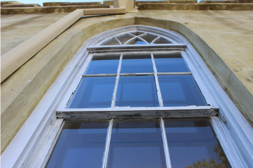
**Figure 95:** The upper sash is damaged and is cracking along the stiles.
