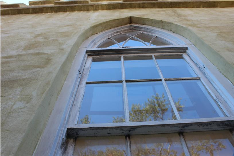
**Figure 107:** The transom casing is proud of the lower casing.
