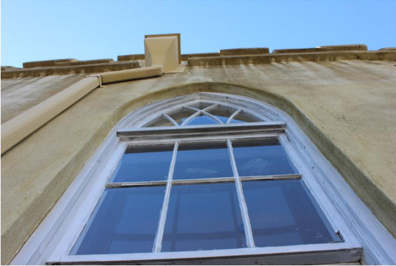
**Figure 91:** There is extensive glazing and paint failure throughout the window.
