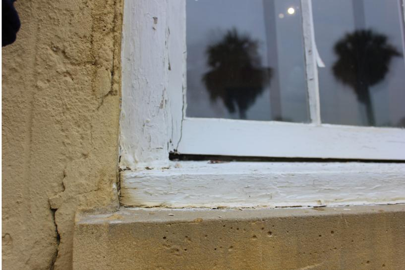
**Figure 4:** Category 2 windows typically have evidence of deterioration or excessive weathering on the casing and the sills.
