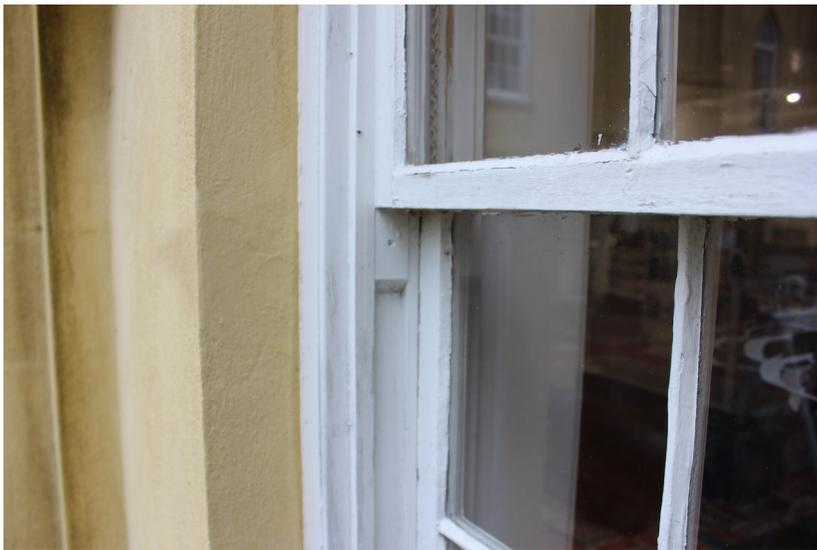
**Figure 64:** Glazing putty and paint failure is present throughout the window.
