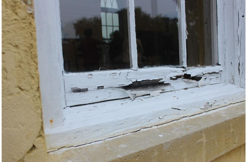
**Figure 8:** Common failures include deterioration at the meeting rail and the bottom rail of the lower sashes.
