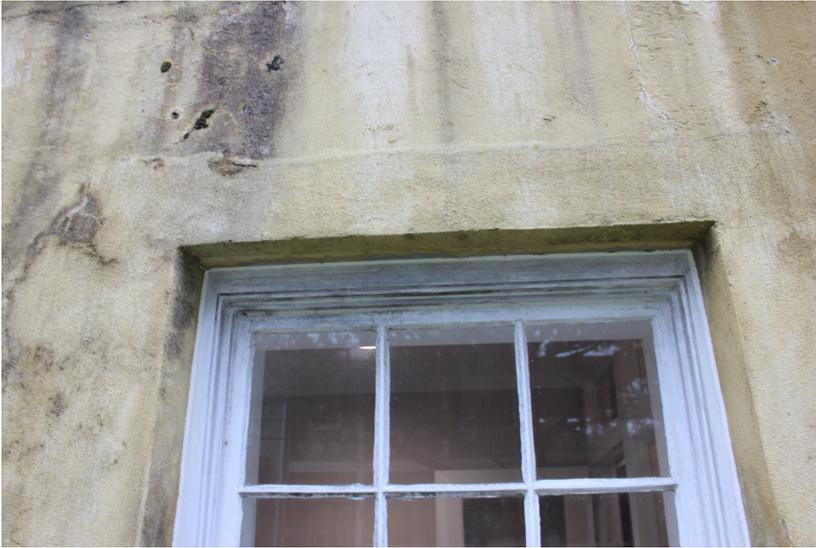
**Figure 159:** The wooden elements are in good condition.
