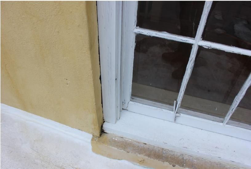
**Figure 52:** The lower sash is deteriorated on the right hand side.
