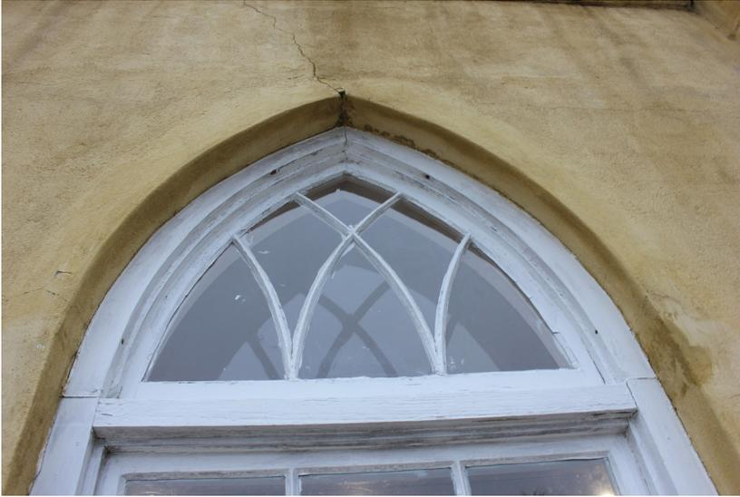
**Figure 51:** The transom casing is beginning to separate at the joints. The glass is in good condition.
