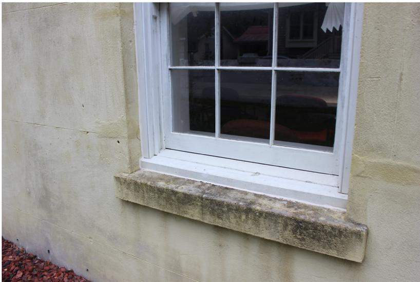
**Figure 155:** A small gap is present between the lower sash and the wood will.
