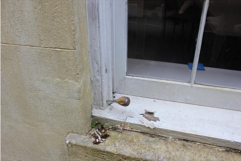
**Figure 134:** The bottom of the casing on the left hand side is deteriorated.
