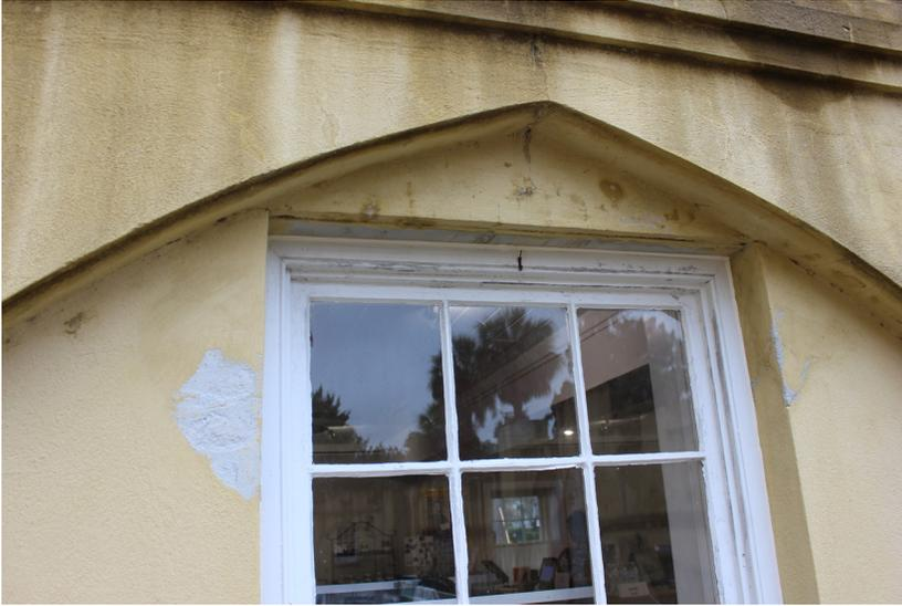
**Figure 67:** A small gap is present between the steel lintel and the wood casing at the head of the window.
