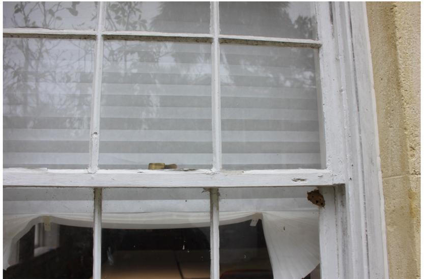
**Figure 3:** Detail of casing of transom windows that is proud of the lower casing. This condition is typical on the second-floor windows.
