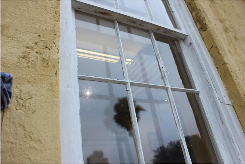
**Figure 24:** There is extensive paint and glazing failure throughout the window.
