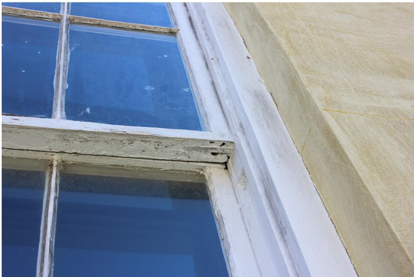
**Figure 147:** Detail of separation with the bottom of the lower sash.
