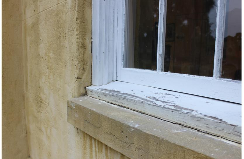
**Figure 2:** Glazing putty failure is prominent feature on all the inspected windows.
