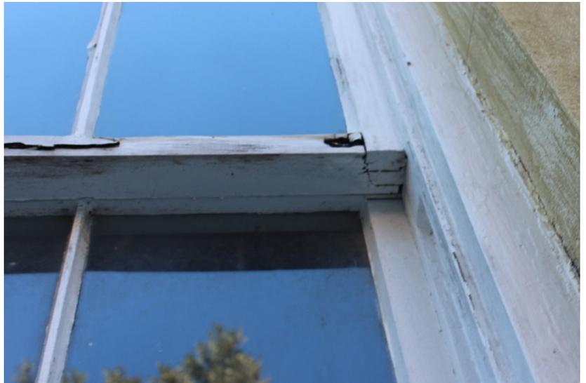
**Figure 9:** Detail of deterioration on a fixed casement window.
