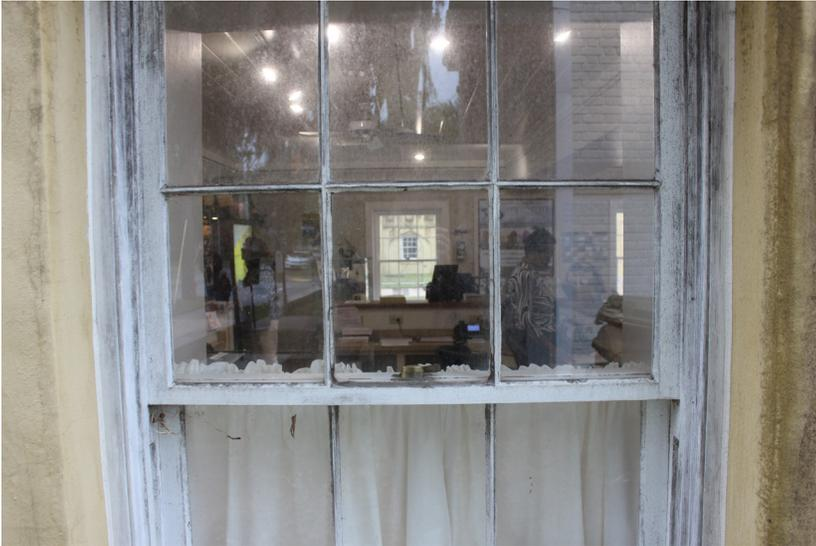
**Figure 72:** The woodwork is in fair condition. Biogrowth is present on the wooden elements.
