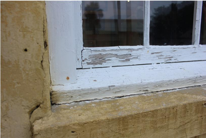
**Figure 28:** The bottom rail of the lower sash is heavily weathered and is separating at the joints.
