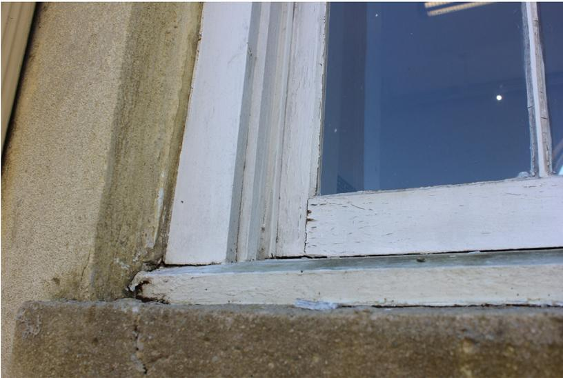
**Figure 96:** Detail of separation at the joints within the lower sash.
