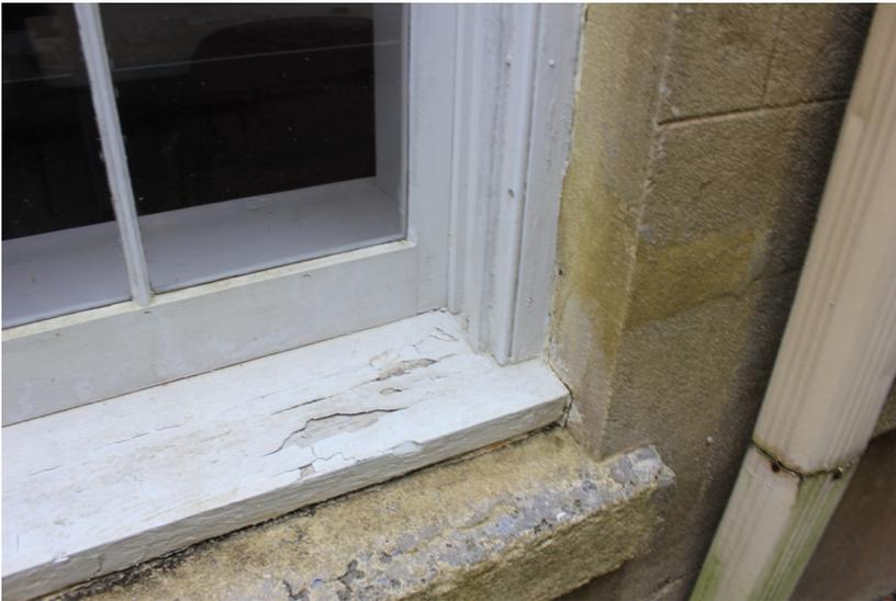
**Figure 135:** The sill is heavily weathered and checked but is sound.
