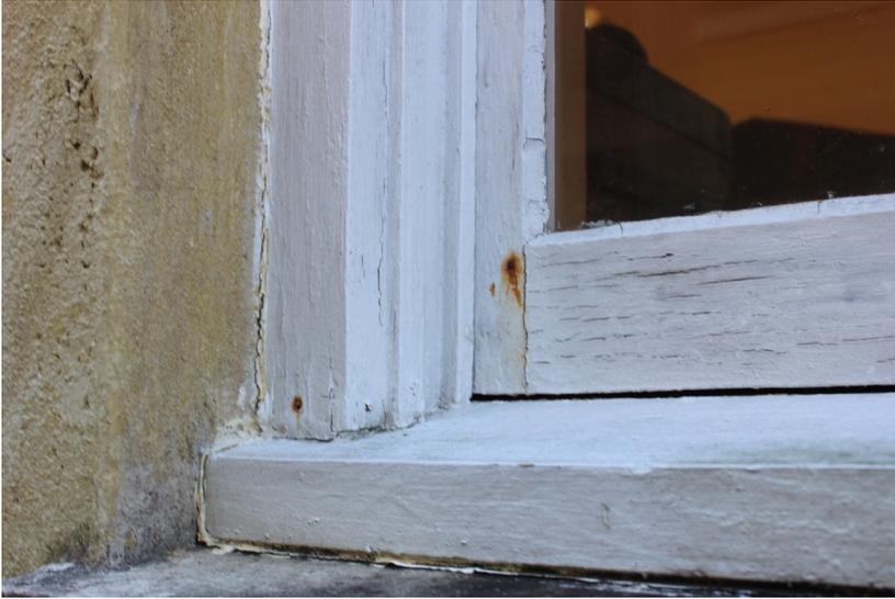
**Figure 119:** The ferrous fasteners within the window are actively corroding.
