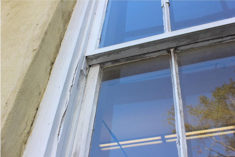
**Figure 100:** Detail of paint and glazing failure.
