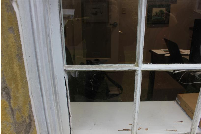
**Figure 162:** Detail of glazing failure
