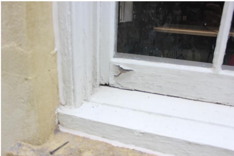
**Figure 151:** Detail of paint failure.
