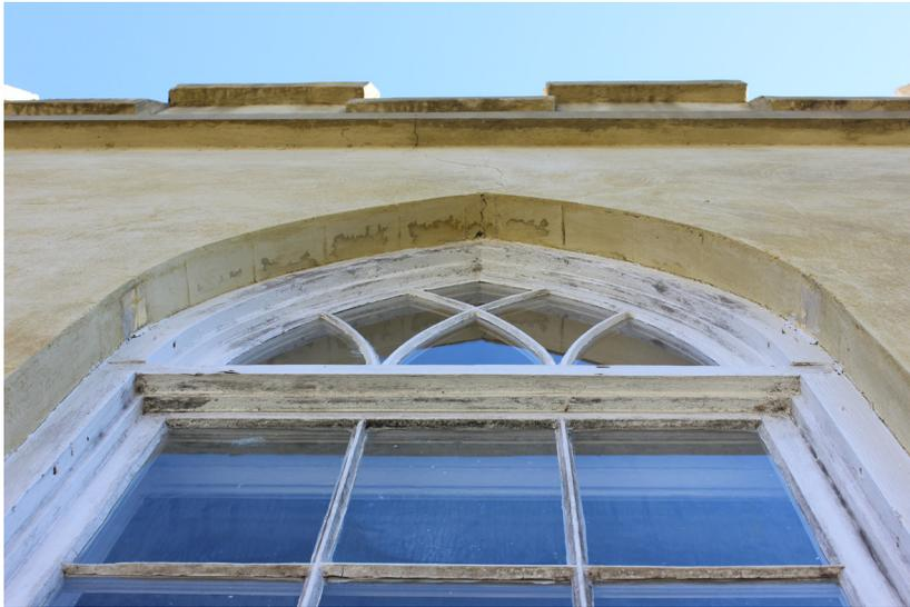
**Figure 146:** Biogrowth is present on all wooden elements.
