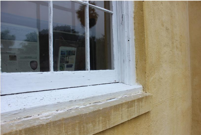
**Figure 44:** Several dutchman are present within the casing. The casing is soft at the lower portions of the window.
