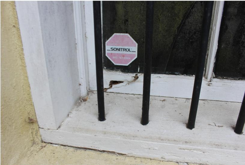
**Figure 84:** The window is heavily deteriorated at the bottom. The pane of glass is broken at the location.
