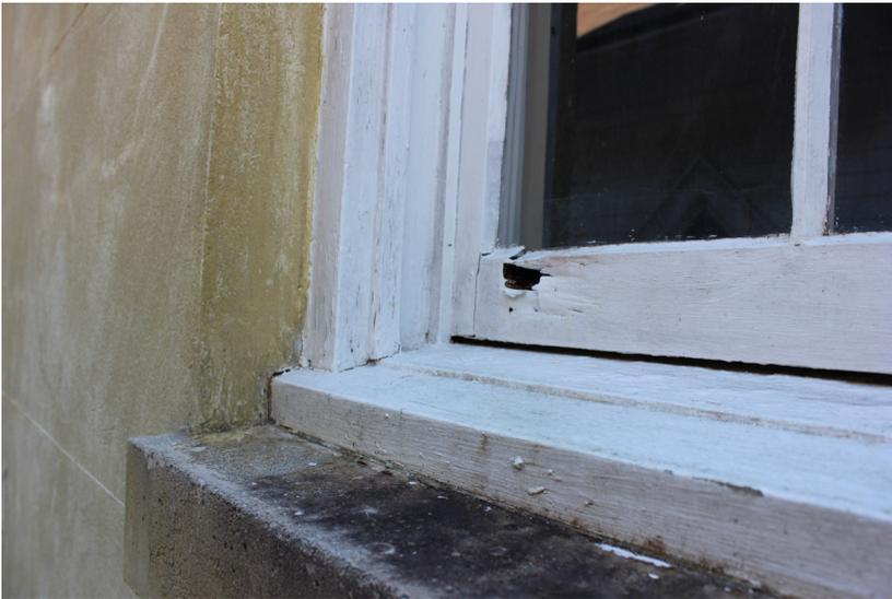
**Figure 128:** The bottom rail of the lower sash is deteriorated.
