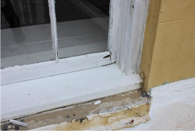
**Figure 15:** The lower sash is deteriorated along the bottom rail.
