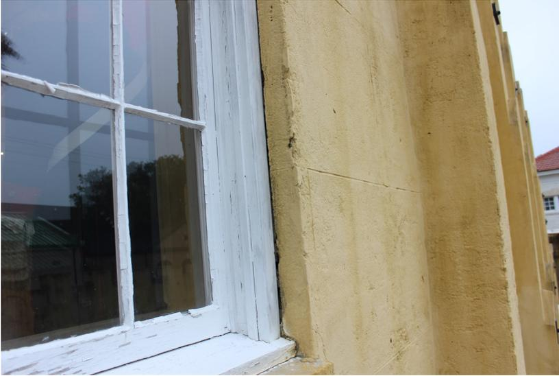
**Figure 27:** There is a small gap between the casing and the exterior stucco.
