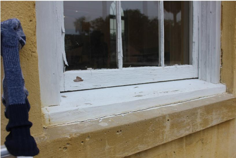
**Figure 40:** The lower sash is weathered but appears sound.
