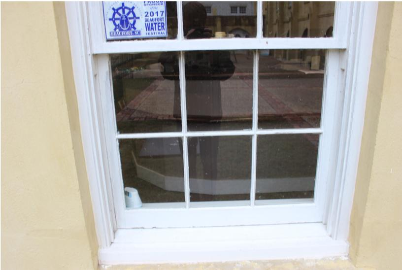
**Figure 60:** The bottom of the jamb and casing where it intersects the masonry sill is not caulked.
