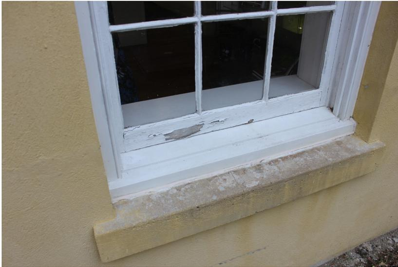
**Figure 63:** The bottom rail of the lower sash is heavily weathered.
