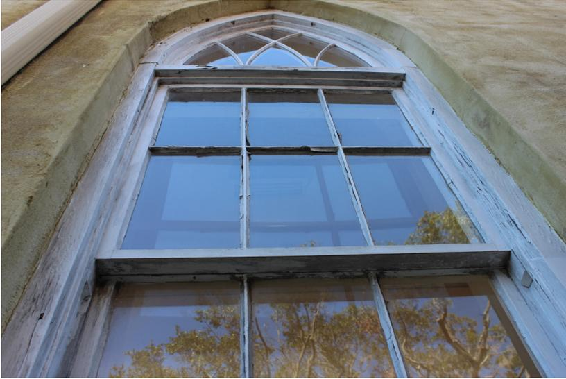
**Figure 103:** The casing on the left and right hand sides of the window are deteriorated.
