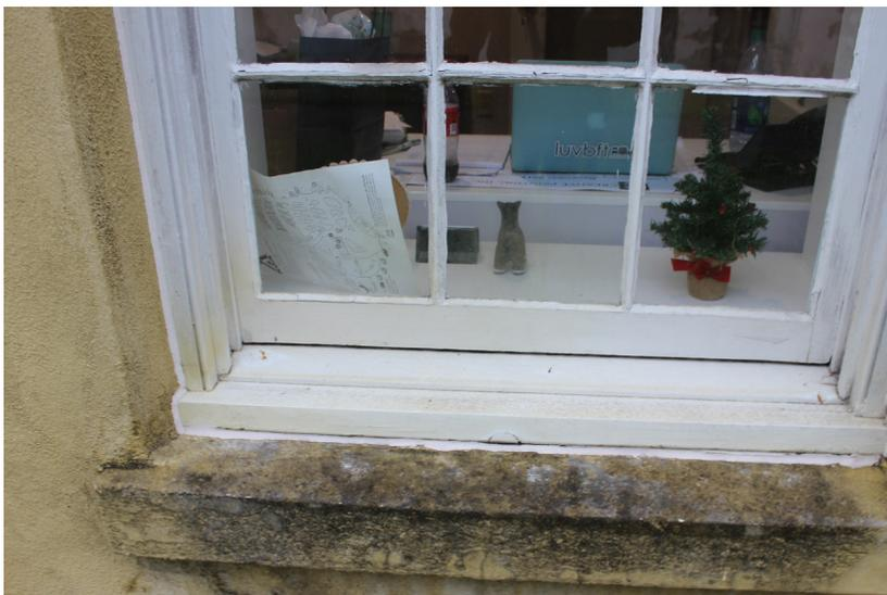
**Figure 160:** Detail of interior conditions and sill. A knot is present within the sill.
