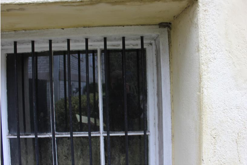
**Figure 83:** The head of the window is in fair condition.
