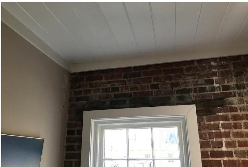
**Figure 57:** Detail of interior conditions. A leak is present within the masonry above this window.
