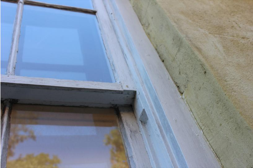
**Figure 115:** There is moderate separation of the joints within this window.
