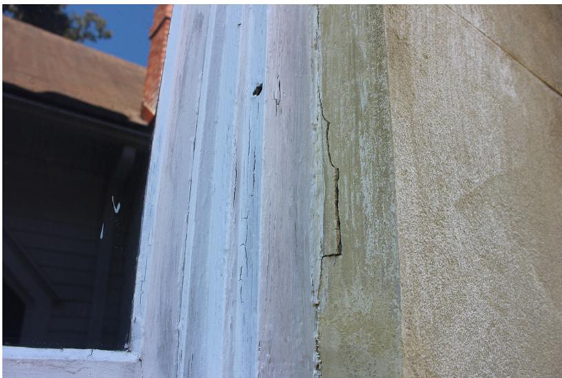
**Figure 129:** Detail of hole within the casing to secure plywood used for hurricane protection.
