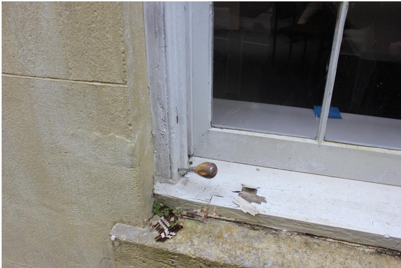
**Figure 5:** Detail of typical deterioration.
