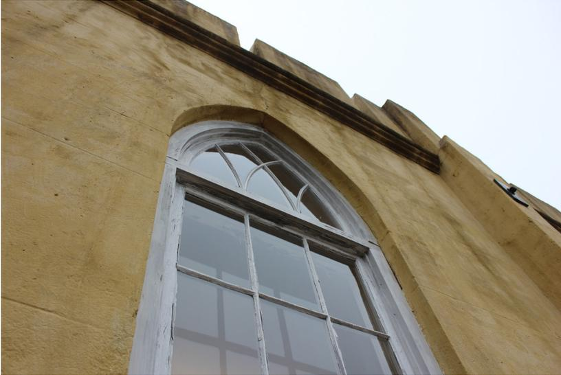
**Figure 39:** The transom casing is slightly proud of the lower window casing.
