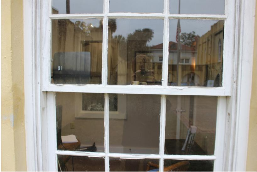
**Figure 55:** Glazing putty and paint failure are present throughout the window.
