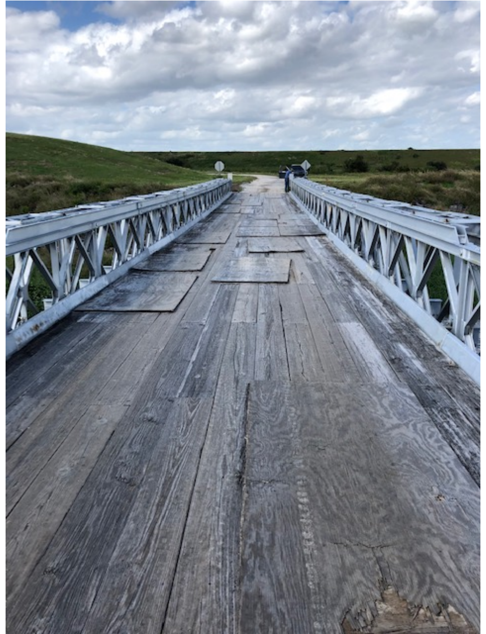
Existing Bridge Decking (South of S-157)
