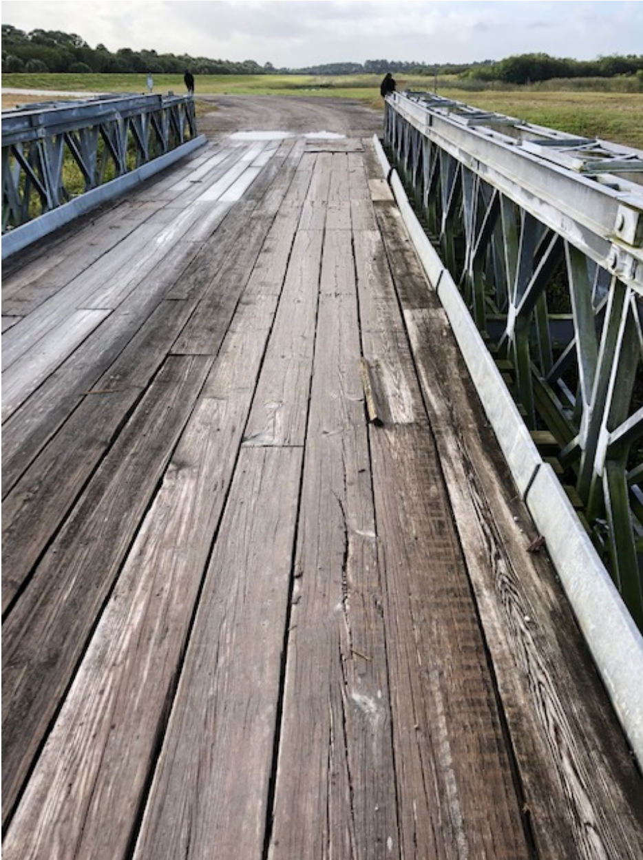
Existing Bridge Decking (North of Malabar)
