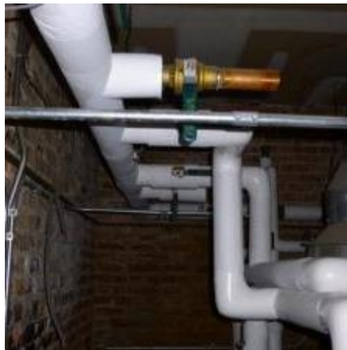
Insulate 100% of hot water pipe
