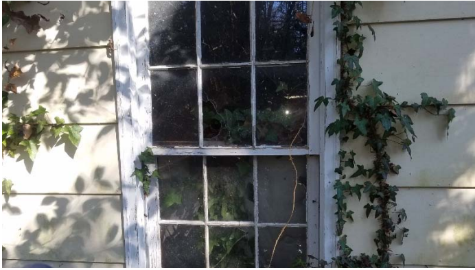
Photo 13 – Window glaze on detached shed.
