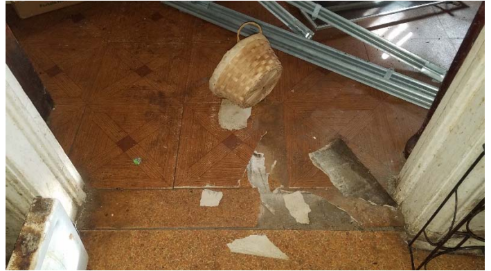
Photo 8 – Dining room wood pattern self-stick tile over orange roll vinyl flooring with felt.
