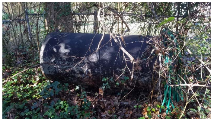
Photo 6 – 300 gallon fuel oil tank behind detached shed.
