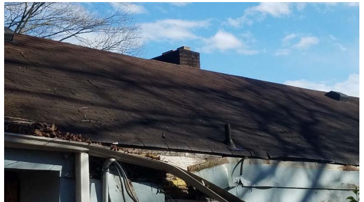
Photo 4 – Shingled roof and assumed asbestos chimney tar.
