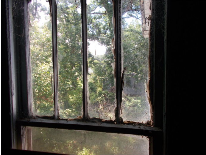
Photo 7 - Window glazing on the exterior windows.
