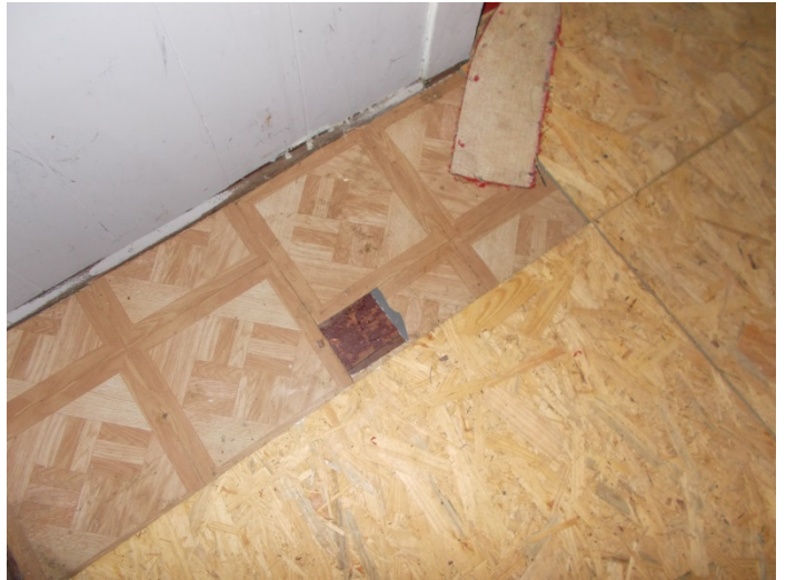
Photo 2 – Two layers of self-stick tile under wood in the kitchen.
