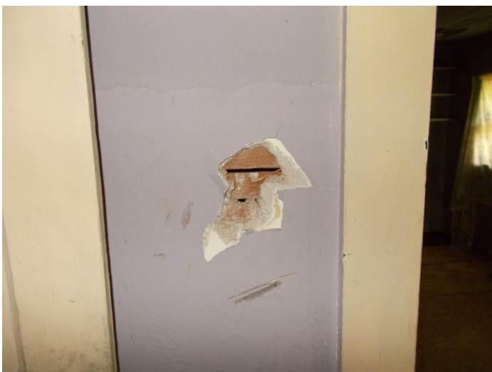
Photo 5 – Plaster with skim coat walls in the left room.
