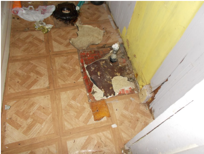
Photo 3 – Three layers of self-stick tile, under linoleum and wood in the bathroom.
