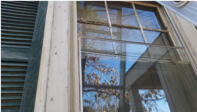
Photo 3 – Exterior window glazing.
