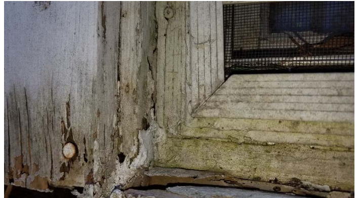
Photo 4 – Exterior window caulk.
