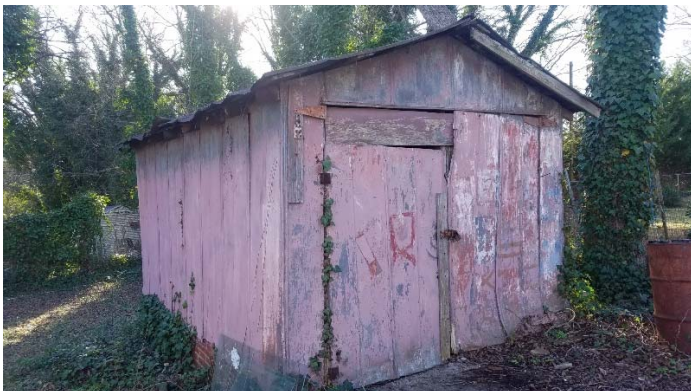
Photo 5 – Detached shed in back yard.
