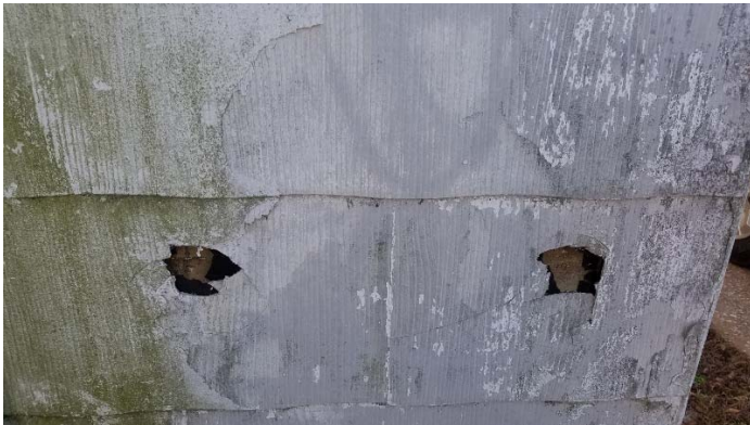
Photo 3 – Transite exterior siding with felt.
