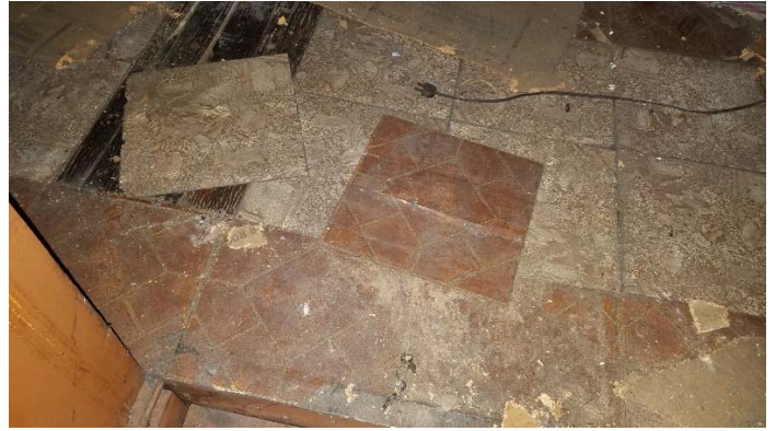
Photo 14 – Self-stick tile flooring in partially finished attic. Same as two layers in kitchen samples.
