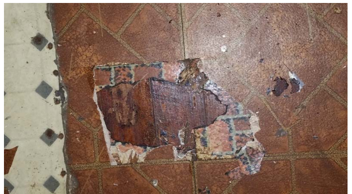
Photo 12 – Multiple layers of kitchen flooring.
