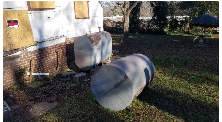
Photo 4 – Two fuel oil tanks behind the house.
