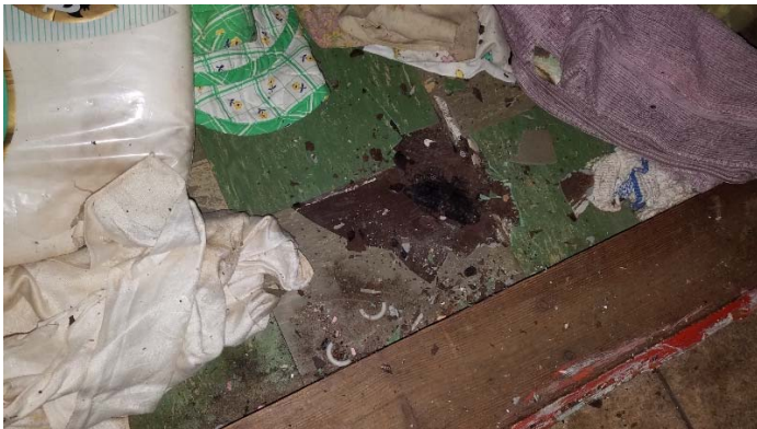
Photo 9 – Bathroom closet flooring.
