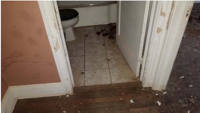
Photo 9 – Bathroom tan roll vinyl flooring with mastic under tile and wood sub-floor.
