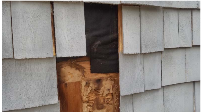
Photo 10 – Black felt under exterior cedar shake siding.
