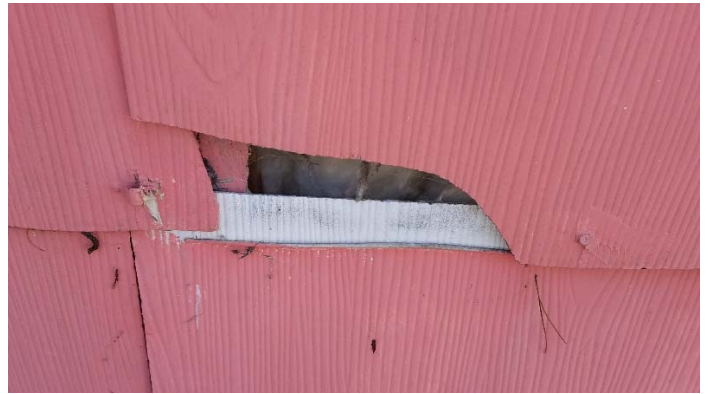
Photo 2 – Transite exterior siding without felt.
