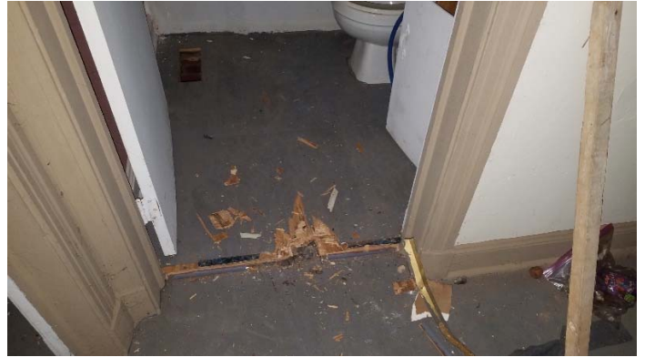
Photo 8 – Bathroom tile under wood sub-floor.
