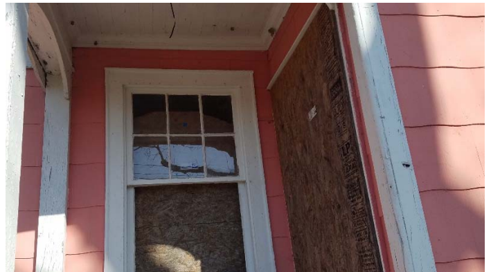
Photo 4 – Exterior window glaze and caulk.
