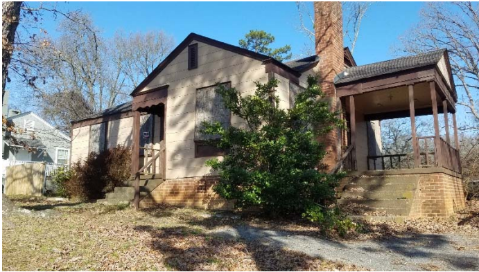
Photo 1 – 690 Saxon Avenue in Spartanburg, South Carolina.
