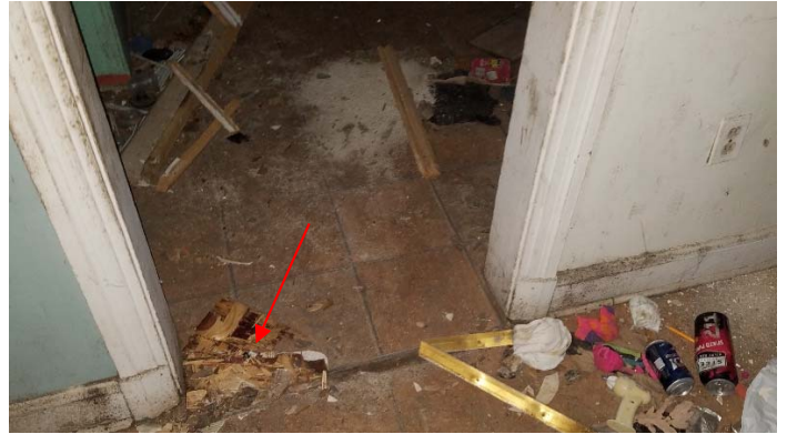
Photo 8 – Kitchen flooring layers under wood sub-flooring.
