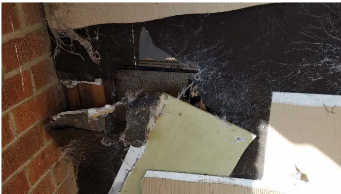
Photo 5 – Transite siding over black felt over drywall with attached black paper.
