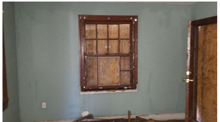
Photo 6 – Exterior window glaze and caulk.
