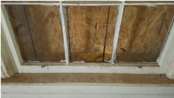
Photo 3 – Exterior window glazing.
