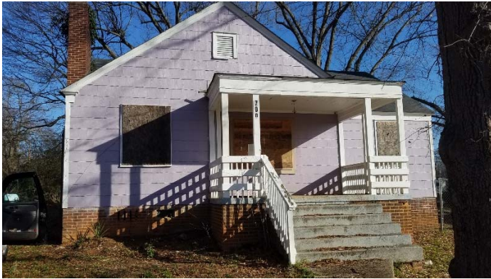
Photo 1 – 700 Saxon Avenue in Spartanburg, South Carolina.
