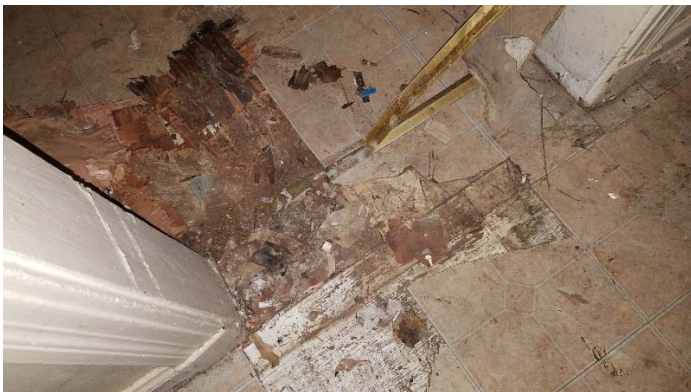
Photo 5 – Multiple flooring layers kitchen and dining room.
