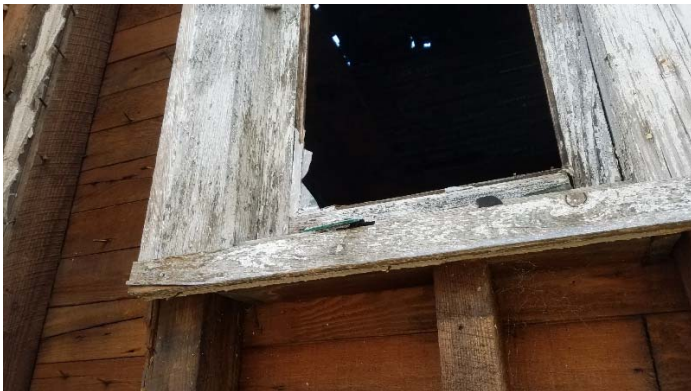
Photo 3 – Exterior window glazing.
