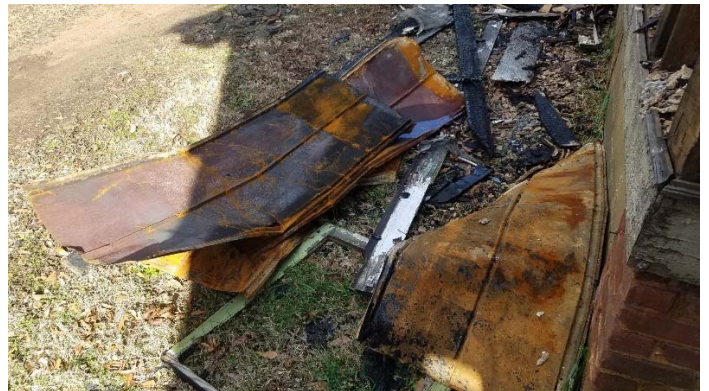
Photo 4 – Tar on metal roofing.
