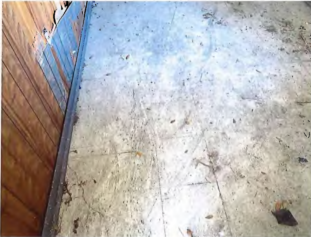
Asbestos Containing 12" X 12" Floor Tile (Beige) Two Layers, Throughout Radio House
