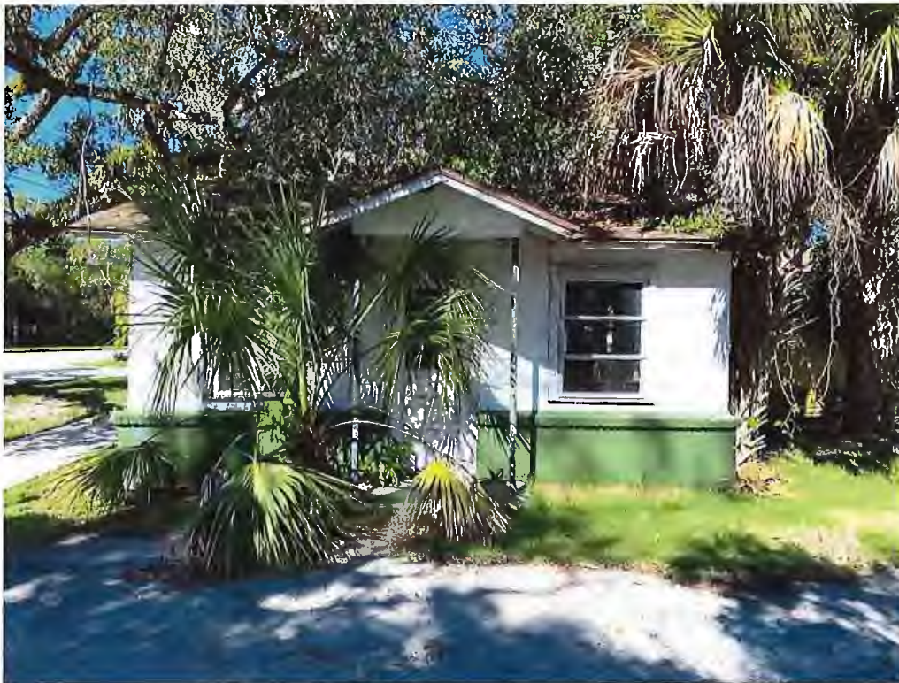
Looking West at Radio House
