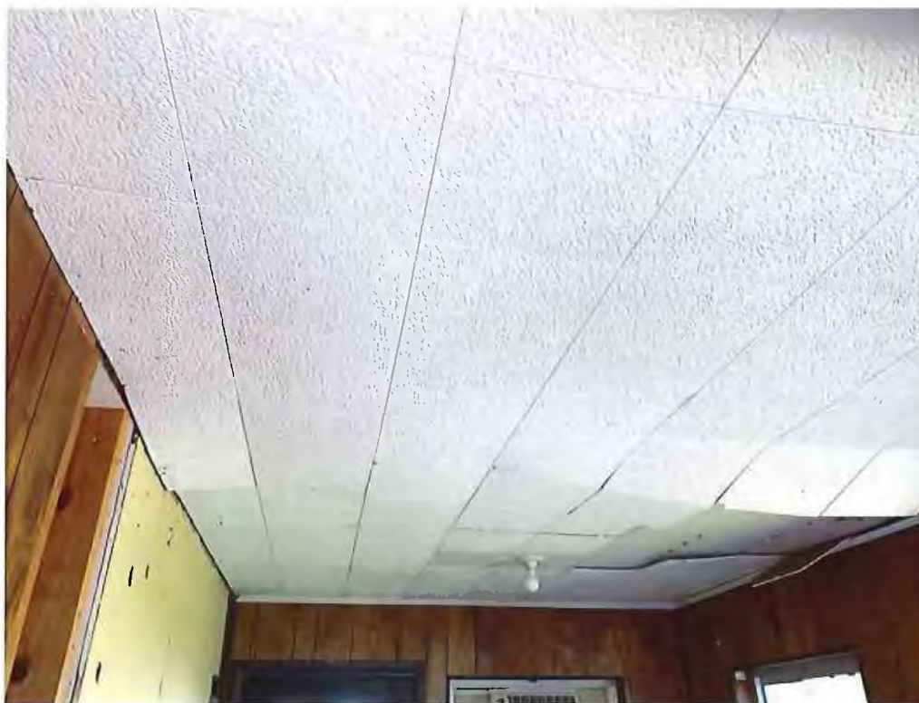
1' X 1' Z Spline Ceiling Tile, Throughout Radio House
