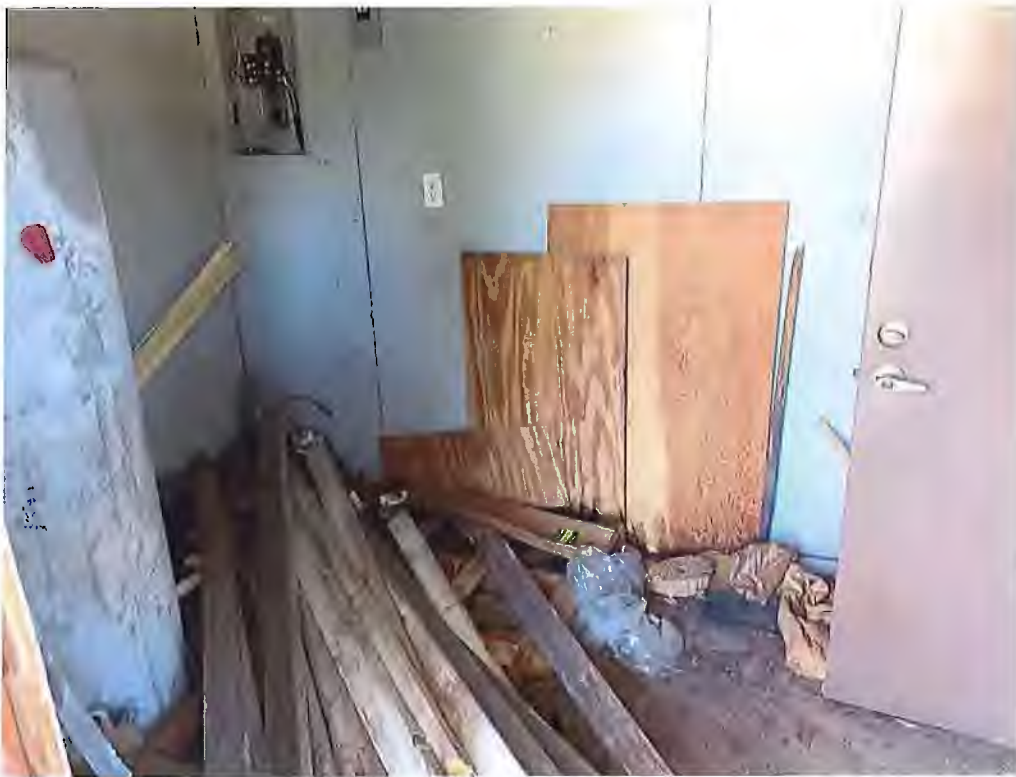
Interior View, Shed
