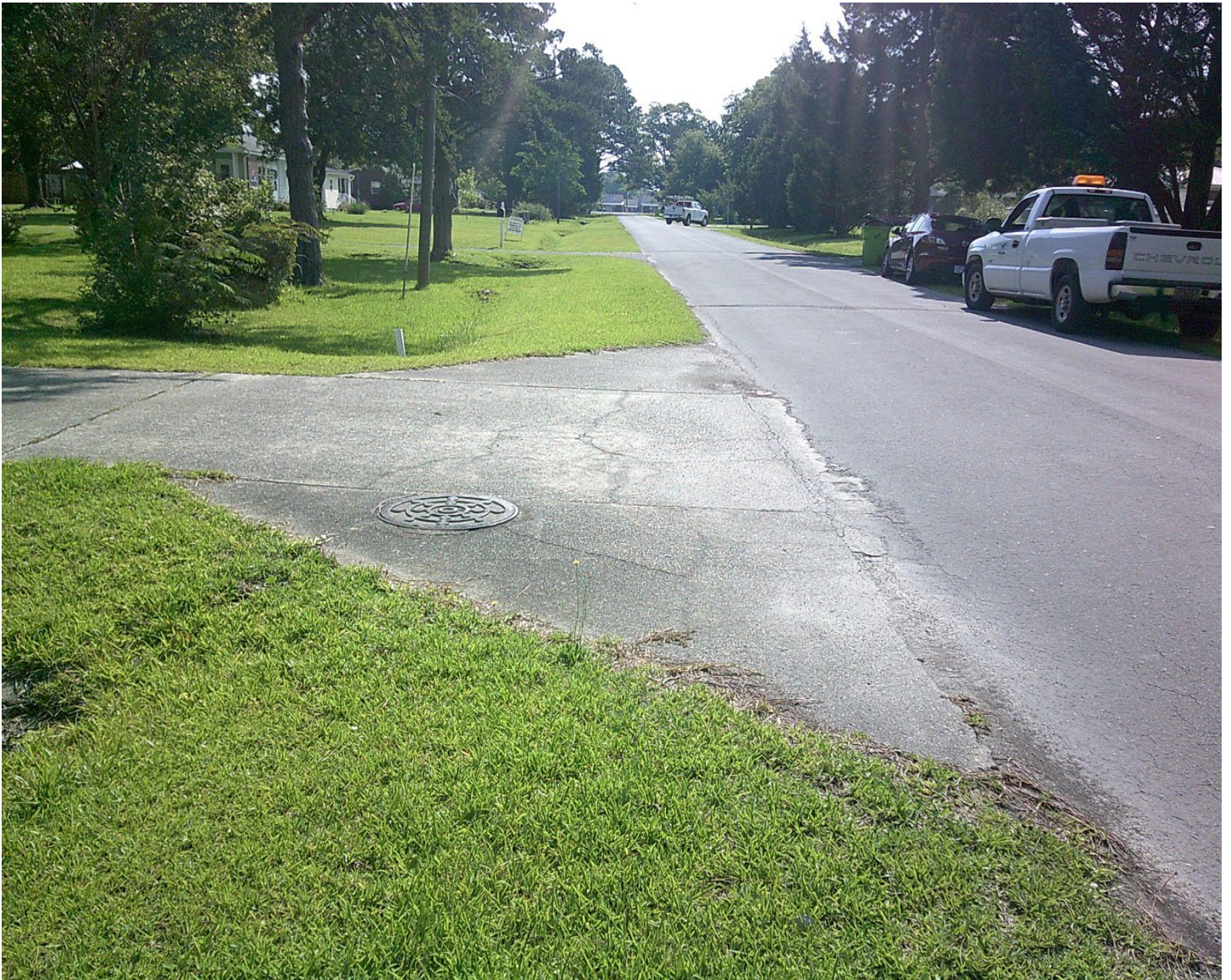
Figure 2. East End Work area.
