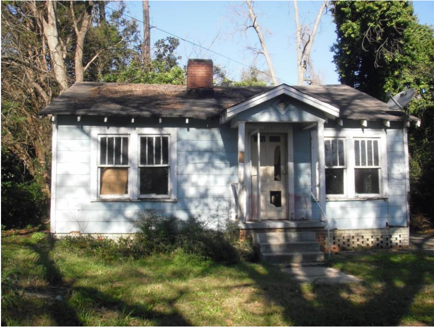
205 Prince St. – siding tested positive for asbestos
