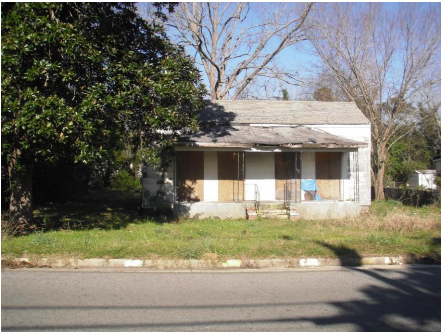
303 E. Mary St. – siding tested positive for asbestos
