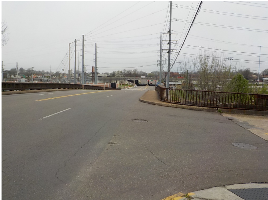
APPROACH BACK ON LOG - RAIL REPAIRED 2 LEFT
