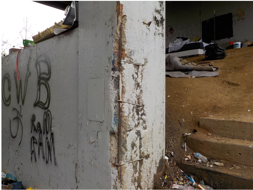
COLUMN A BENT 1 EXP REBAR TYPICAL
