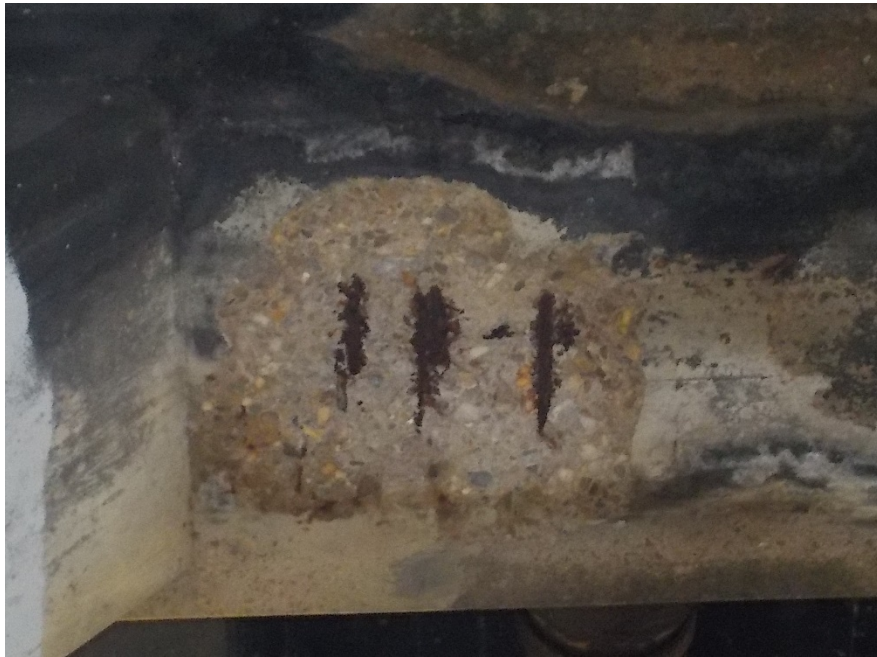
BENT CAP 1 EXP REBAR TYPICAL
