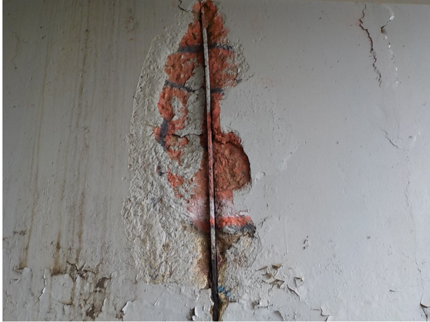
ABUTMENT 1 EXP REBAR TYPICAL
