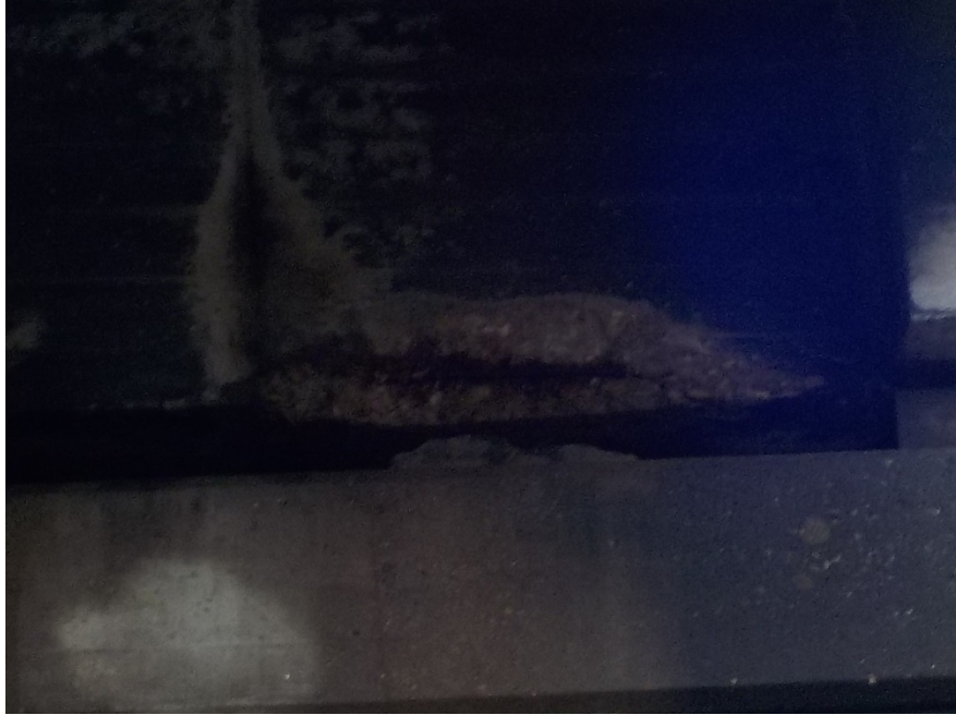
DIAPHRAM BENT 2 EXP REBAR TYPICAL
