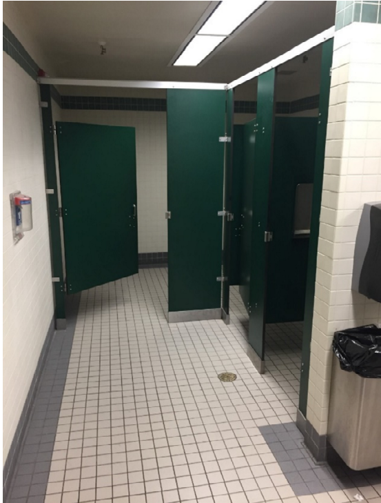
Existing Women's Restroom Area
