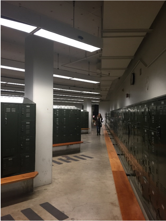
Existing Men's Locker Area
