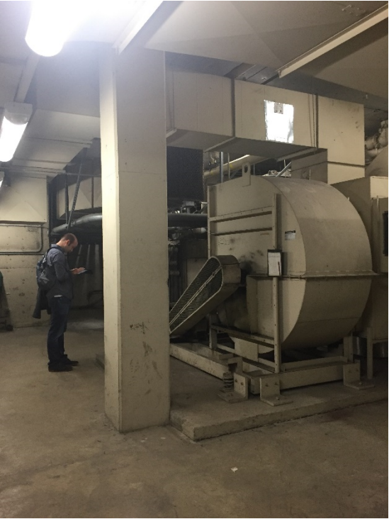
Existing Mechanical Room
