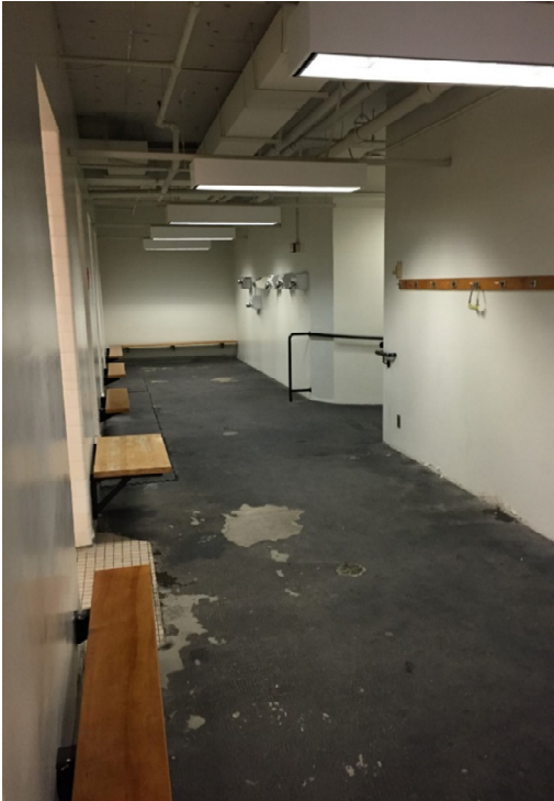
Existing Women's Shower Area
