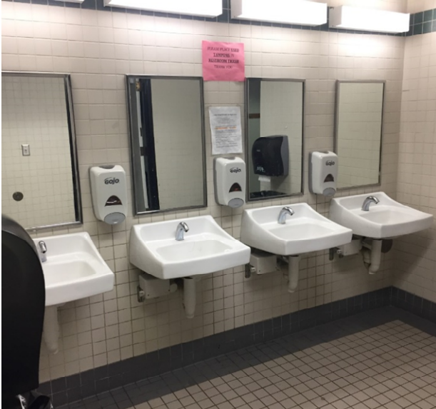
Existing Women's Sink Area
