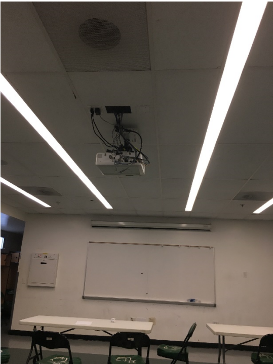
TEAM ROOM: LOCKER AREA
