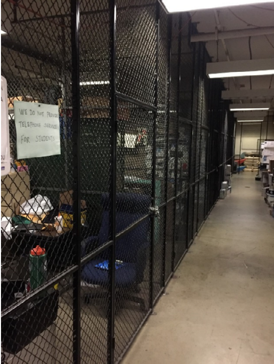
Existing Caged Storage Room
