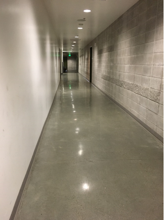
HALLWAY (STORAGE AREA)
