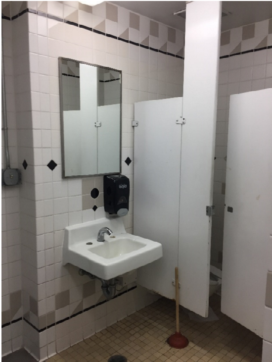
Existing Faculty/Staff Restroom Area
