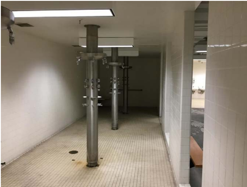
Photograph 6: View depicting the shower room area.
