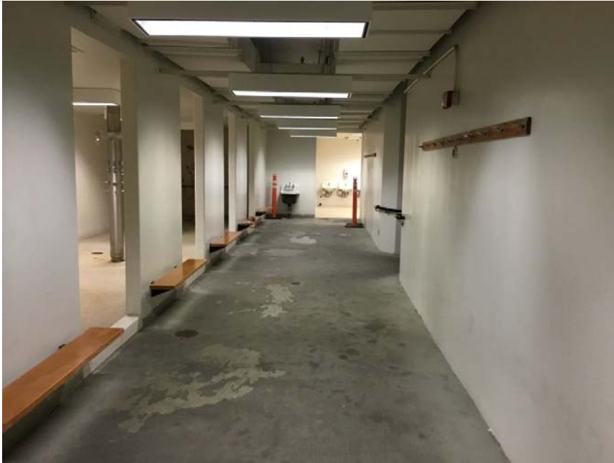
Photograph 5: View depicting the shower room vestibule area.
