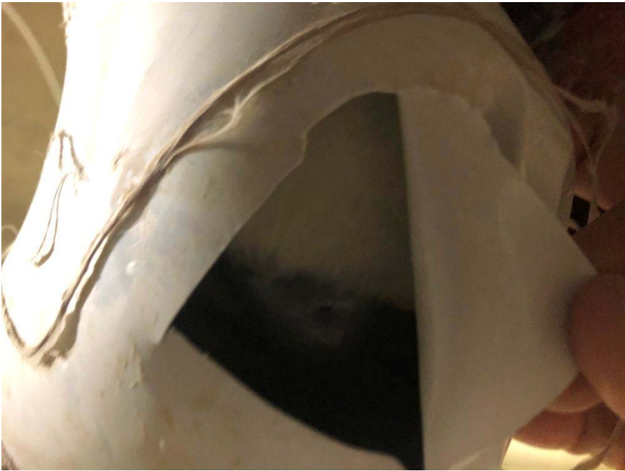
Photograph 12: View of non-asbestos insulation pipe runs.
